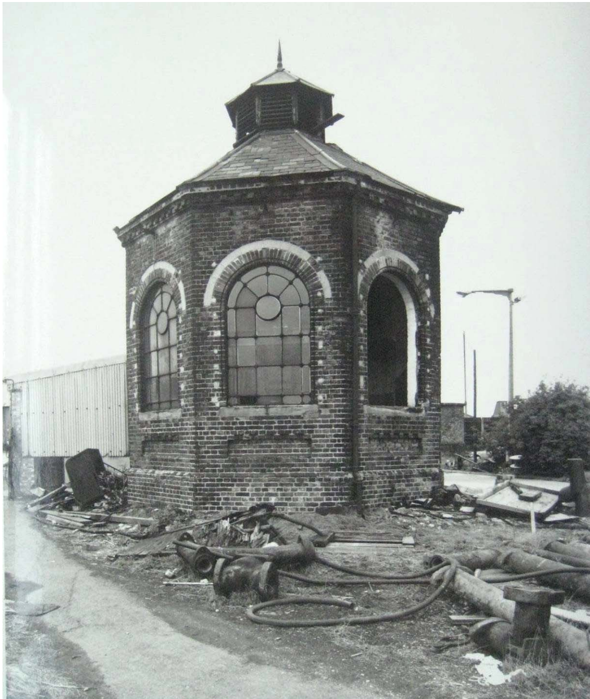
Fig 10 The eastern elevation looking west, taken 1977. (LMA SC/PHL/02-SSo4 0921-30)
