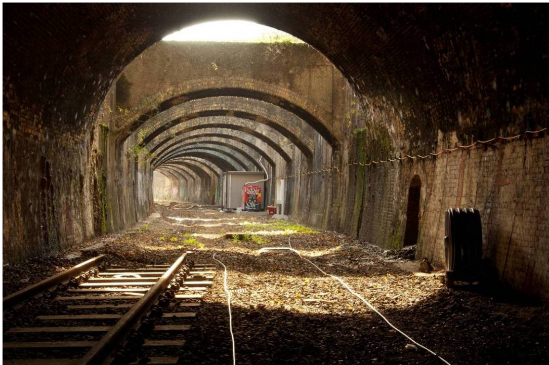
Photo 41 The view south through the southern portal towards the buttresses of the southern cutting.
