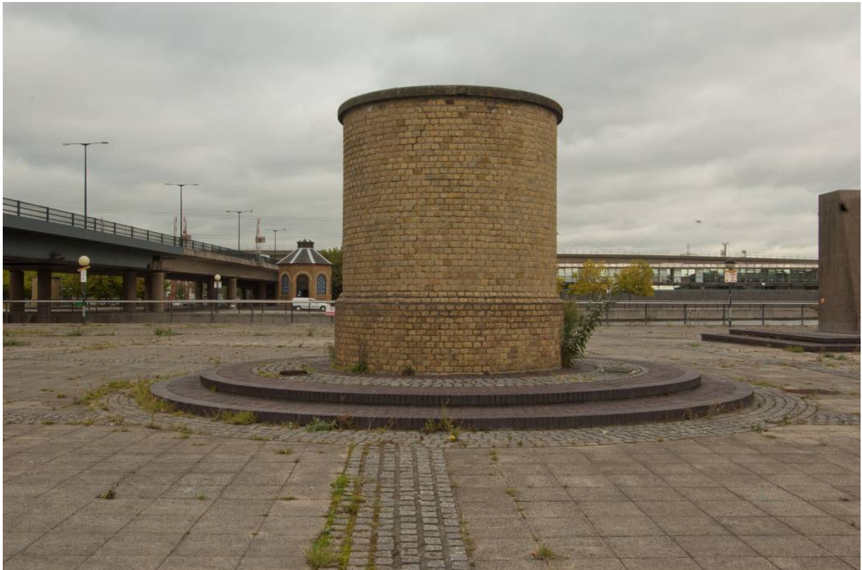
Photo 21. The southern air vent structure with the pumphouse in the background, the northern air vent is just visible behind the Connaught Bridge in the far left of the photo.
