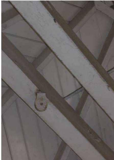
Photo 12 left and Photo 13 right. The two pulleys within the pumphouse. The left pulley was mounted on the northernmost cross timber, the right in the south east corner.
