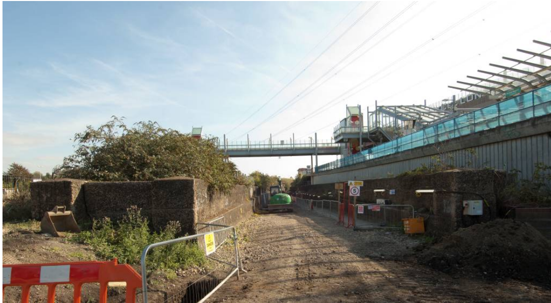
Photo 22. The northern entrance to the cutting of the Connaught Tunnel looking east.
