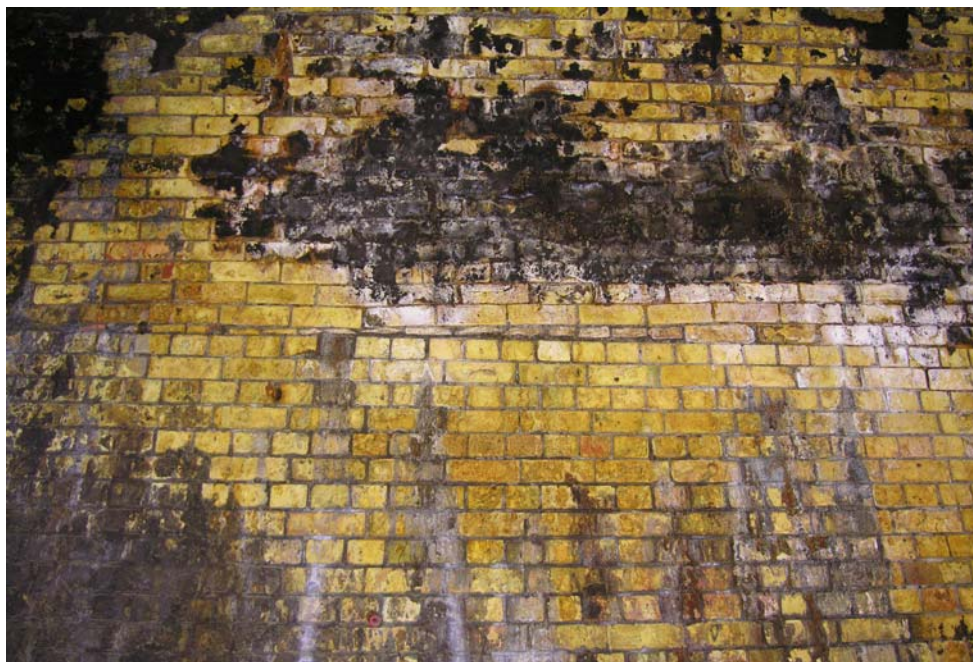
Photo 29. The change in brick bonding from English to stretcher in the northern single tunnel section and the gradual insertion of an extra course of stretcher bricks from left to right.
