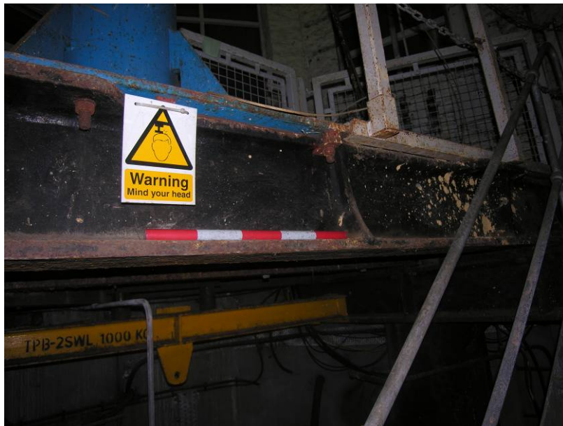
Photo 16. The possible 19th century wrought iron joist across the centre of the shaft opening, used to support the modern hoist.
