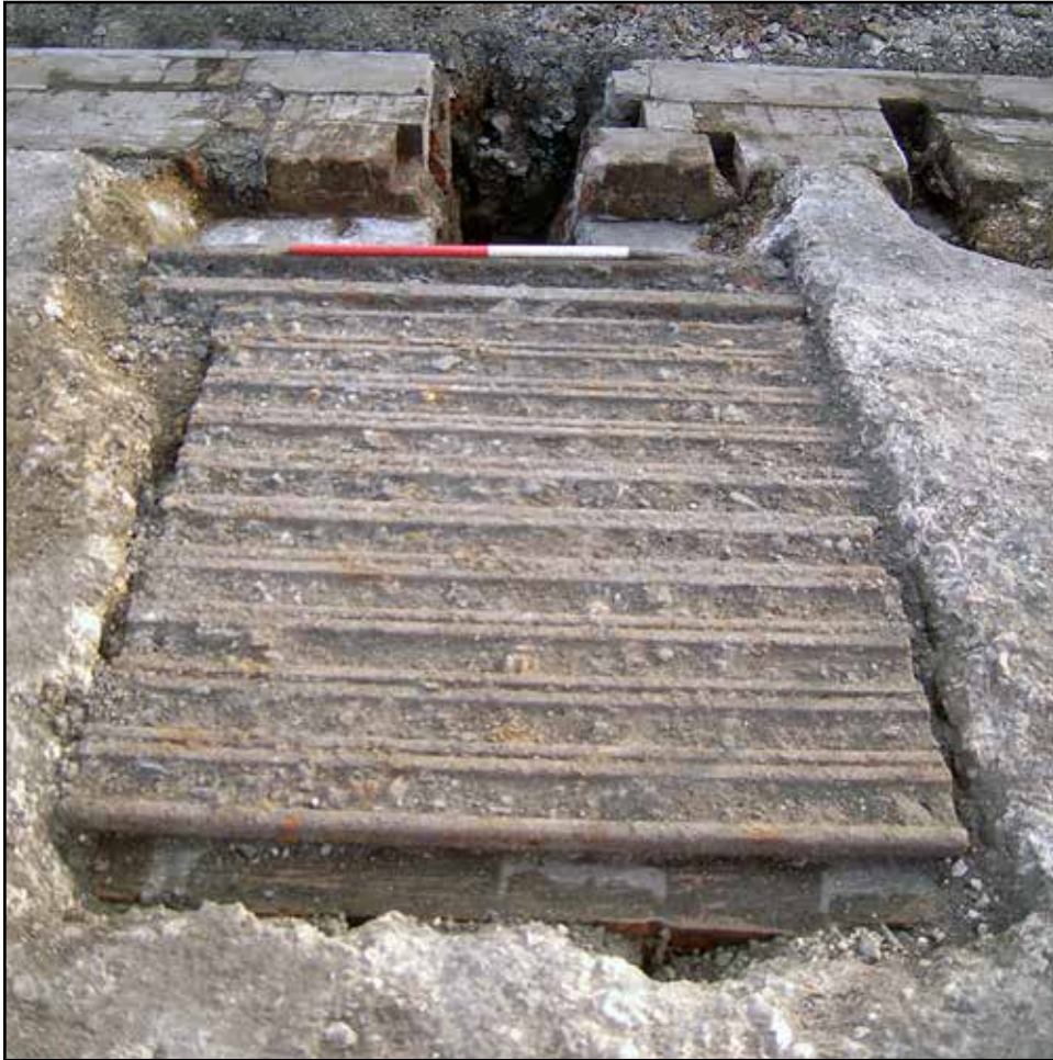
Plate 53: Access chamber [8448] into Marcon Sewer covered by sections of bridge rail [8447]
