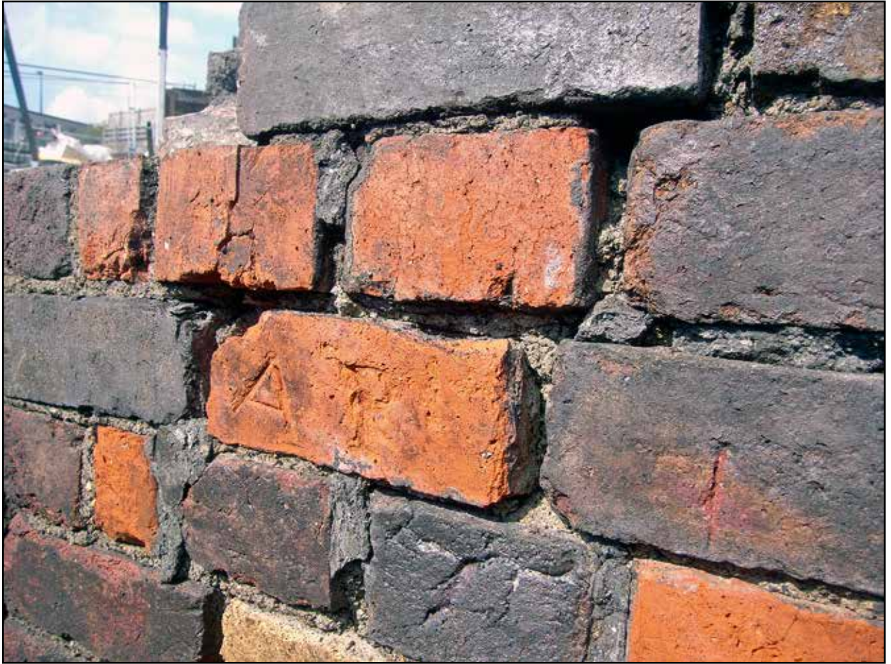
Plate 9: Graffiti on northern wall of engine house [8528]
