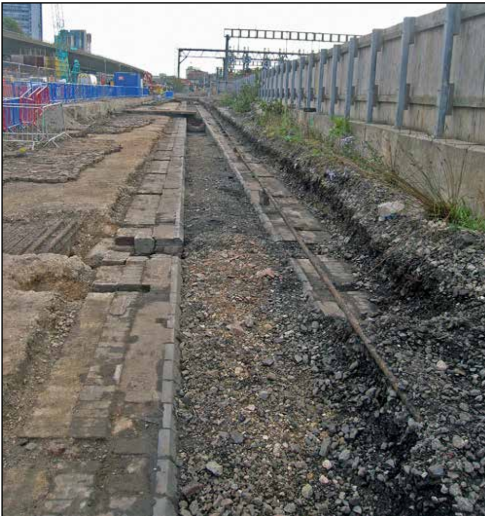
Plate 50: Partly excavated inspection pit
