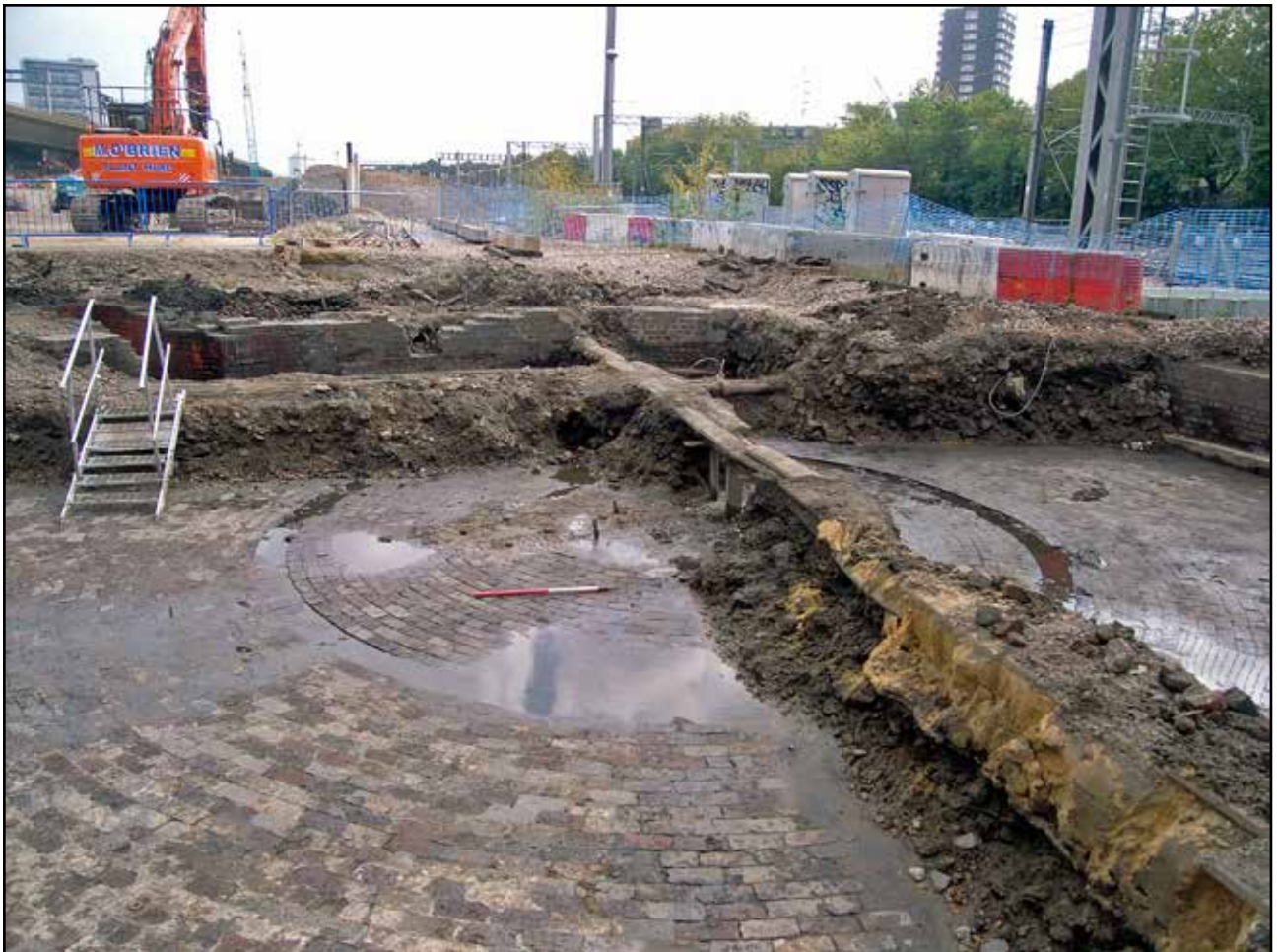
Plate 2: Turntable pit floor [8524] and drainage gully [8525]
