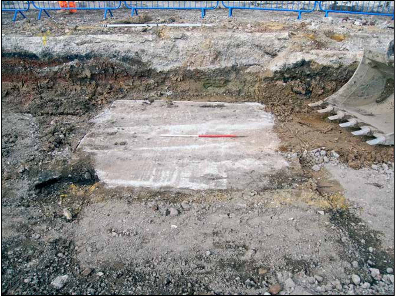
Plate 59: Concrete foundations of Alfred Road Warehouse
