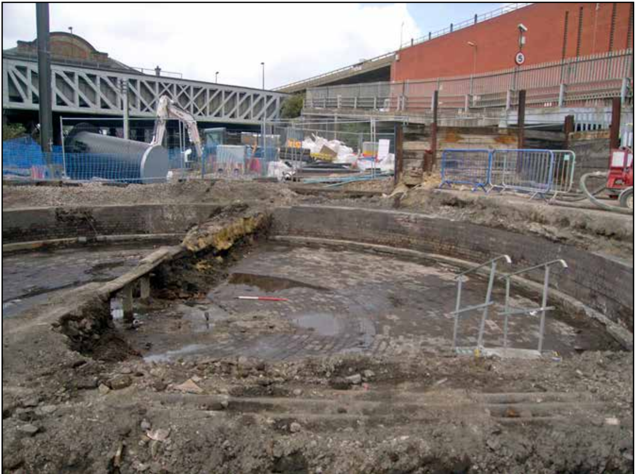
Plate 4: Overall from east showing floors [8524] and [8526]
