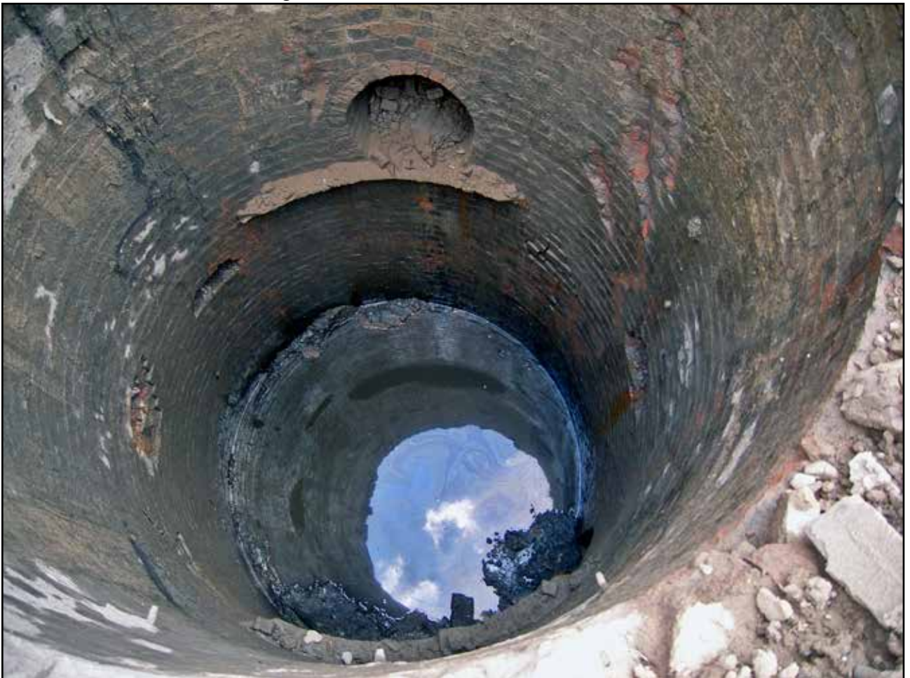
Plate 44: Base of [8227] showing entrance to [8251] and [8250]
