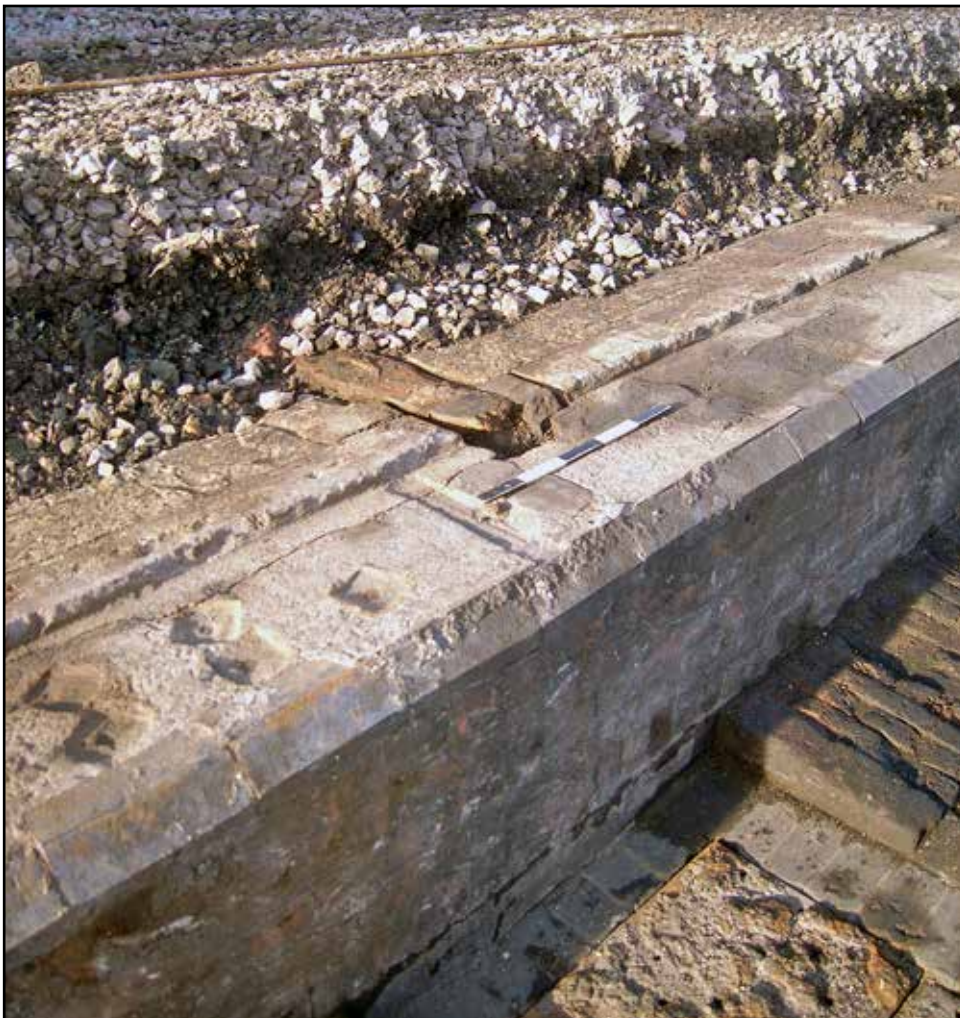
Plate 52: Detail of standard gauge pit wall showing timber sleeper and marks of screw jacks
