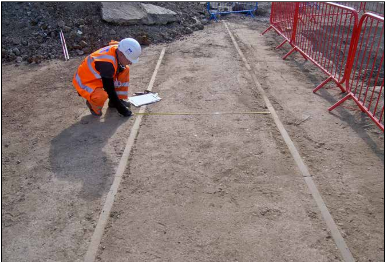
Plate 46: Remains of Portobello Junction
