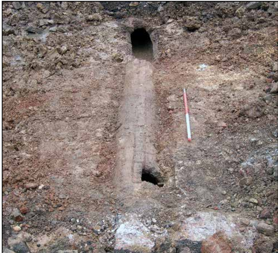
Plate 32: Conduit [8153] beneath 1852 Workshop's "Store Rooms"
