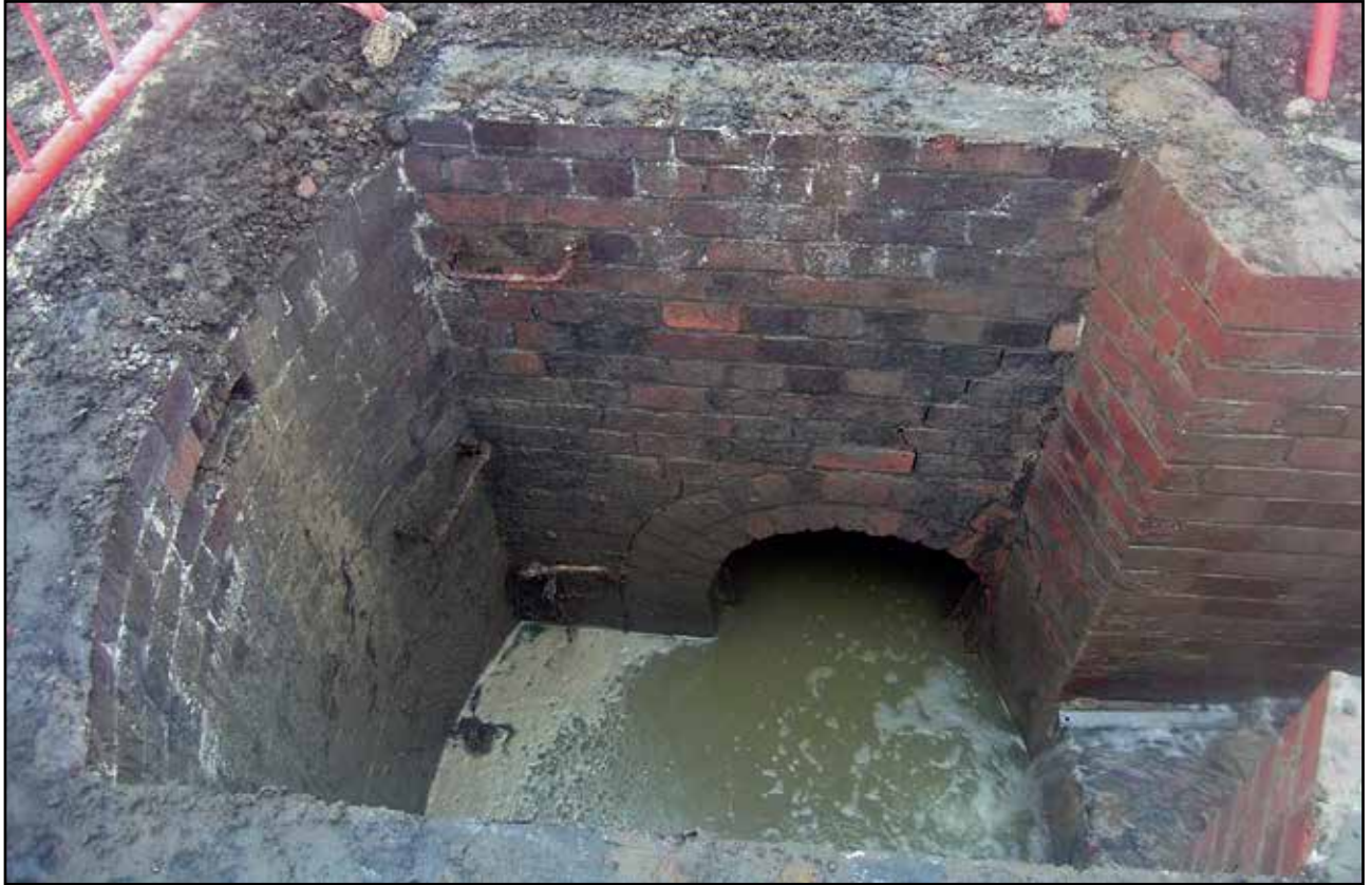
Plate 55: Access chamber [8897] and entrance to Marcon Sewer [8898]
