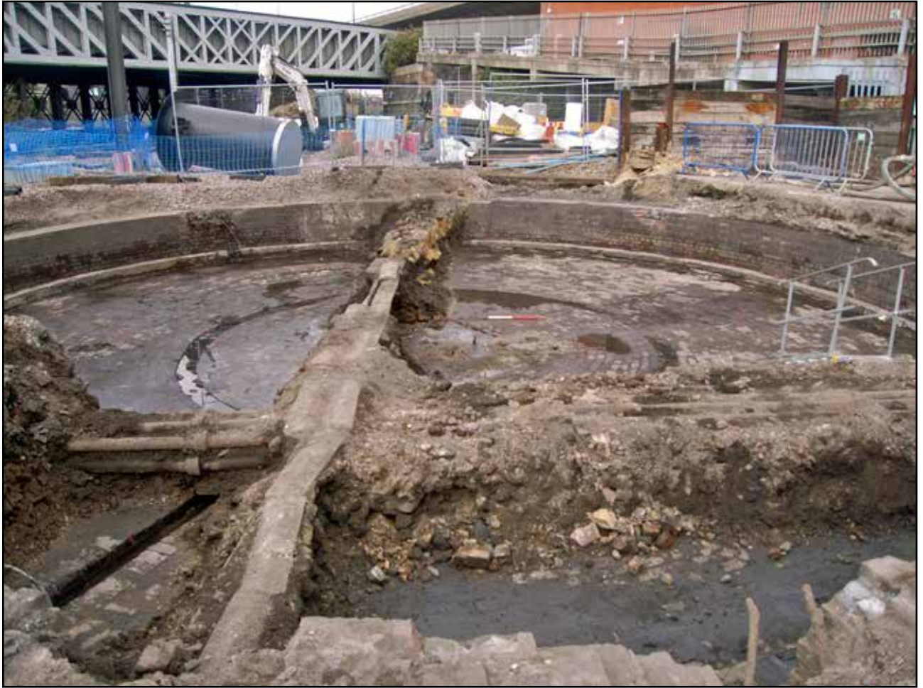
Plate 1: Overall view of western Turntable from southeast
