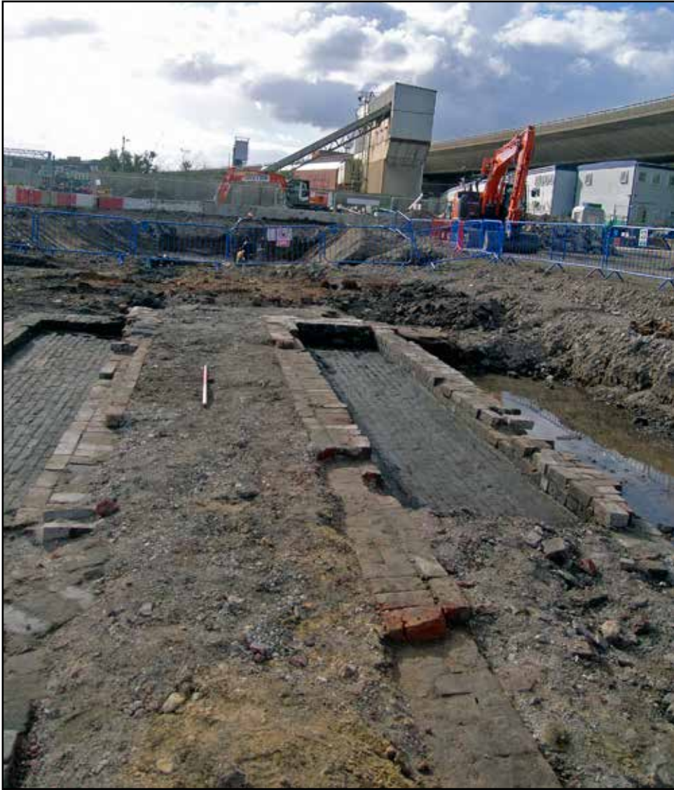
Plate 35: Inspection pits 8915 and 8916 in western extension of Workshop
