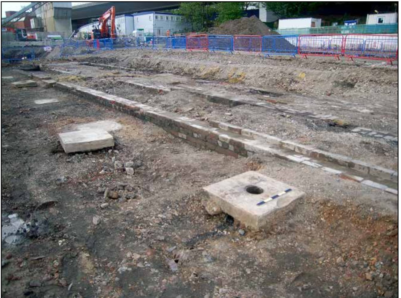
Plate 38: Stone plinths for roof supports along southern edge of western extension of Workshop
