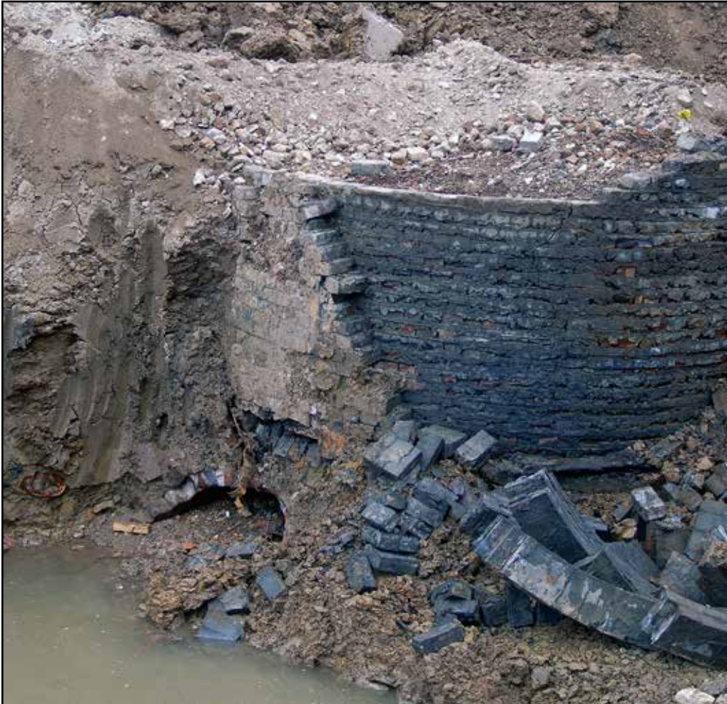
Plate 43: Shaft 8206 showing double skinned wall
