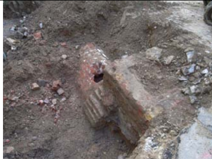
4769 and manhole 4770 from south west
