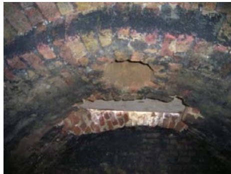
Aperture in 4036 roof, looking east
