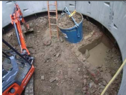
Grout Shaft 4, exposed manhole
