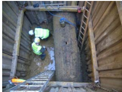
Sewer in situ, looking east
