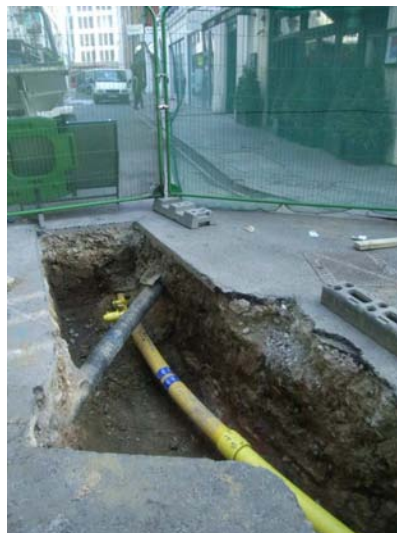
Installing gas services Tenterden Street, looking north to Dering Street
