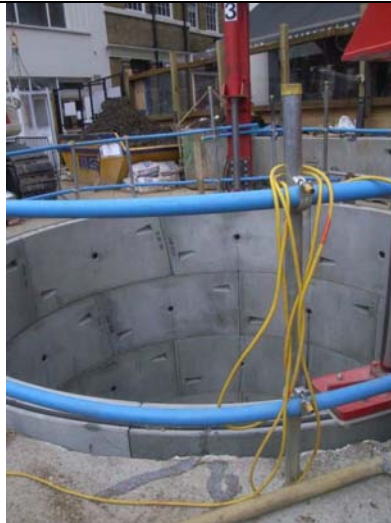
Grout Shaft 3, location view, looking west
