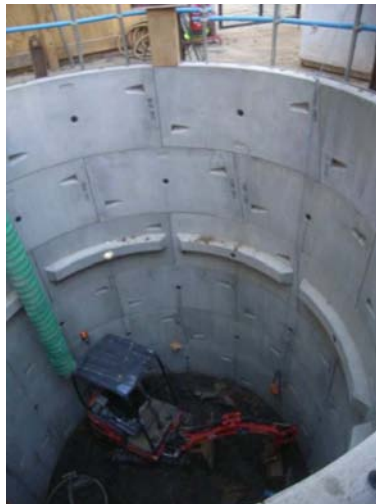
Grout Shaft4, natural clay at the base
