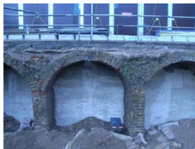
Arched vaults, 4625, visible beyond the western side of the XSC10 excavation, below Gilbert Street, looking south-west
