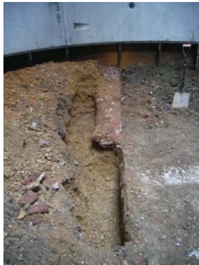
Grout Shaft 3, lower brick structure
