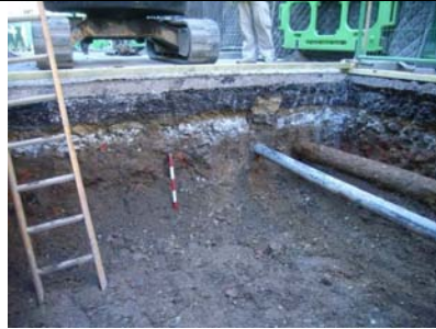
Sewer diversion, upper layers, looking west
