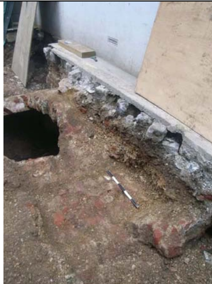
Adjacent brick vaults, looking NE
