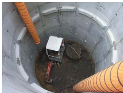
Grout Shaft 3, natural gravels and clay at base
