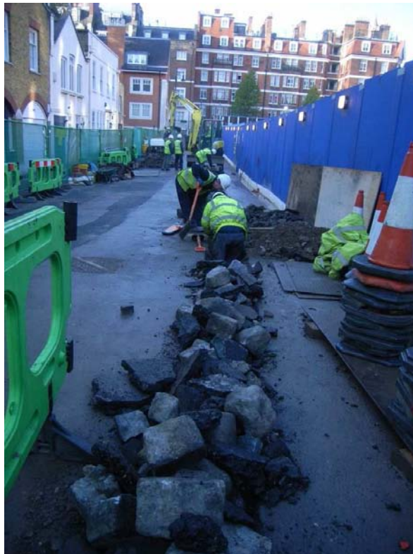
Plate 3: St. Anselm's Place, a third service diversion trench being dug, the earlier ones are to the left of the picture, looking west.
