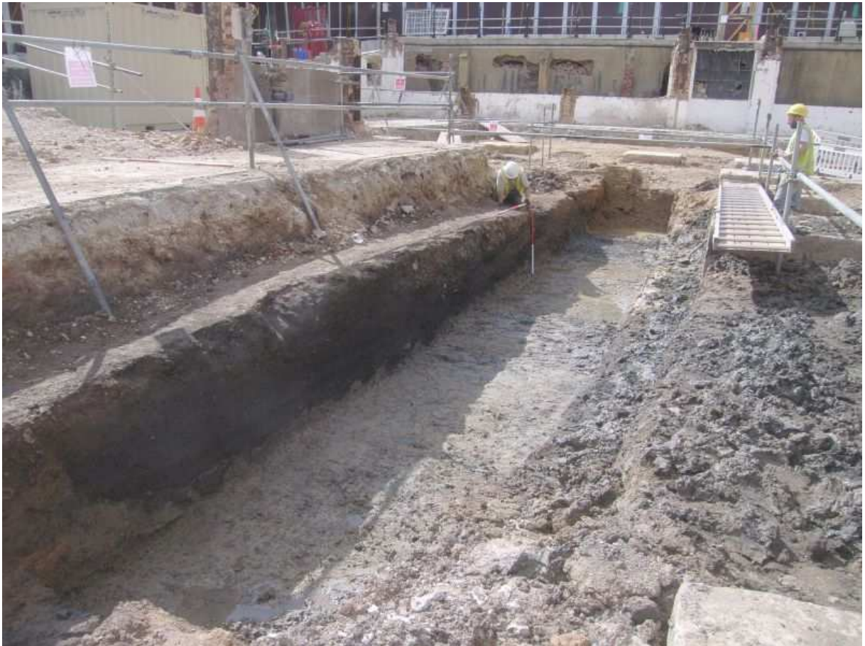
Plate 2: View of the section through the upper Tyburn river deposits, looking south-west
