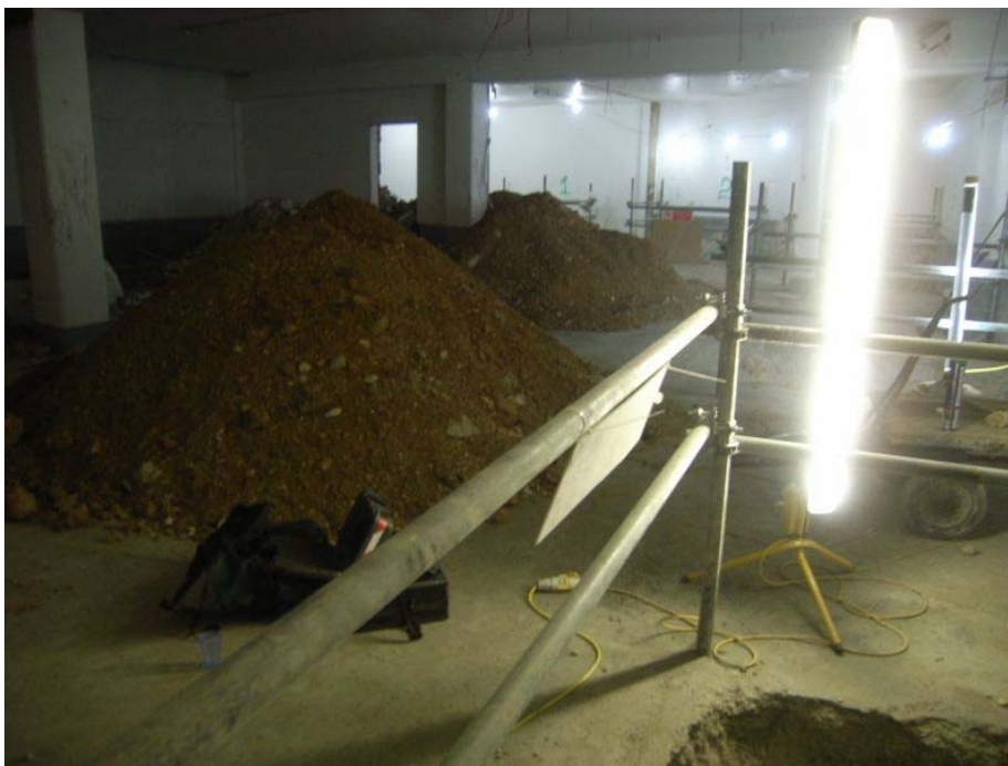
Plate 4: General view of test pit works in the basement of 18 Hanover Square, looking west
