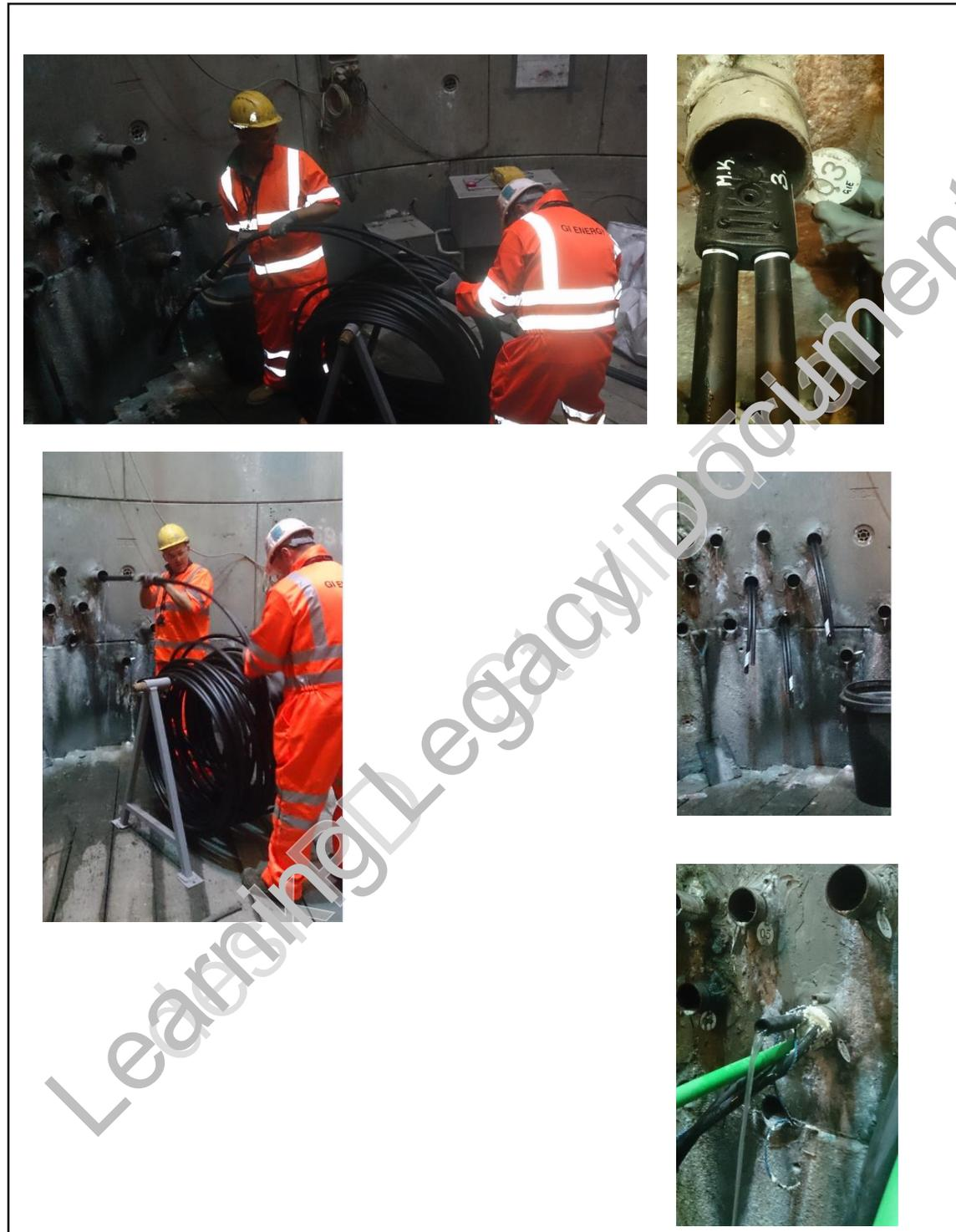
Figure 5: Installation of Loops into the TAMs
