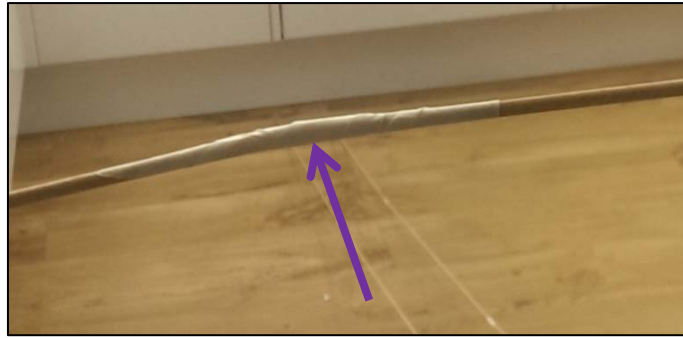
Figure B: The temptation will be to just tape where the joint is, but this won't work well. Apply tape liberally. The arrow shows where the joint is. The taped section here is about 10cm long
