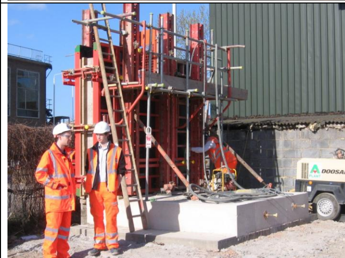
Photograph 66 Trial Panel Wall Pour formwork. Pre-pour inspection. 14th April 2014
