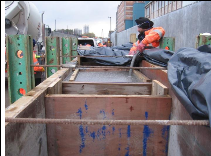
Photograph 34 Second Block Trial, discharge and placing 21st November 2013
