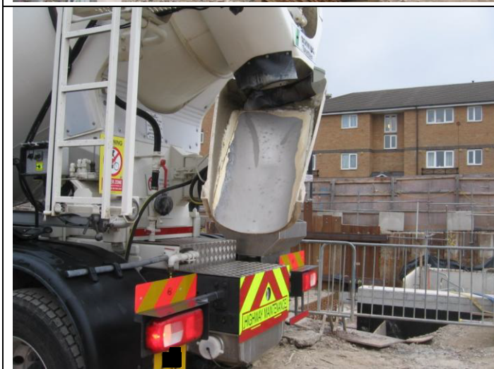
Photograph 59 Trial Panel Base Pour concreting. Second concrete delivery. 4th April 2014
