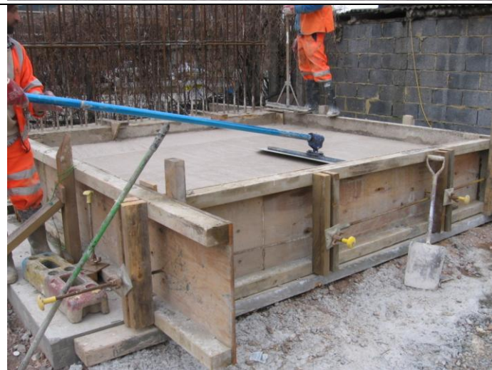
Photograph 63 Trial Panel Base Pour concreting. Surface finish 4th April 2014
