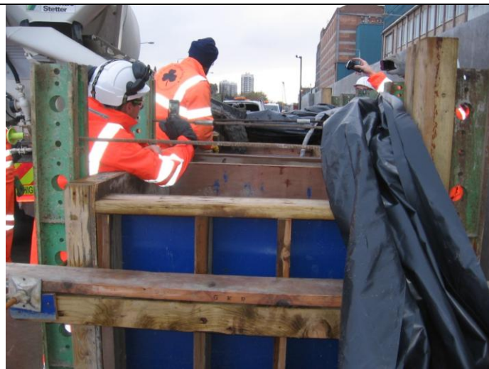
Photograph 32 Second Block Trial, discharge and placing 21st November 2013
