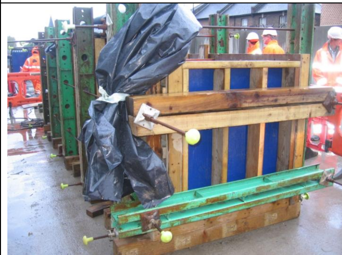
Photograph 05 Block Trial formwork. 21st November 2013
