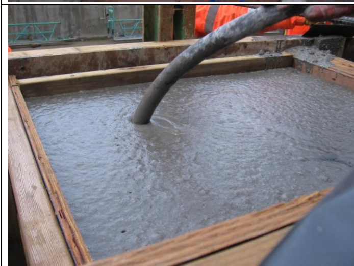
Photograph 35 Second Block Trial, discharge and placing 21st November 2013
