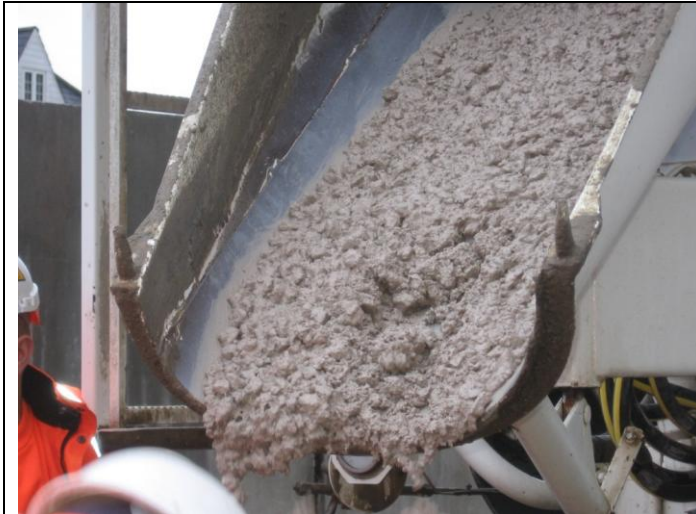
Photograph 16 First Block Trial, concrete on chute 21st November 2013
