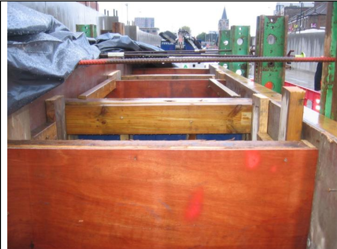
Photograph 04 Block Trial formwork 21st November 2013
