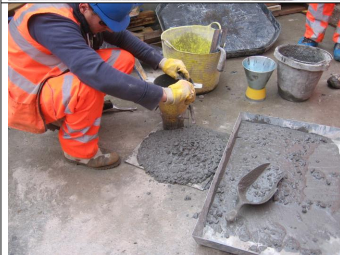
Photograph 30 Second Block Trial, slump prior to pouring 21st November 2013
