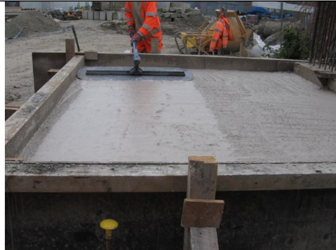
Photograph 61 Trial Panel Base Pour concreting. Surface finish 4th April 2014
