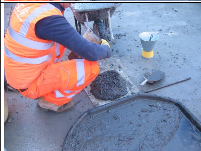
Photograph 41 Third Block Trial, slump prior to pouring 21st November 2013
