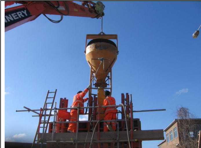
Photograph 67 Trial Panel Wall Pour concreting. 14th April 2014
