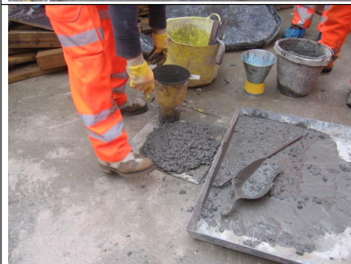
Photograph 29 Second Block Trial, slump prior to pouring 21st November 2013
