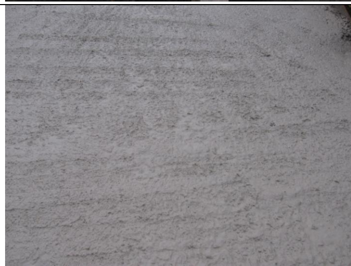
Photograph 62 Trial Panel Base Pour concreting. Surface finish 4th April 2014
