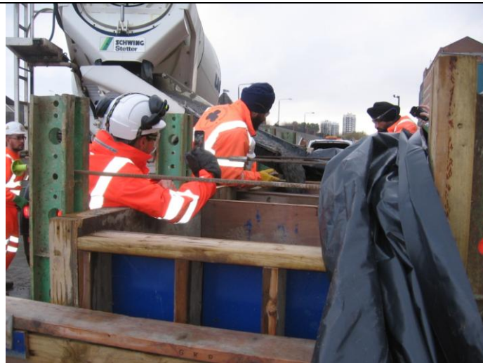
Photograph 33 Second Block Trial, discharge and placing 21st November 2013
