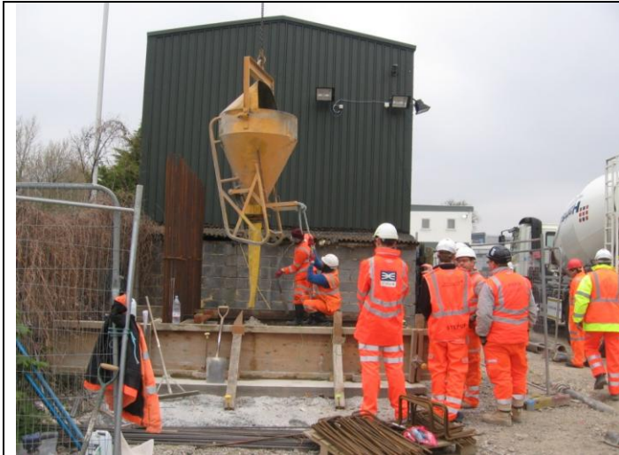
Photograph 58 Trial Panel Base Pour concreting. 4th April 2014
