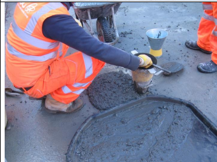
Photograph 42 Third Block Trial, slump prior to pouring 21st November 2013
