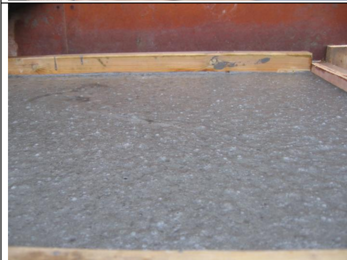
Photograph 36 Second Block Trial, float finish not applied as too workable. 21st November 2013
