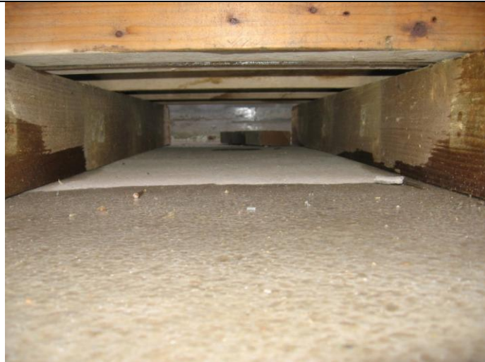
Photograph 07 Block Trial formwork, base 21st November 2013
