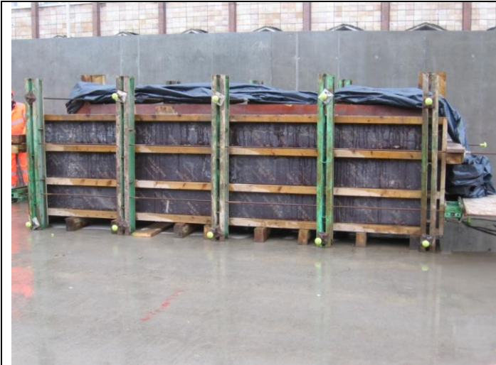
Photograph 13 Block Trial formwork 21st November 2013
