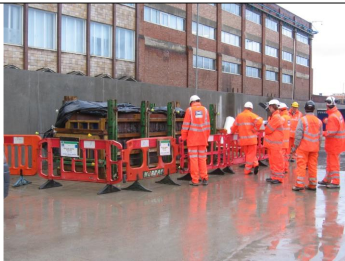
Photograph 08 Block Trial formwork 21st November 2013
