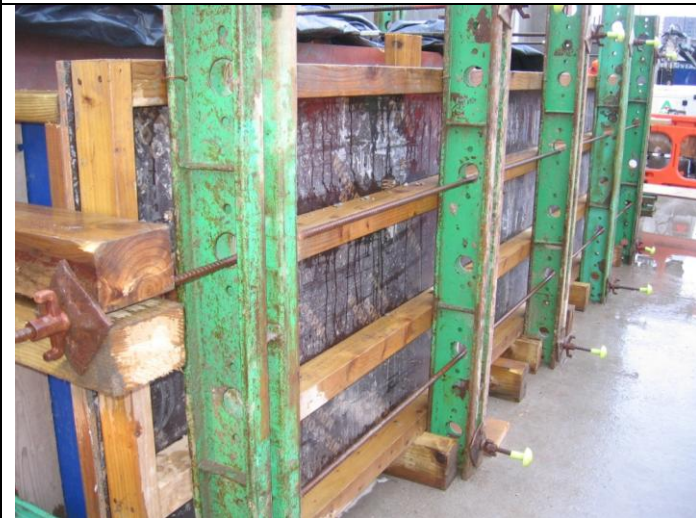
Photograph 06 Block Trial formwork 21st November 2013
