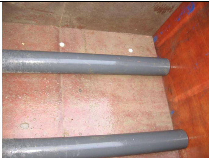
Photograph 02 Second Block Trial formwork 21 st November 2013
