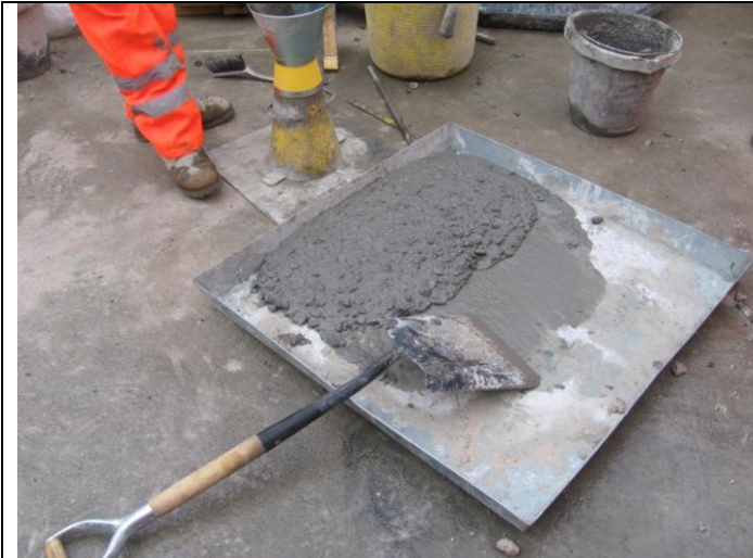
Photograph 28 Second Block Trial, slump prior to pouring 21st November 2013
