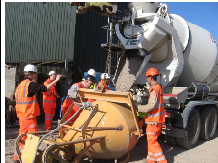
Photograph 69 Trial Panel Wall Pour concreting. 14th April 2014
