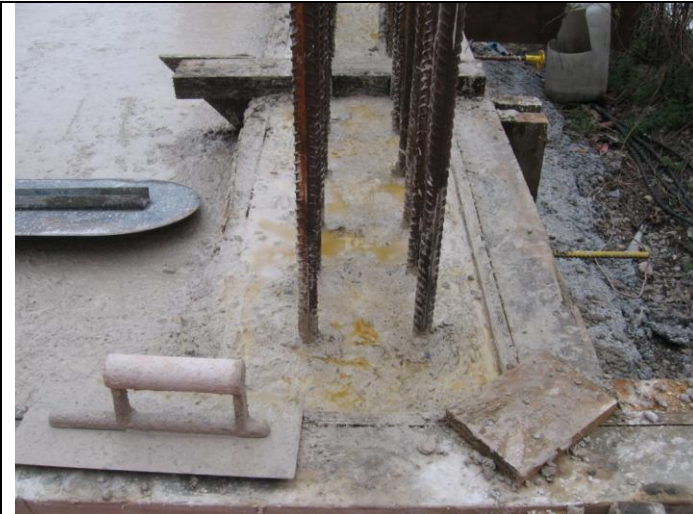
Photograph 64 Trial Panel Base Pour concreting. Finish on kicker. 4th April 2014
