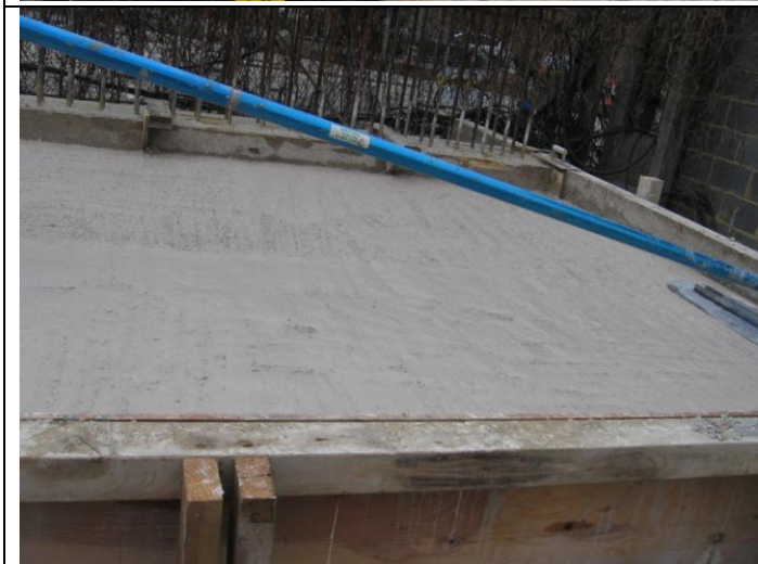
Photograph 60 Trial Panel Base Pour concreting. Surface finish 4th April 2014
