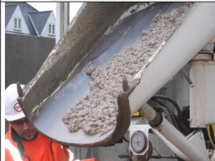
Photograph 15 First Block Trial, concrete on chute 21st November 2013
