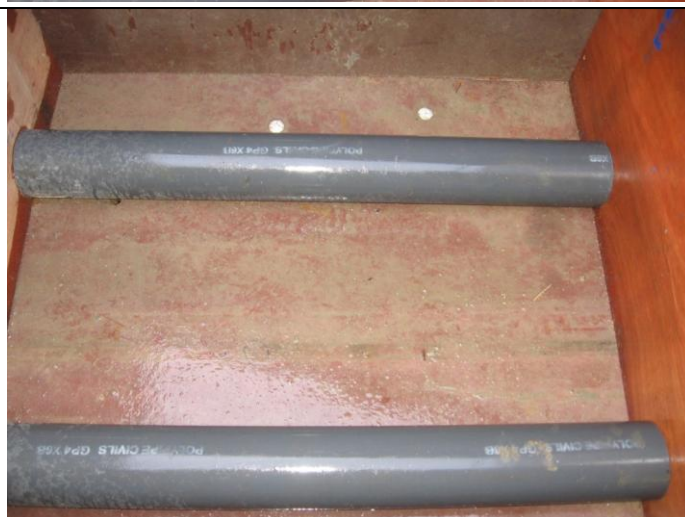
Photograph 03 Third Block Trial formwork 21 st November 2013
