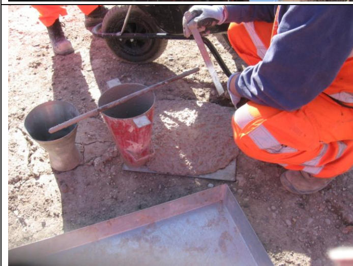
Photograph 68 Trial Panel Wall Pour initial slump test. 14th April 2014
