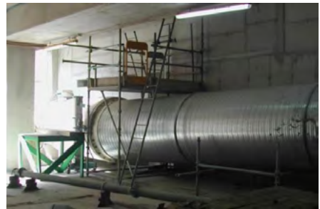
Fan at tunnel entrance with steel ducting
