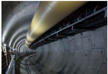
1.6 m Layflat ventilation duct to TBM
