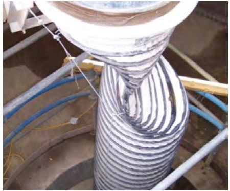
Collapsed ducting
