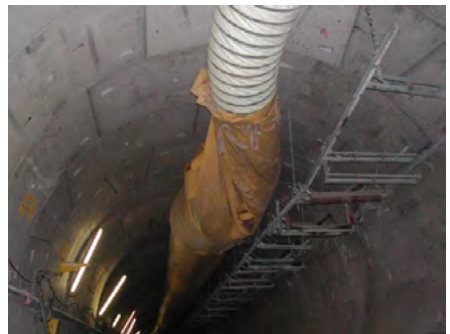
Damaged ducting
