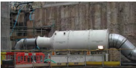
Wet de-duster at surface
