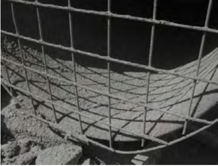
Build-up of debris on fan inlet
