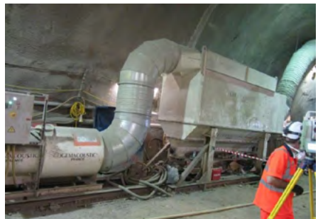
Dry de-duster underground
