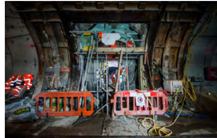
Working in limited space
