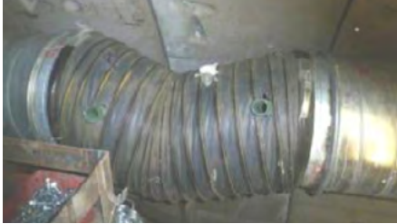
Ad-hoc air distribution system
