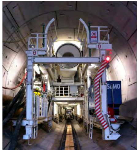
View of ducting system at rear of TBM
