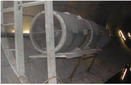
Jet Fan mounted on tunnel wall
