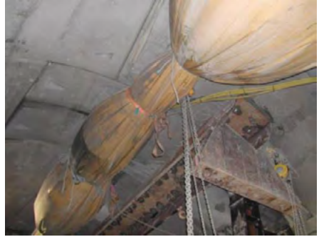
Ducting secured to protect it from damage by passing vehicles.
