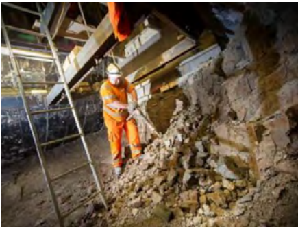
Hand mining in large opening
