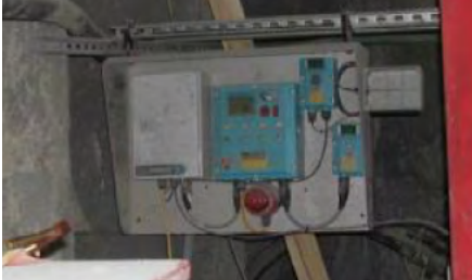
Underground gas measuring station
