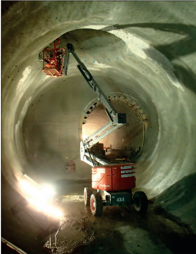
Figure 16. Ventilation tunnel VEW shaft connection into the crown of the platform tunnel
