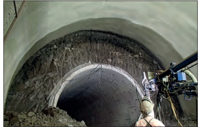
Figure 14. Sprayed concrete lining platform tunnel enlargement from a tunnel-boring machine pilot – top heading
