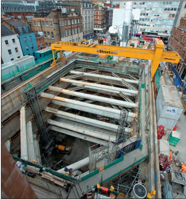
Figure 11. Tottenham Court Road western ticket hall showing gantry crane, temporary propping scheme, shotcrete batching plant with Oxford Street immediately beyond – excavation took around 9 months from January to October 2012
