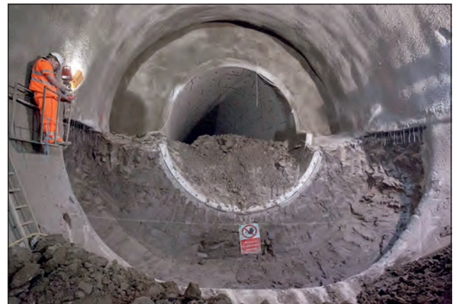
Figure 15. Sprayed concrete lining platform tunnel enlargement from a tunnel-boring machine pilot – invert
