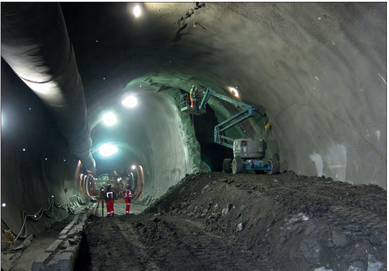
Figure 10. Final excavation stage of Whitechapel eastbound cavern
