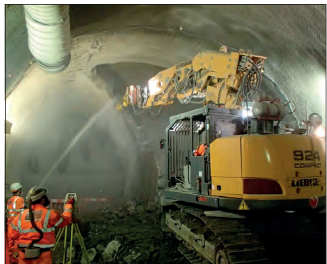
Figure 5. Removal of temporary side-drift side-wall in eastbound cavern of Stepney Green cross-over
