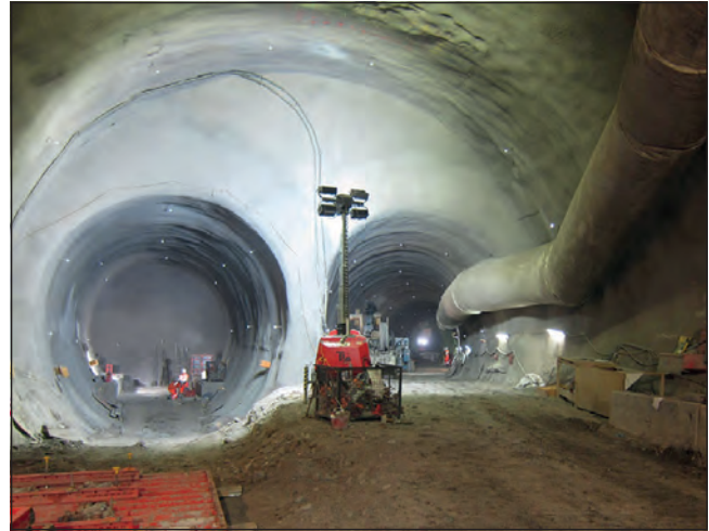
Figure 8. Completed stage 6 excavation of the larger end of the Whitechapel westbound cavern, showing tunnel boring machine launch chamber (left) and cross-over tunnel (right)
