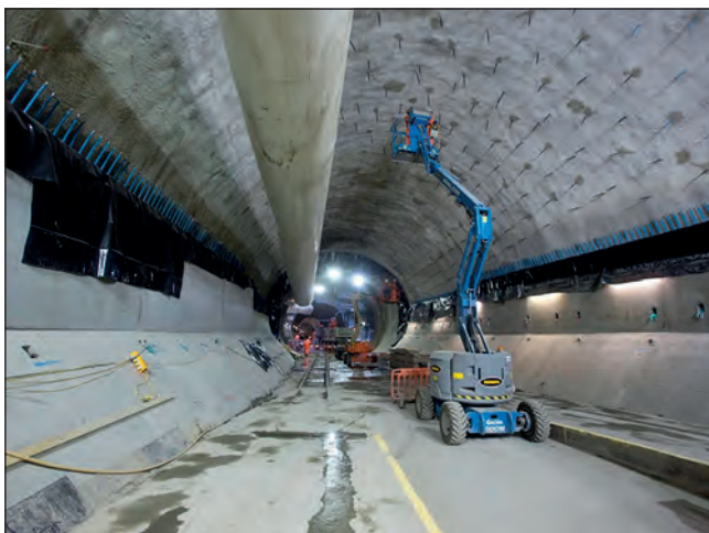
Figure 6. Stepney Green westbound cavern was waterproofed from invert to shoulder level with a PVC sheet membrane and a cast in situ steel-bar-reinforced concrete secondary lining
