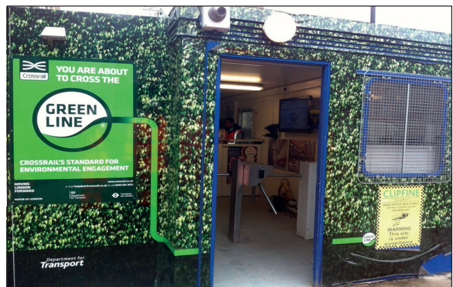
Figure 7. Green Line treatment at site entrance
