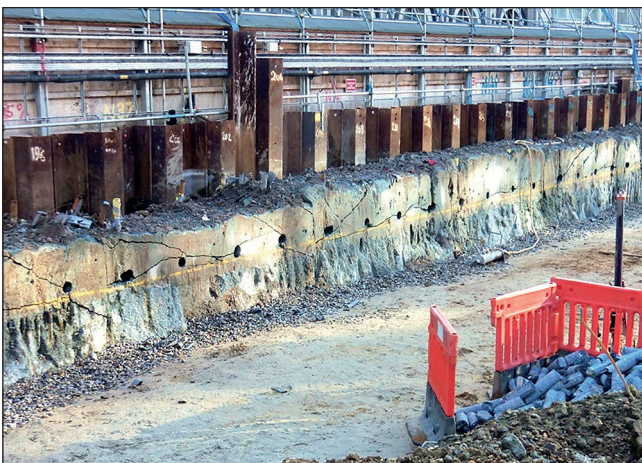
Figure 8. 'Drill-and-burst' technique for removing diaphragm wall
