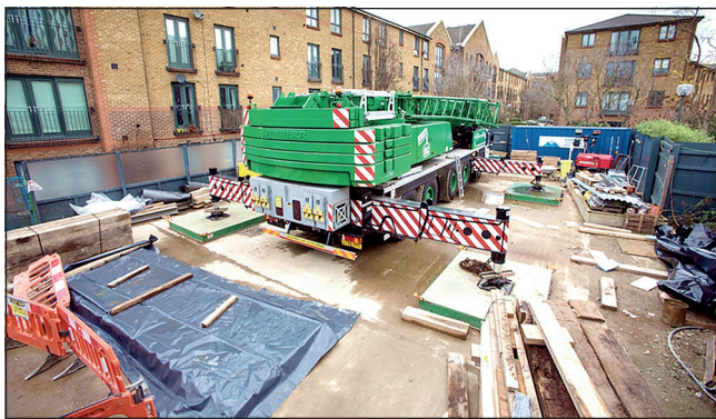
Figure 2. Construction on small sites immediately adjacent to residential properties
