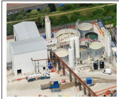
*Above: Plumstead Slurry Treatment Plant, where recycled groundwater is used for slurry dilution.*
