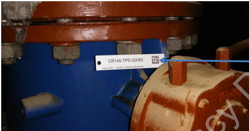
Figure 15: Typical asset tag label position for drainage valve
