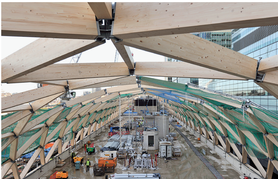
Figure 10 Timber roof under construction. Galvanised tubes that will supply air to pillows are visible from this angle, but were carefully positioned so they cannot be seen from eye level. Concrete floor forms roof to retail units below, prior to receiving waterproof membrane and soil for garden
