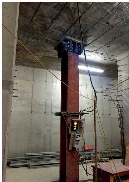
Figure 5 Collar to plunge column
