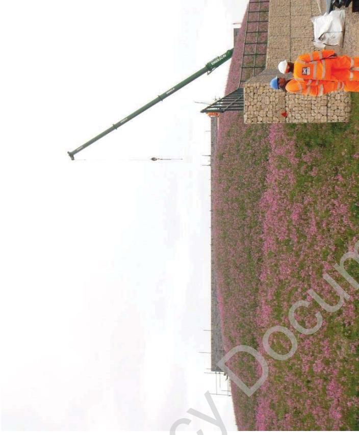
Fig 12. Limmo Peninsula Shaft mound turf and gabion handrail
