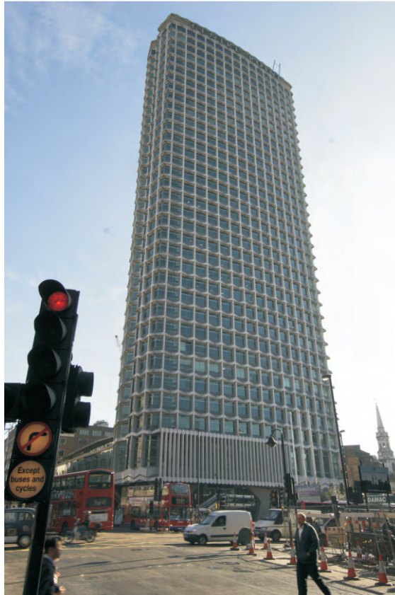
Fig 20 View of the tower from the east end of Oxford Street, looking east
