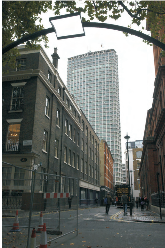
Fig 18 General view of the tower from Soho Square, looking east
