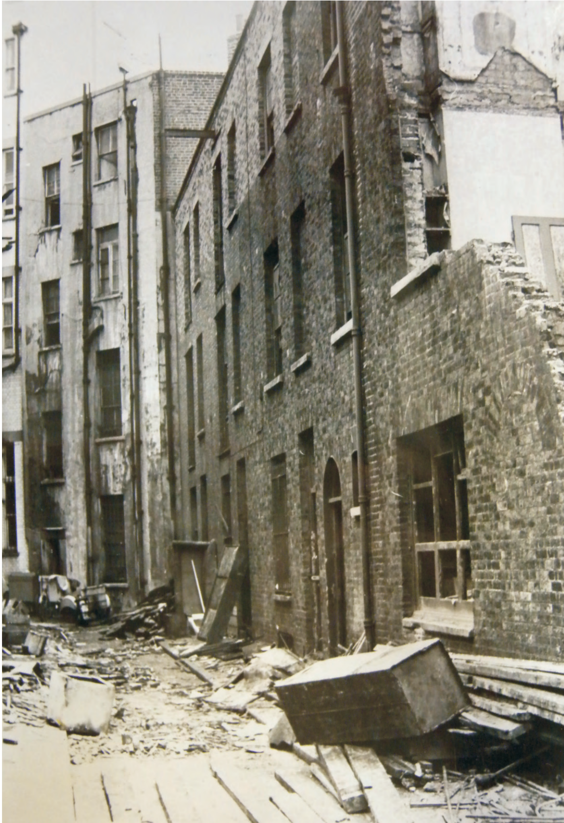
Fig 13 Lawrence Place, ca 1950s, looking north
