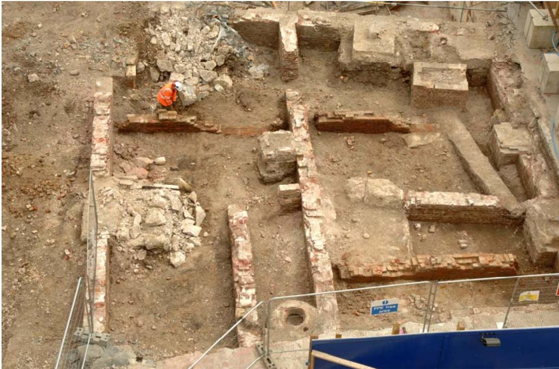
*Fig 11 View of 17th - 19th century wall foundations and circular soak-away in southern area of site, looking East*
