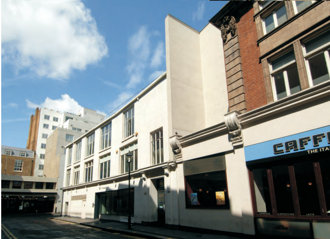
Fig 19 Building 3, looking north west. Note the recent link block between Buildings 2 and 3
