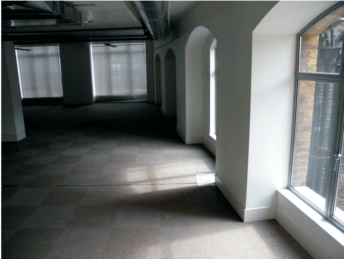
Fig 23 Two blocked and one reduced window arch in Building 1, 2nd floor, south wall, looking east
