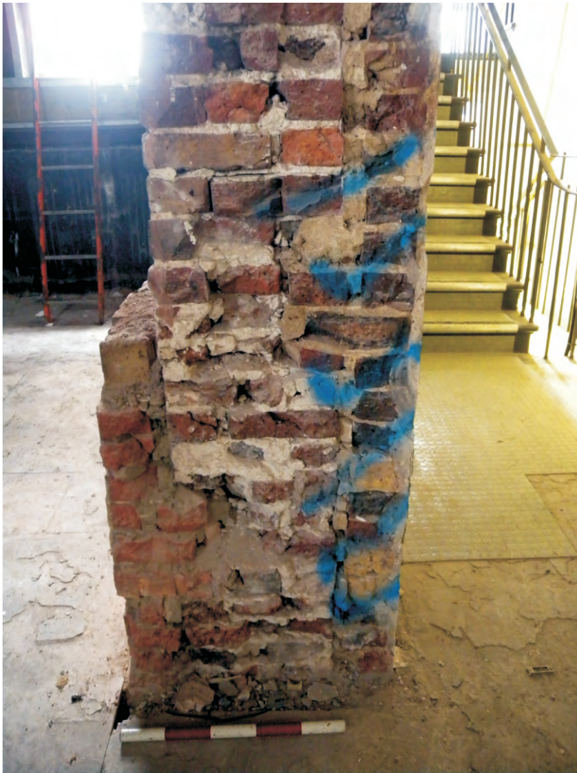
Fig 33 Partially demolished wall between Open Area 2 and Building 3 on the 1st floor, showing the skin wall of Building 3 abutting earlier masonry, looking south
