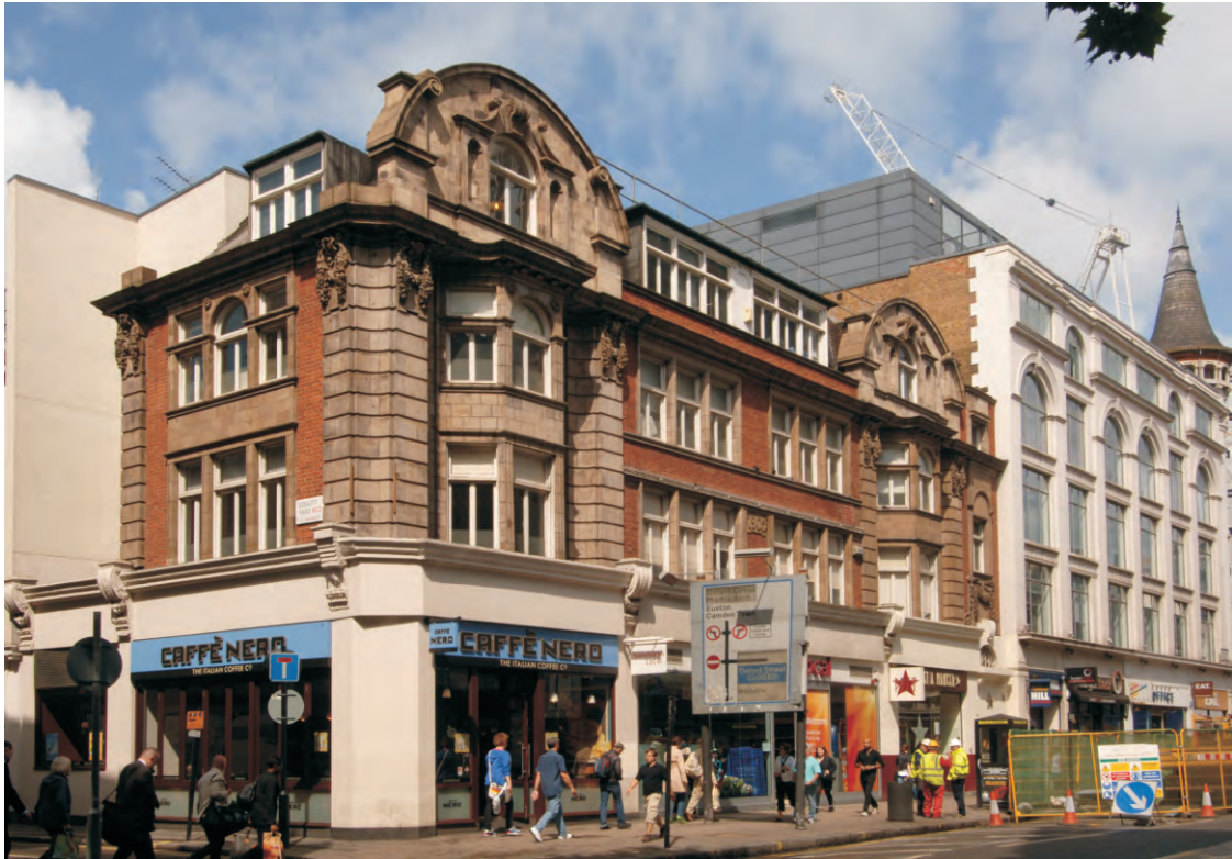
Fig 17 Building 2, looking north west
