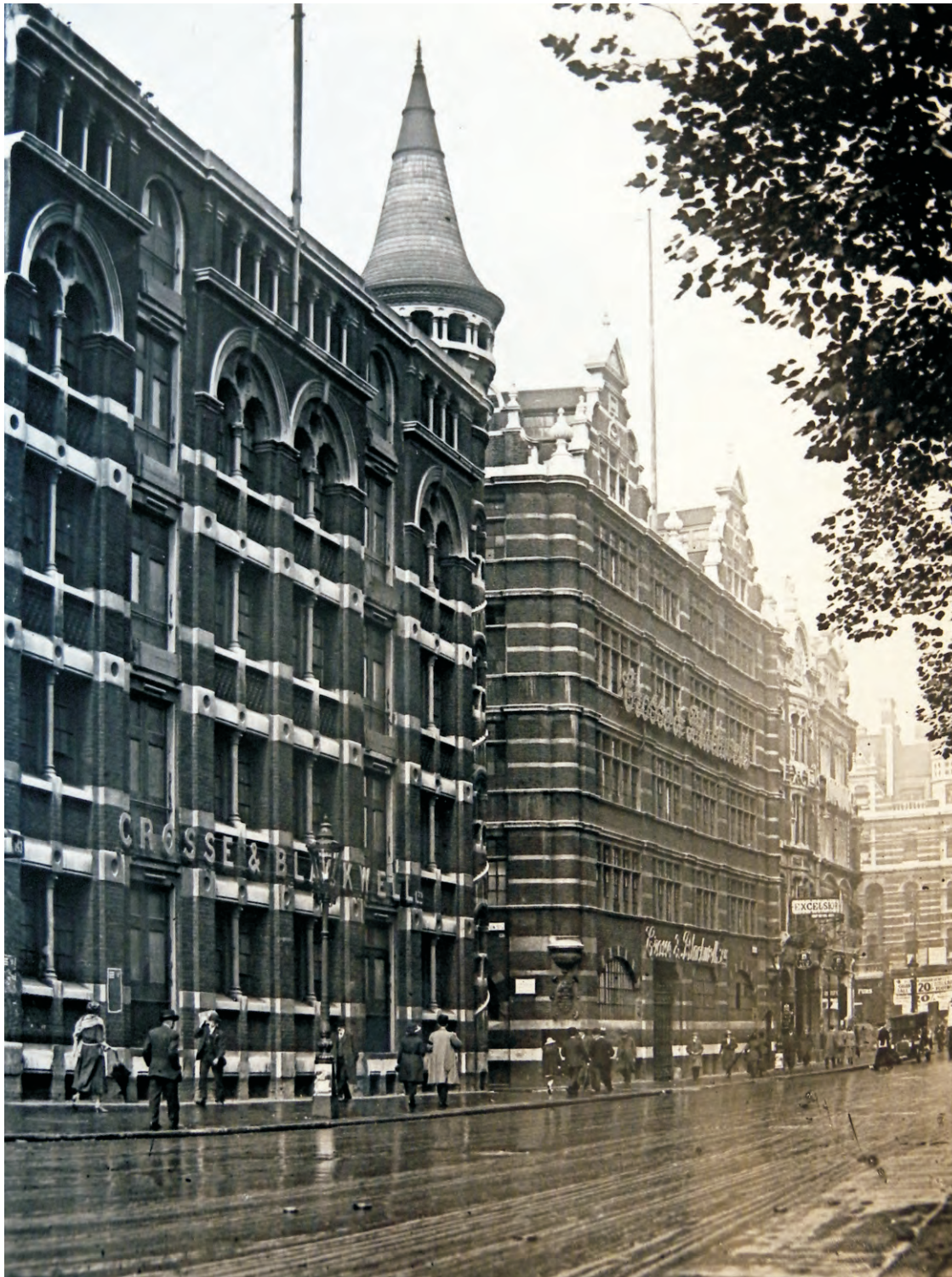
Fig 7 A photograph of the eastern façade of Building 1, when occupied by Crosse and Blackwell taken c 1920 looking north west. Compare with Fig 13
