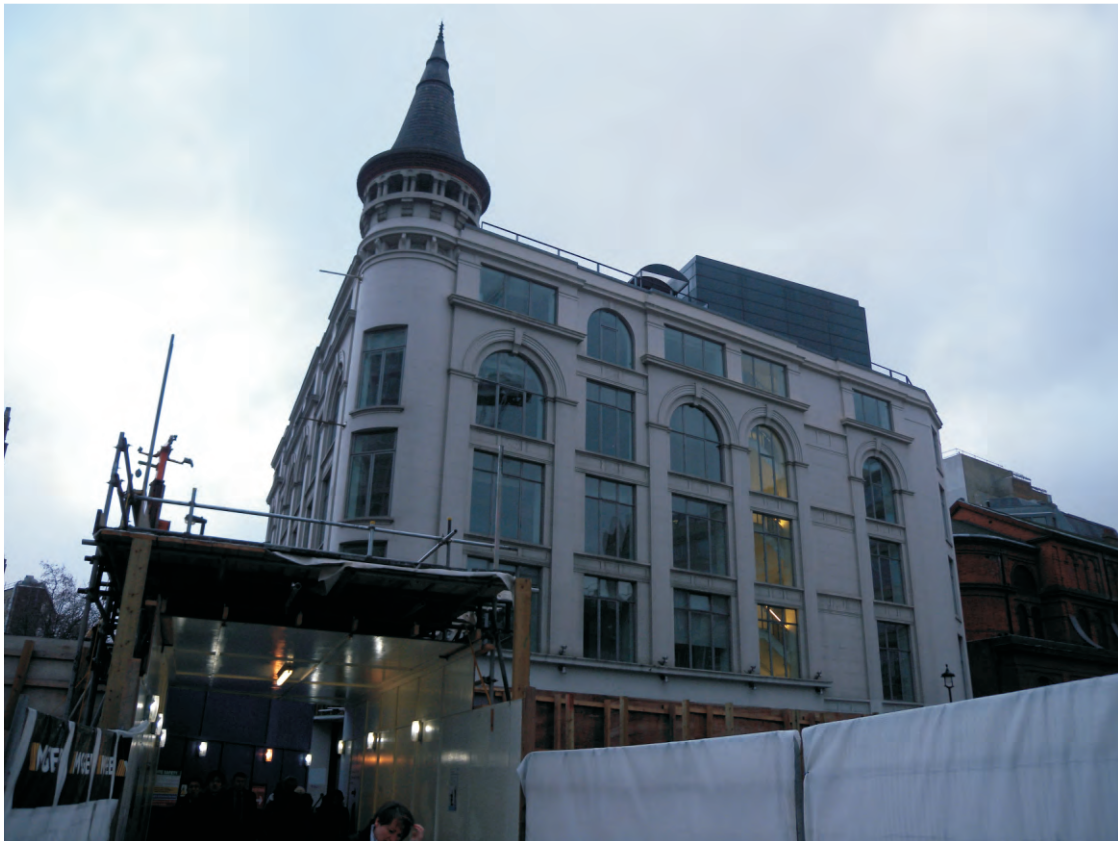
Fig 21 The North facing elevation of Building 1, looking south, after the demolition of the Astoria
