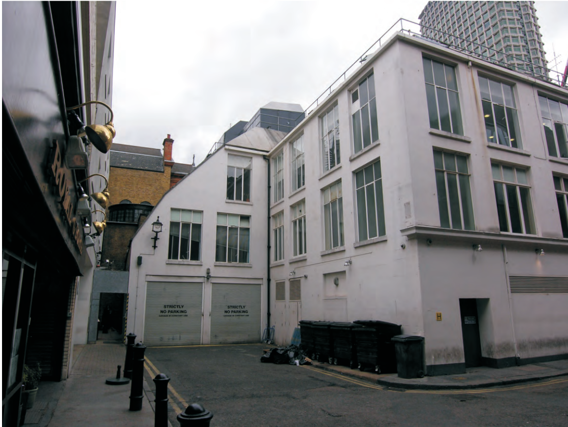
Fig 29 The western end of Building 2, looking north
