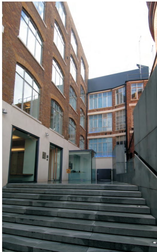
Fig 14 Open Area 1, looking south from Sutton Street
