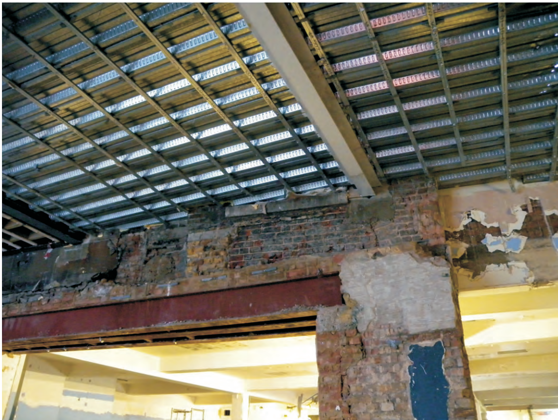
Fig 32 A small section of 19th century brickwork, likely to be the extension of the Building 1 warehouse, exposed during soft strip on the ground floor of Open Area 2, looking west
