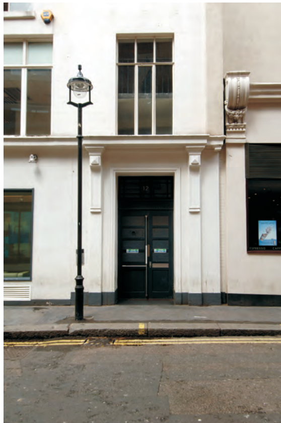
Fig 20 The original entrance to Building 3, looking north
