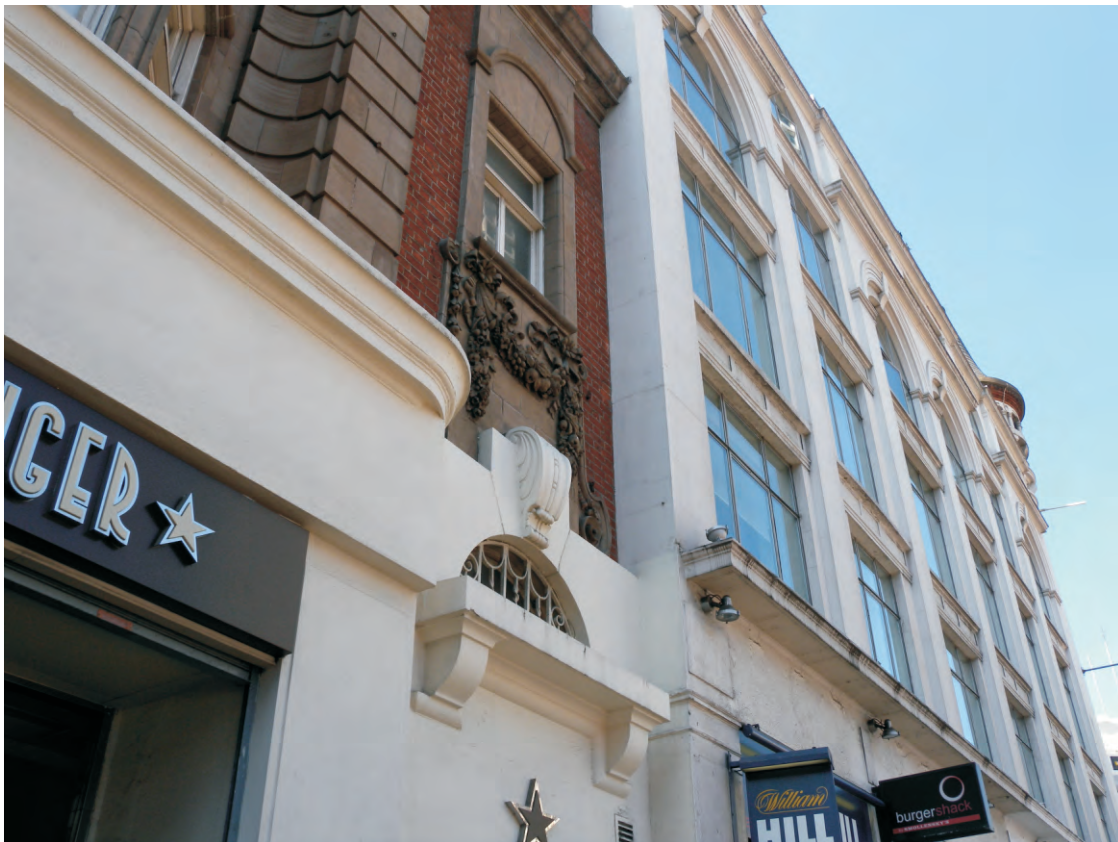
Fig 26 The original Charing Cross Road entrance to the upper floors of Building 2, looking north west
