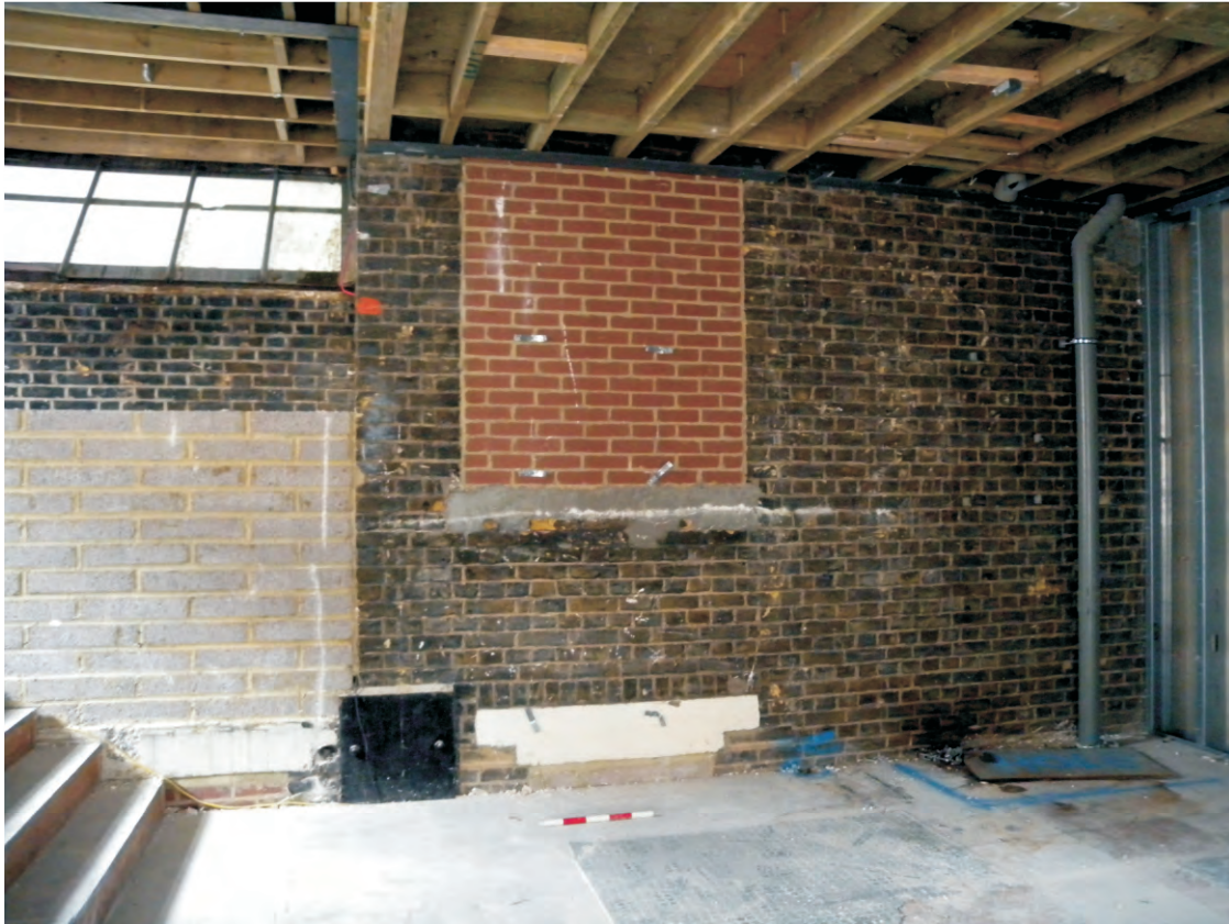
Fig 27 Blocked windows in the western wall of Building 2's 1st floor, at the southern end
