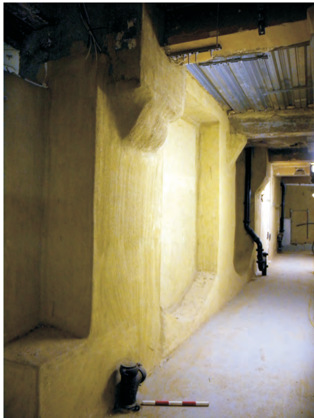
Fig 24 The west wall of Building 1 at basement level, looking north
