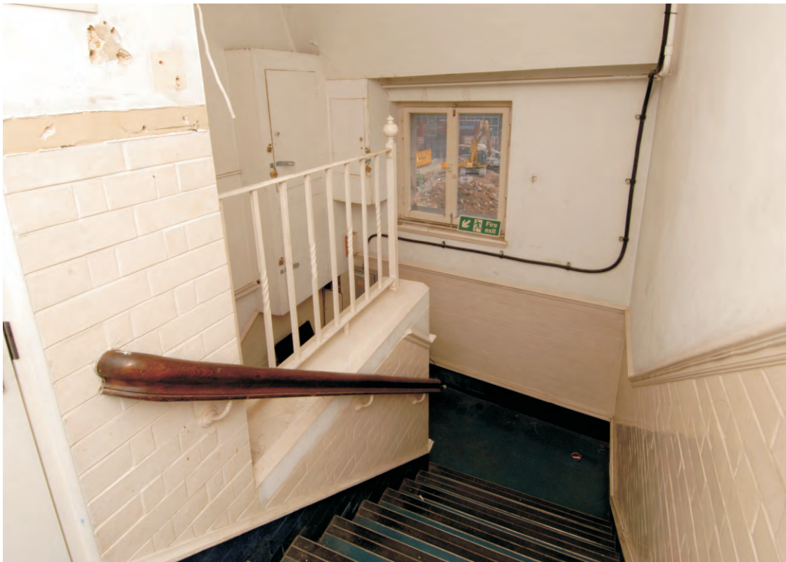
Fig 28 The top of the staircase within Building 1, looking east
