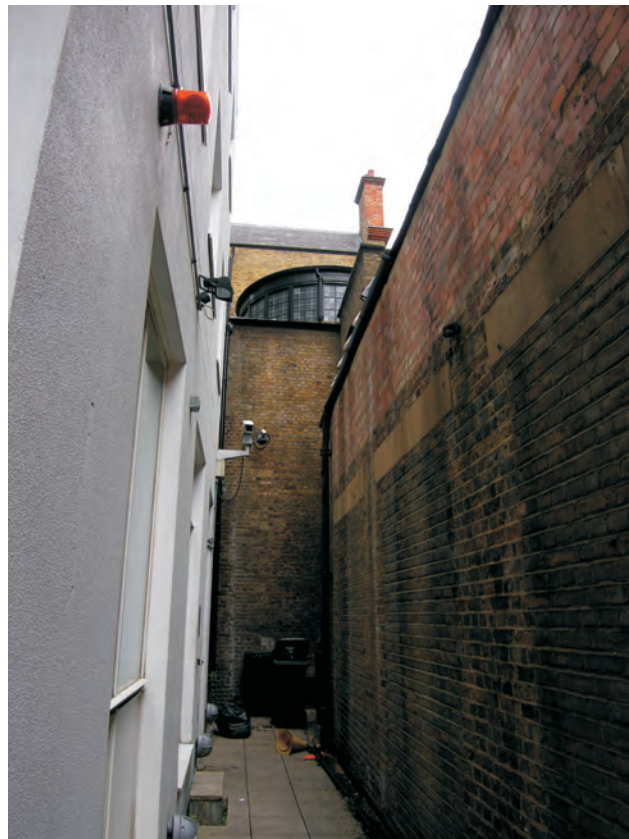
Fig 30 Blocked openings in the western wall of Building 3, looking north
