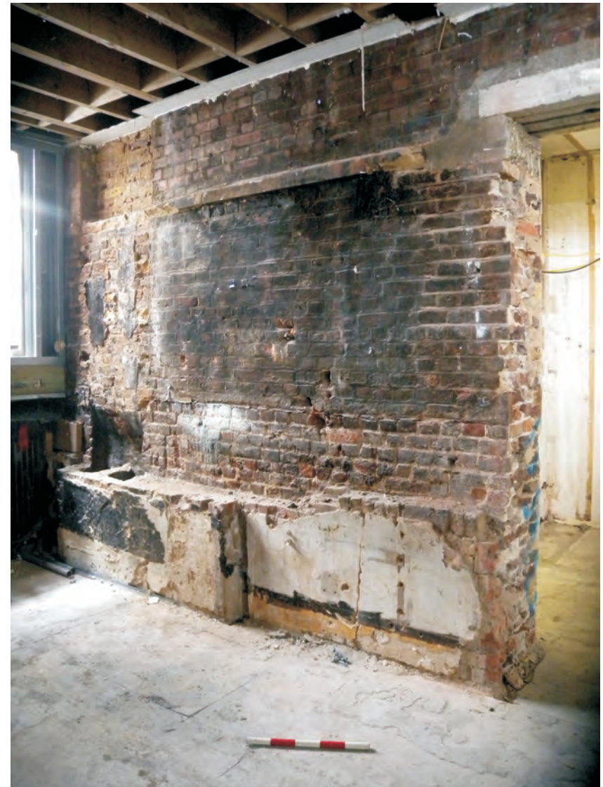
Fig 34 same section of wall, looking south west at the older masonry, with traces of a flue and an opening
