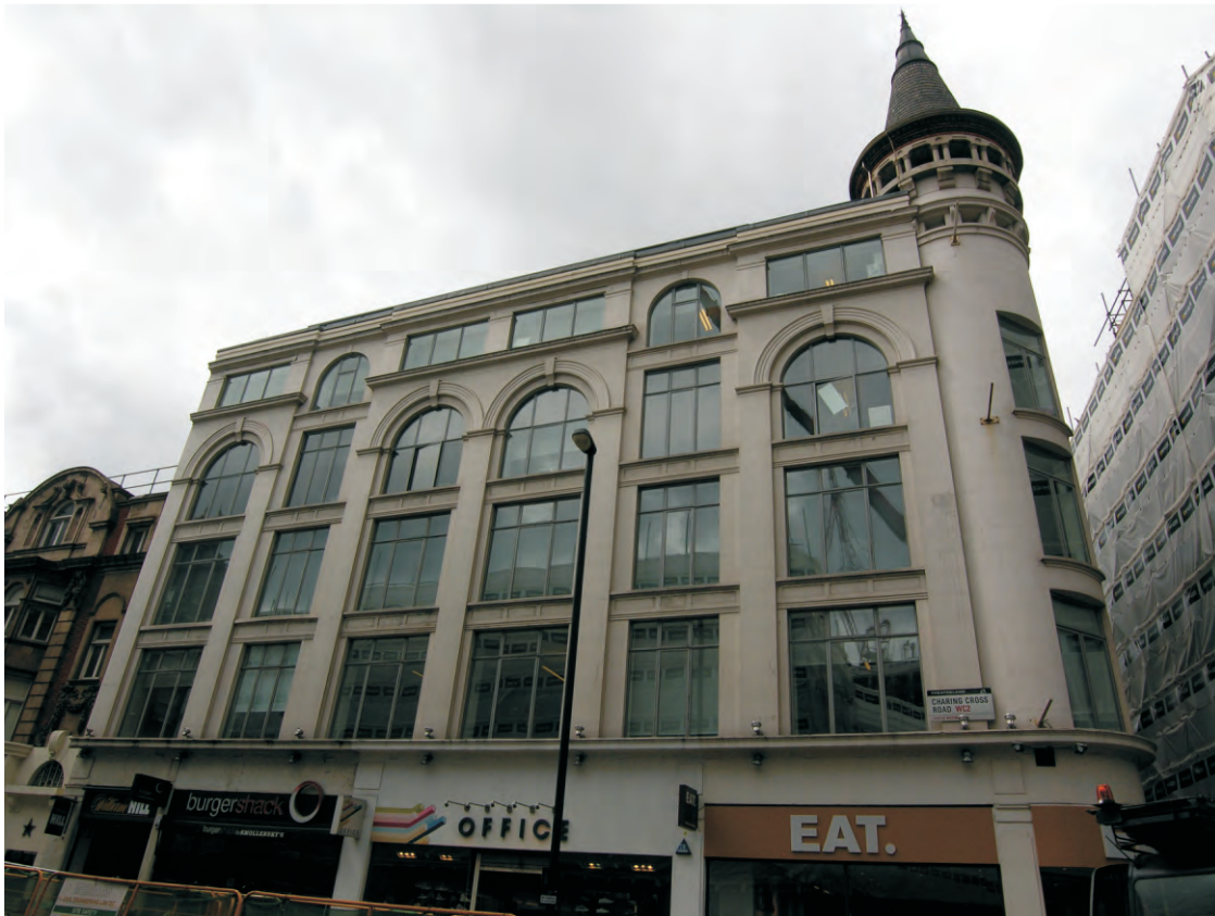
Fig 13 The east facing façade of Building 1, looking west
