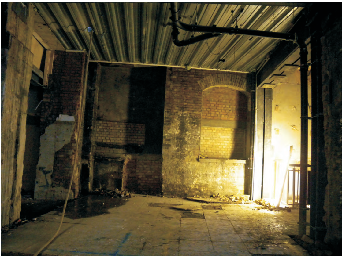
Fig 22 A loading bay and bricked up window in the south wall of Building 1, ground floor, looking north
