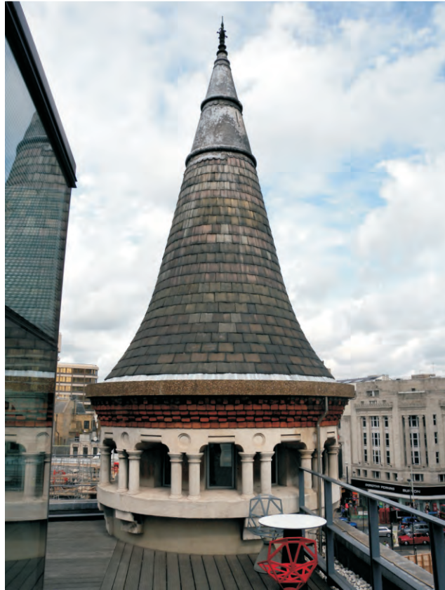
Fig 15 The turret on the north east corner of the roof of Building 1, looking north
