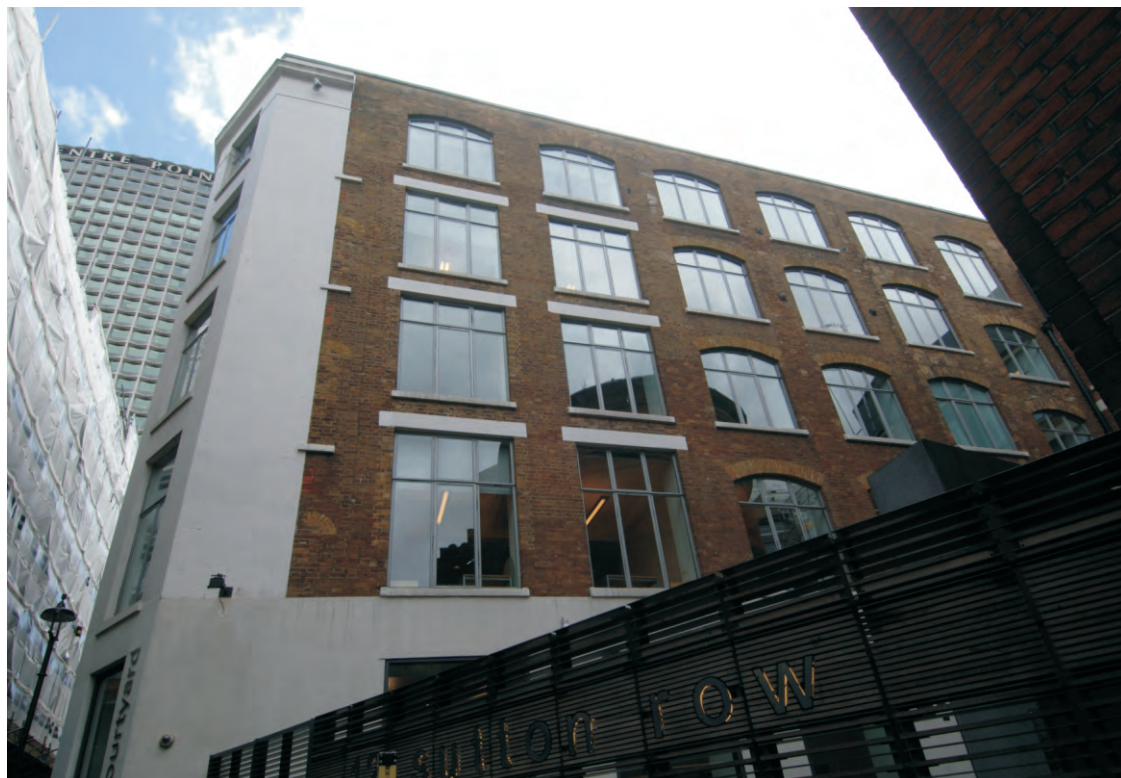
Fig 16 The western façade of Building 1, looking east
