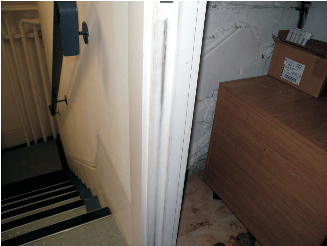
Fig 31 The top of the main staircase of Building 3, showing the change in direction of the moulded coving, into a cupboard, indicating the original direction of the stairs
