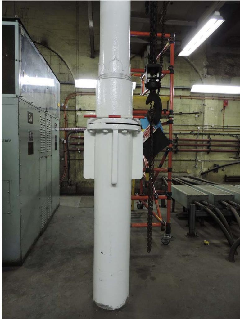
Figure 15 Column height extended due to the low level floor
