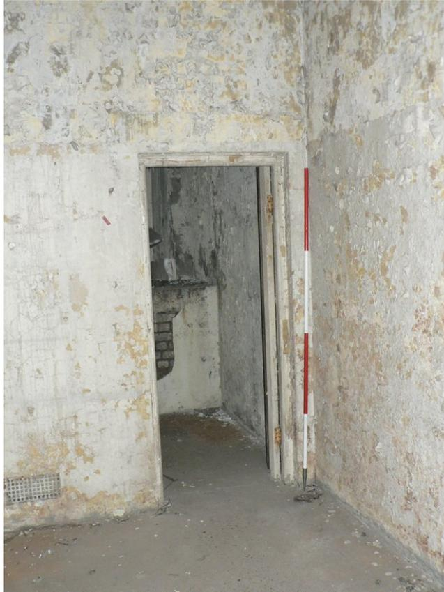
Plate 42 – Modern internal partition wall
