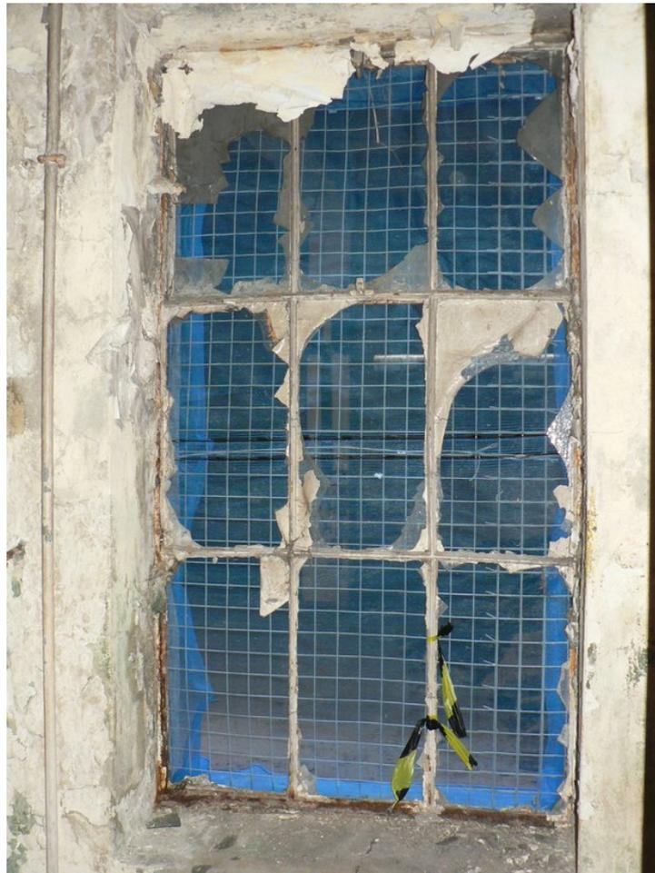
**Plate 55 – Typical metal window detail**
