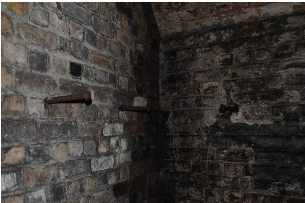
**Plate 82 – Former nail hooks within vault**
