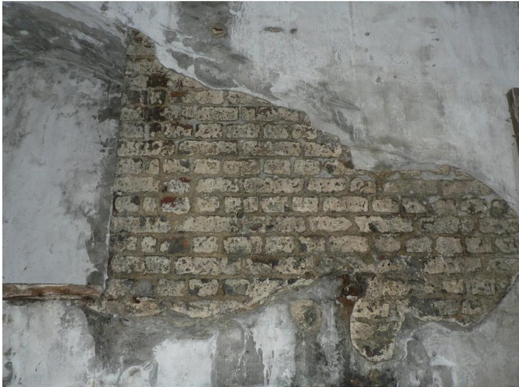
**Plate 60 – Exposed brick work showing English Bond**
