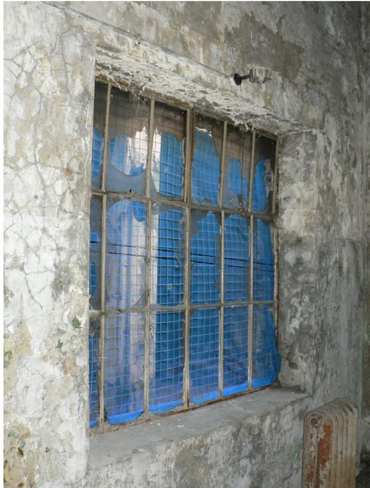
**Plate 66- Typical metal window, here with 18 panes**
