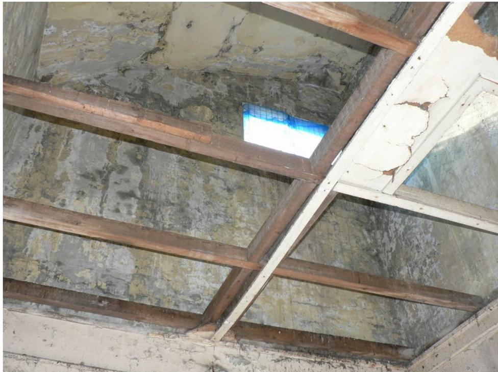
Plate 35 - Eastern section of vault showing ceiling detail and opening for previous upper storey
