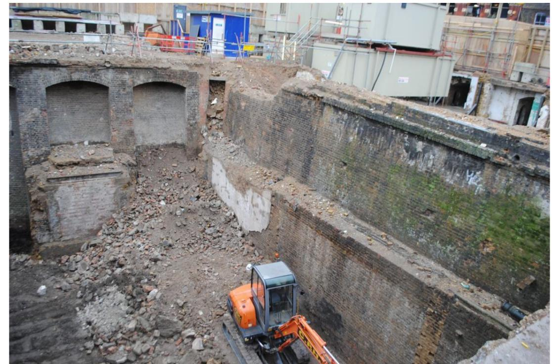
Plate 154 - Chimney and retaining walls, note void at intersection where chimney has been demolished
