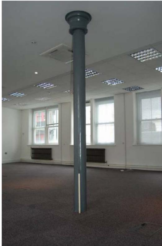
Plate 53 - 8-9 Hayne Street, cast iron column detail
