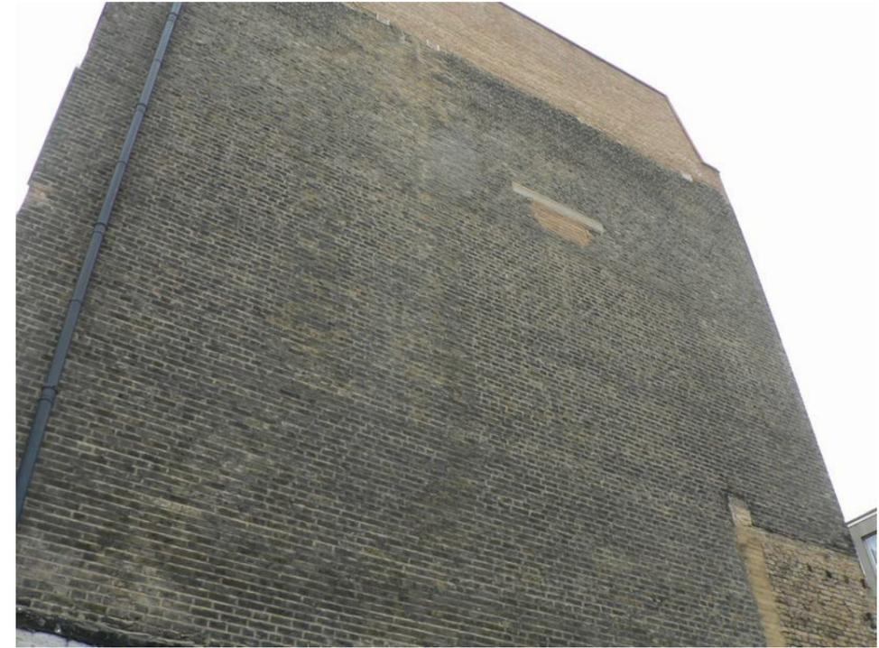
Plate 35 - 8-9 Hayne Street, northern elevation, note modern attic storey visible through modern brick
