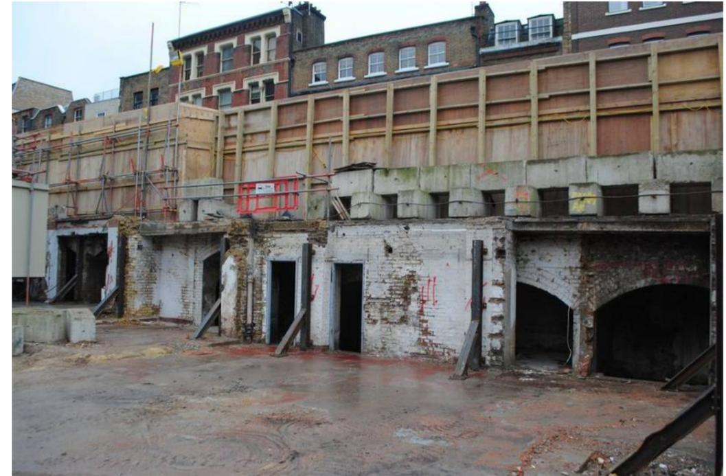
Plate 70 - 20-23 Long Lane and 22 Lindsey Street, vault detail post demolition
