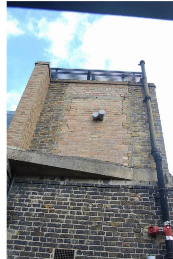
Plate 39 - 8-9 Hayne Street, view to rear, blocked up door that previously housed a bridge to 2 Lindsey Street
