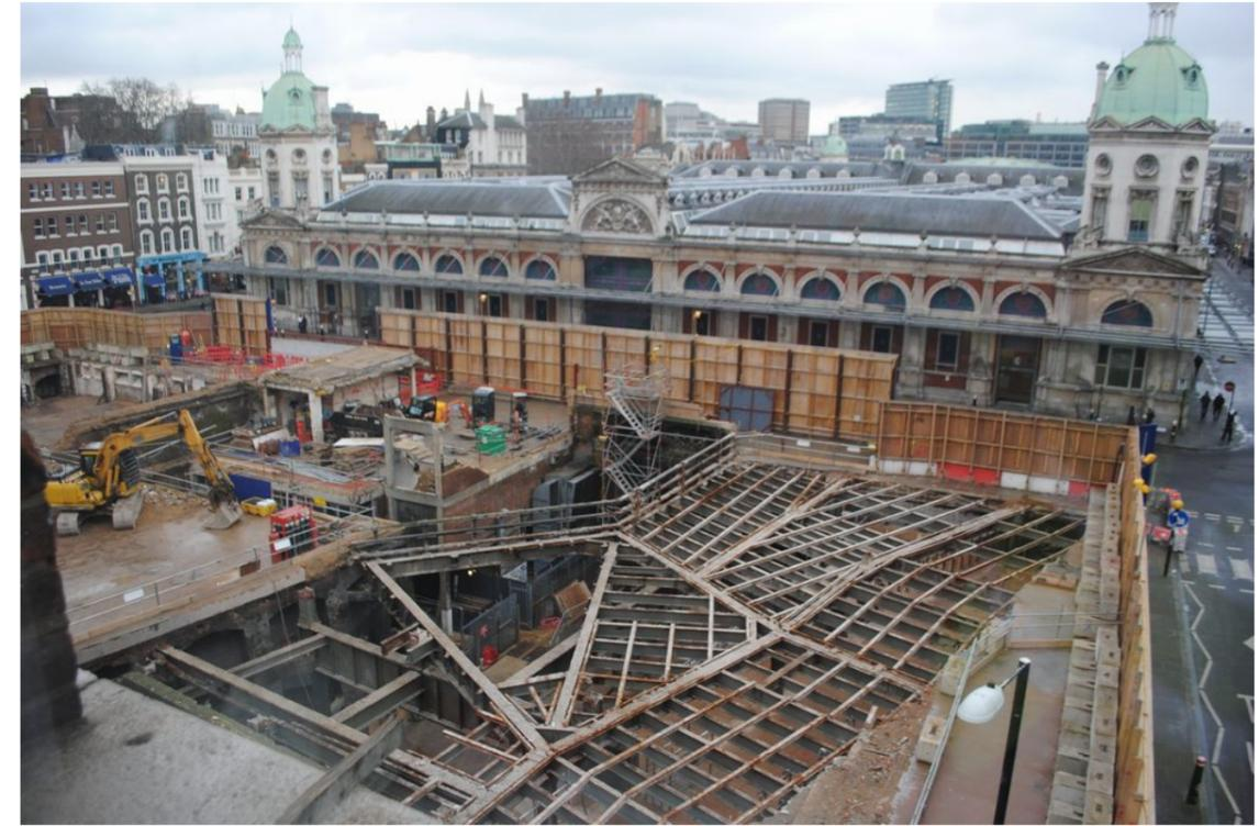
Plate 30 - 54-64 Charterhouse Street, post demolition showing decking structure upon which the structure sat
