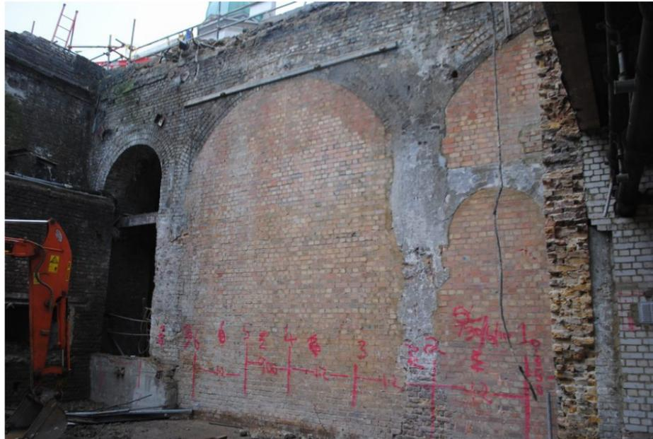
Plate 130 - 3 Lindsey Street, blocked up arches to platform level
