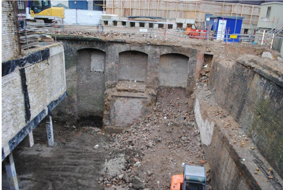
Plate 155 - Chimney and retaining walls, note void at intersection where chimney has been demolished
