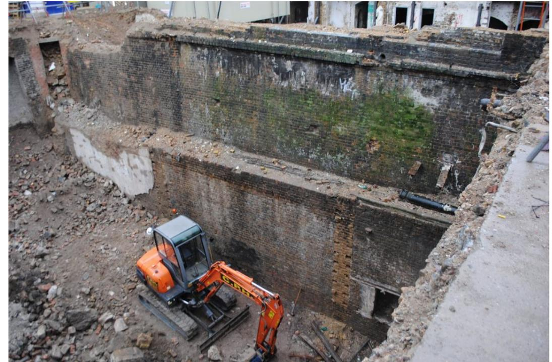
Plate 153 - Chimney and retaining walls, note void at intersection where chimney has been demolished
