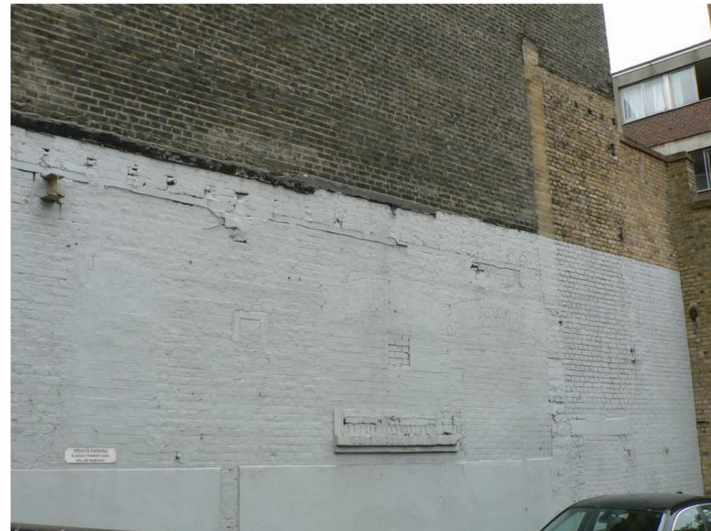
Plate 36 - 8-9 Hayne Street, showing blocked up apertures that used to lead into 10 Hayne Street, note also scarring to right of photo showing former roof over railway sidings
