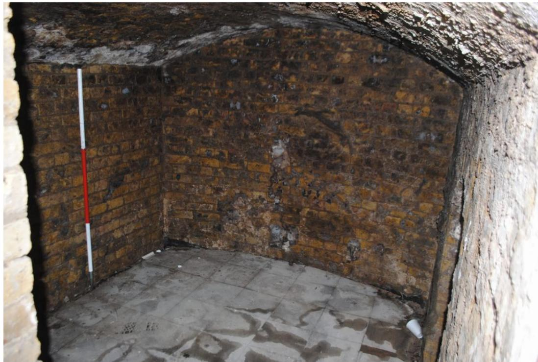
Plate 77 - 20-23 Long Lane and 22 Lindsey Street, vault detail post demolition
