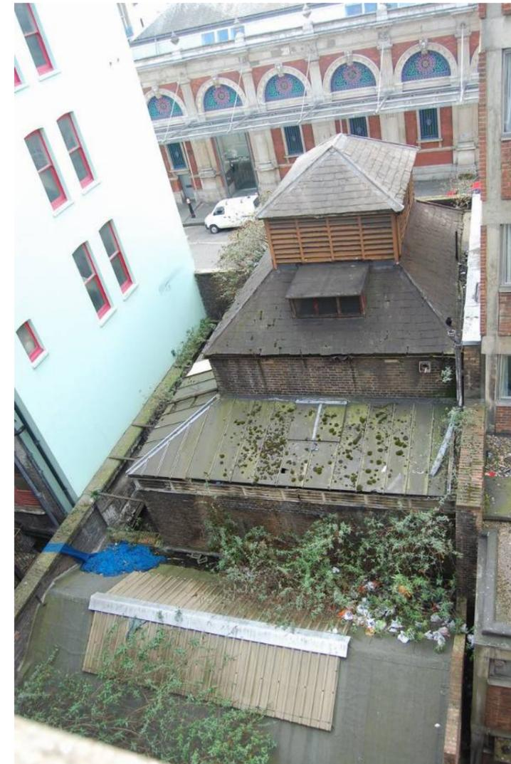
Plate 113 - 3 Lindsey Street, rear view showing main body of structure surrounded by lower toilet block
