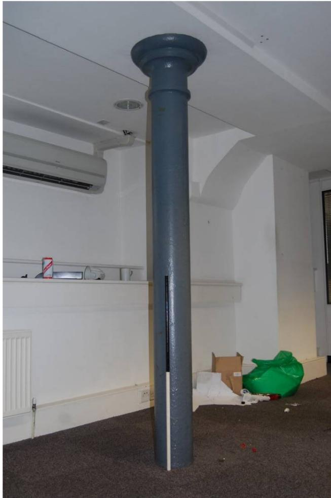
Plate 43 - 8-9 Hayne Street, cast iron column detail
