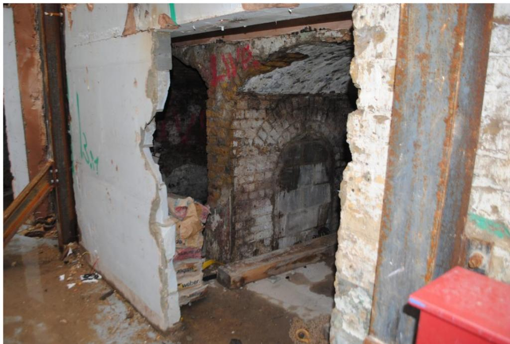
Plate 73 - 20-23 Long Lane and 22 Lindsey Street, vault detail post demolition
