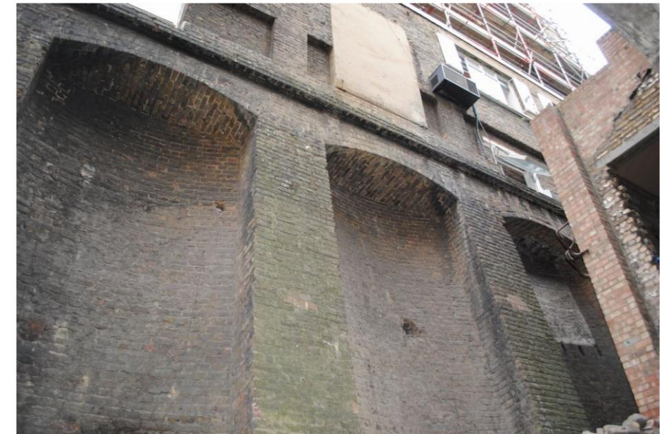
Plate 158 - Chimney and retaining walls, eastern wall detail, showing boarded up door above that linked 8-9 Hayne Street with the former GWR building
