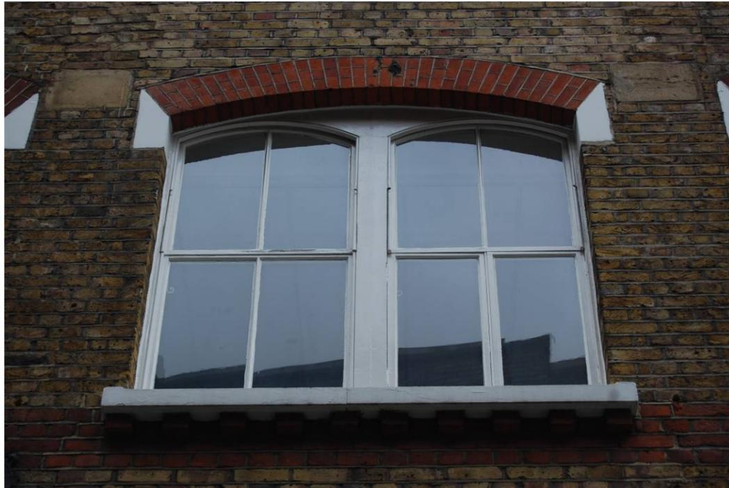
Plate 34 - 8-9 Hayne Street, inserted window after removal of walkway. Note stones either side of lintel
