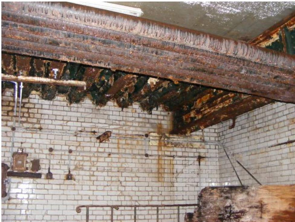
Fig. 16 View of ceiling/roof over well showing roofing materials and electrical conduits and condition resulting from severe water ingress.
