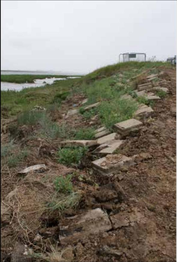
Plate 22: Breach 3. Seaward base of existing sea wall showing disturbed concrete Essex block facing and rough hewn stones along the toe of the clay bank
