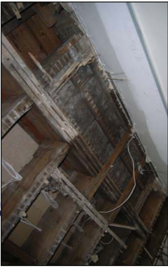
Plate 6: Underside of hearth in floor
