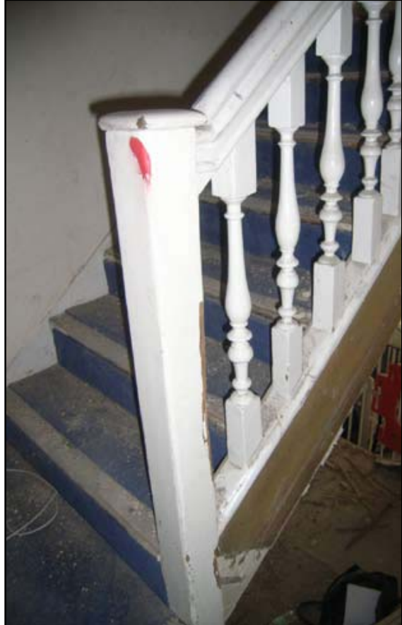
Plate 12: Stairs rising up to first floor level
