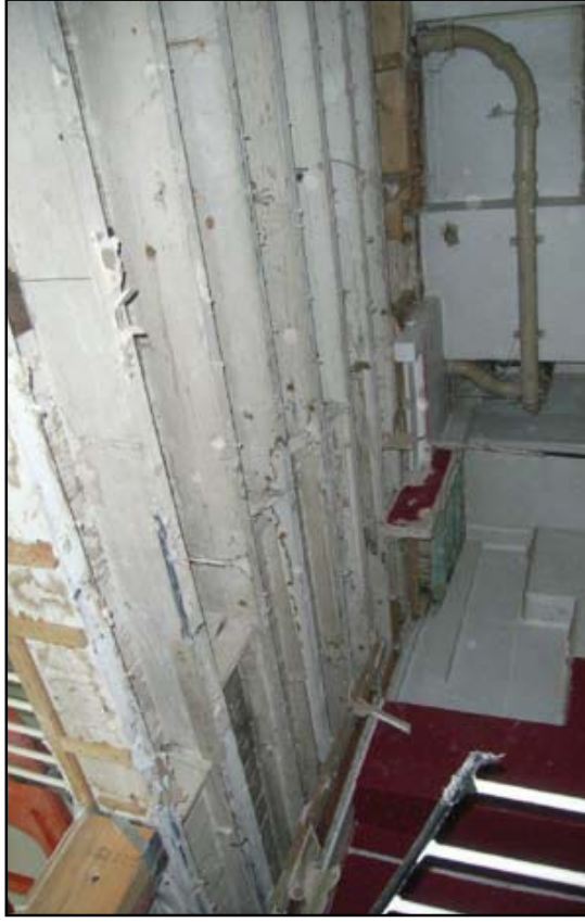
Plate 1: Basement of 5 Great Chapel Street
