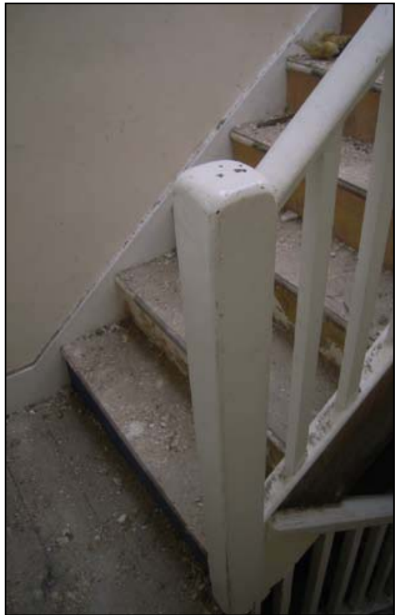
Plate 16: Plainer stairs rising towards 3rd floor
