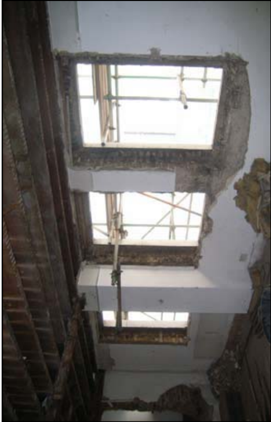
Plate 21: Removed windows at 2nd floor
