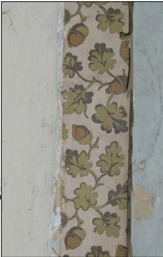
Plate 13: Exposed floor fragment of wallpaper where stair partition removed
