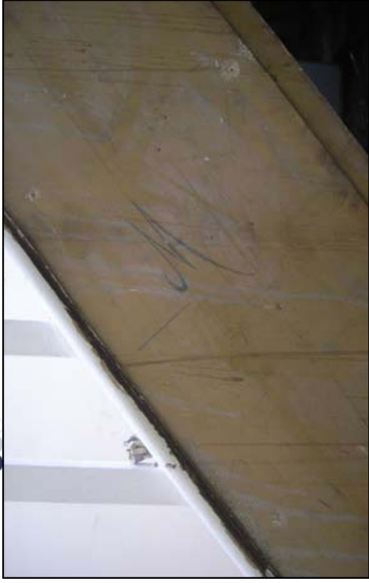
Plate 18: Initial uncovered on board to side of stairs
