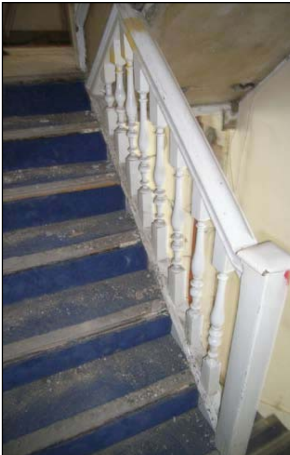
Plate 15: Stairs rising up to first floor
