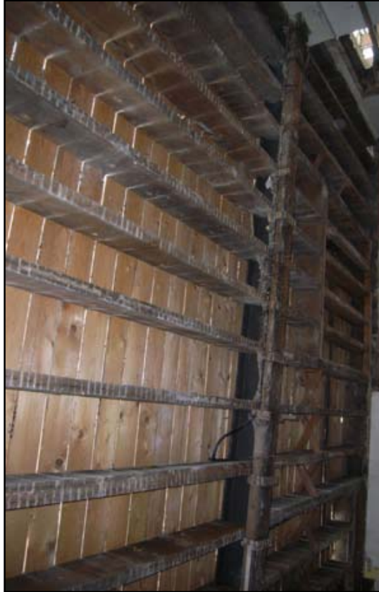
Plate 7: General view of exposed floor joists
