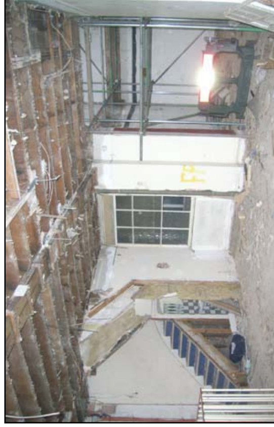
Plate 4: Ground floor after softstrip
