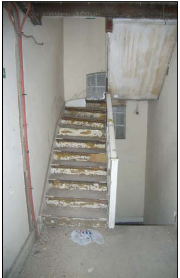
Plate 14: Stairs at first
