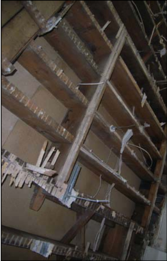
Plate 5: Underside of former hatch in floor joists
