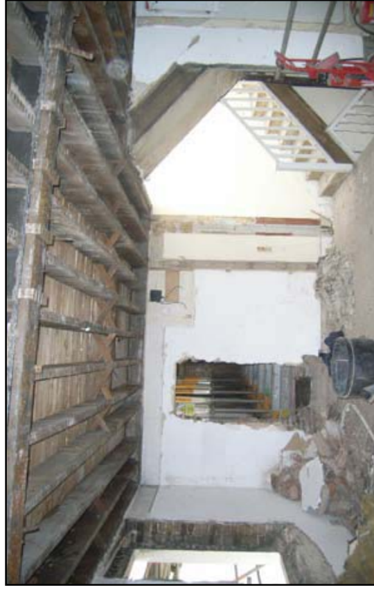
Plate 20: General view of 2nd floor
