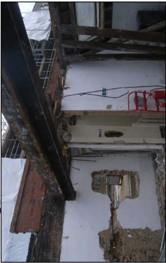
Plate 26: General view at third floor
