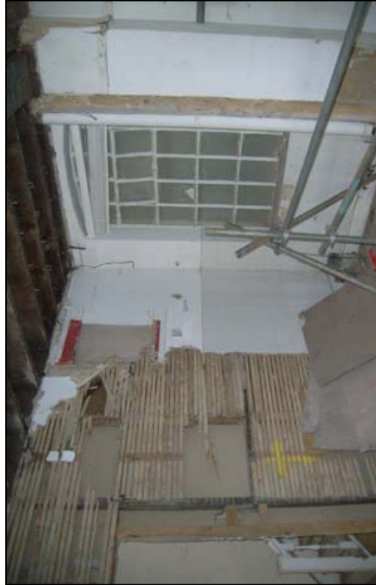
Plate 23: View at first floor
