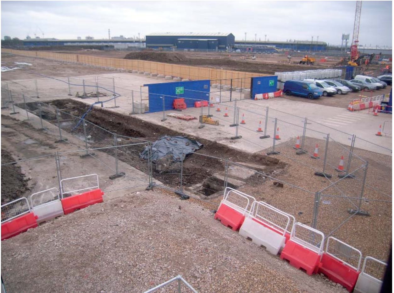
Plate 29: Trench 12. Overall view of trench from NW
