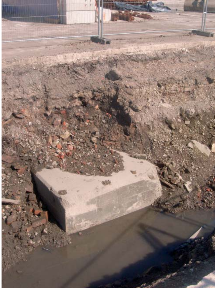
Plate 41: Trench 12. Concrete base of turntable's central pivot. Looking N
