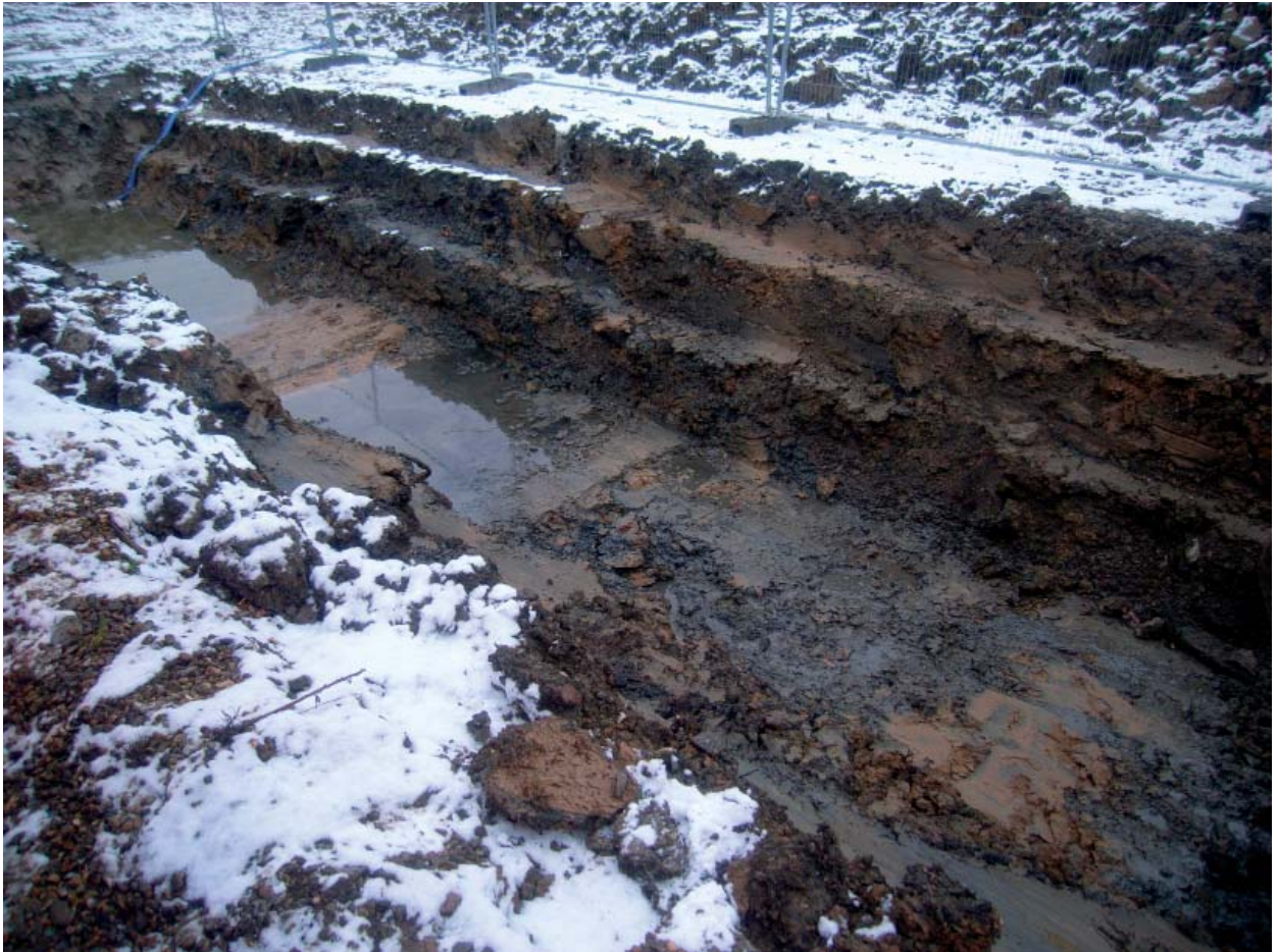
Plate 27: Trench 11. View of excavated trench looking W. Showing recent "madeground" deposit (1101) over Natural clay (1102)
