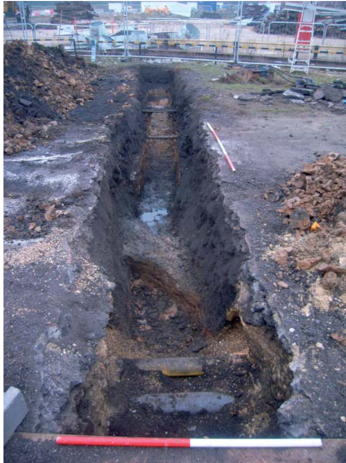
Plate 11: Trench 6. Southern end of trench looking north. Concrete encased water main [604] in foreground
