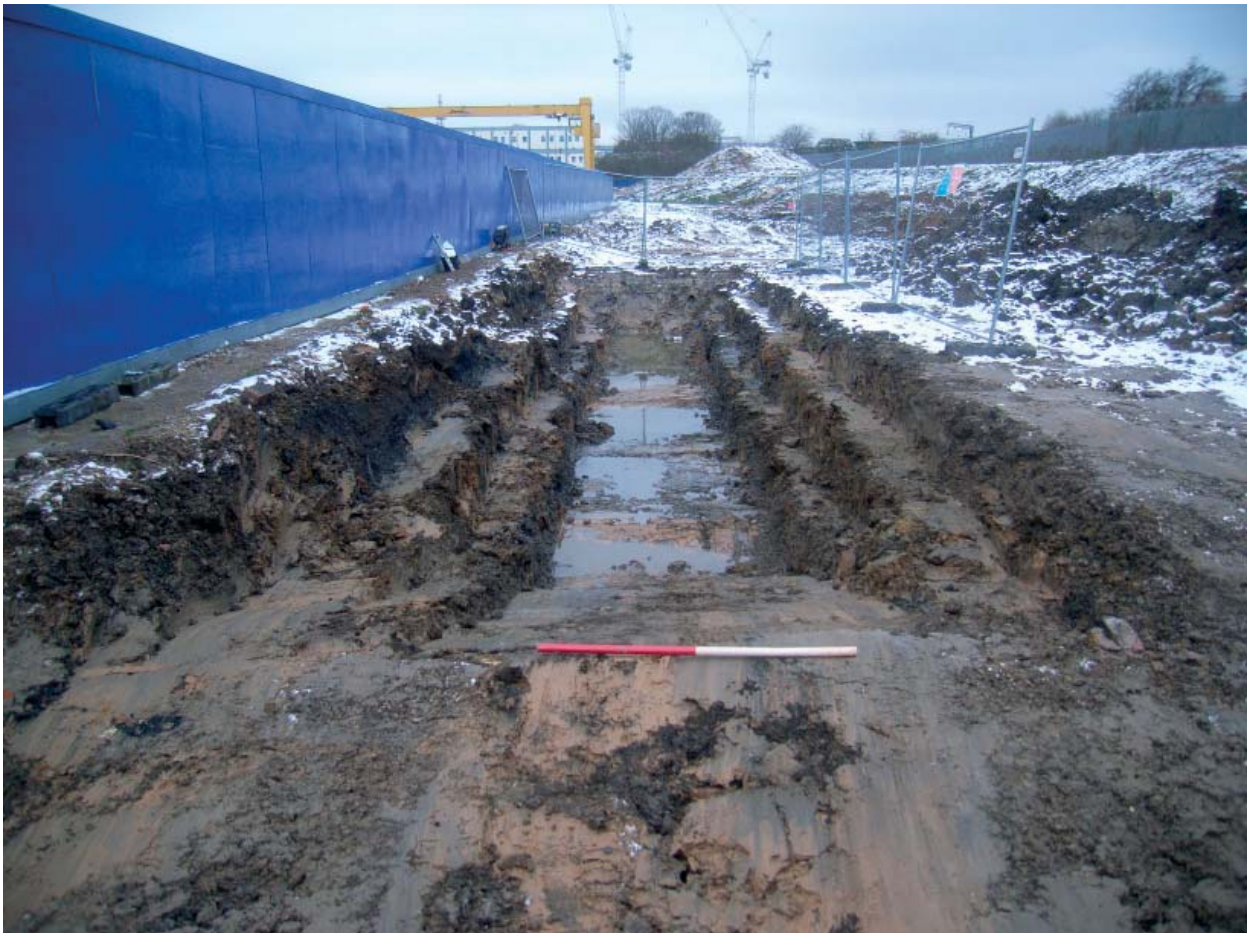
Plate 28: Trench 11. Base of trench looking N. Showing recent "madeground" deposit (1101) over Natural clay (1102)
