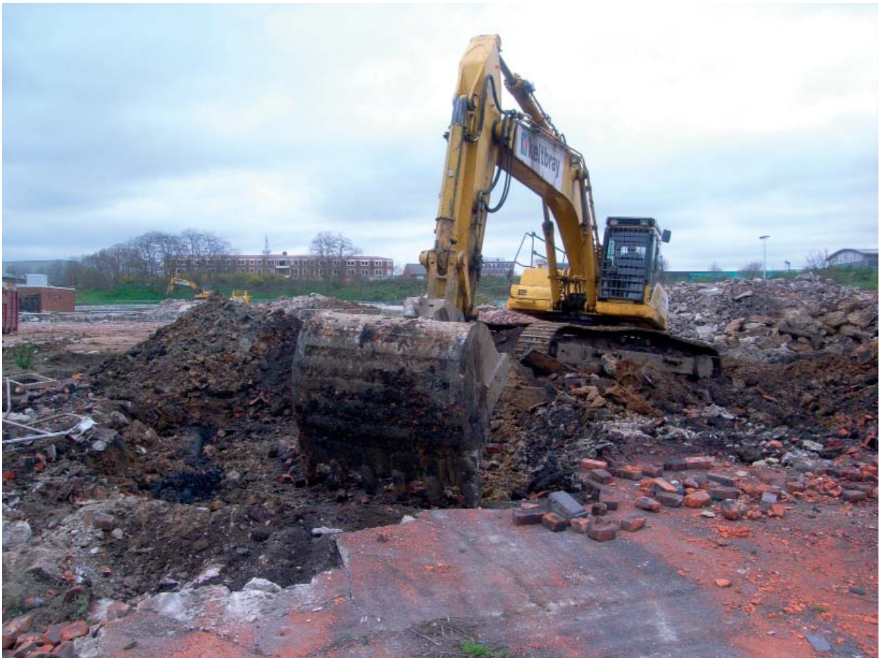
Plate 24: Trench 10. Concrete plinth [1002] for roof column of 1906 Engine Shed. Showing bolts for column and central hole for vertical down drain pipe
