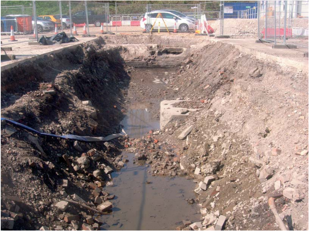
Plate 43: Trench 12. Overview of trench from E. Showing pivot base [1203] turntable floor (1223) and W turntable sidewall [1235]
