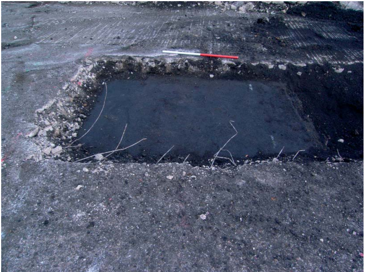
Plate 4: Trench 2. Looking north. Former concrete roadway (203)
