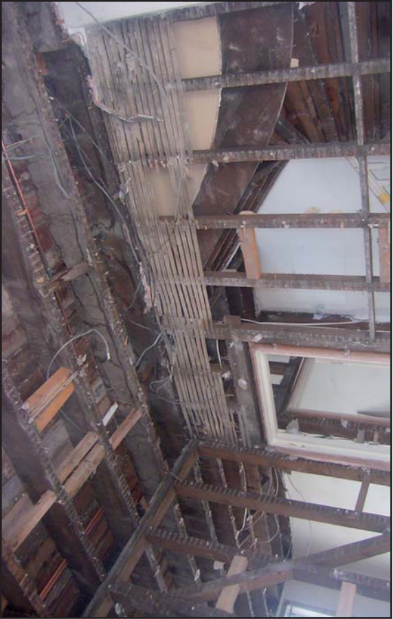
Plate 78: Partitions at 2nd floor (July 2010)
