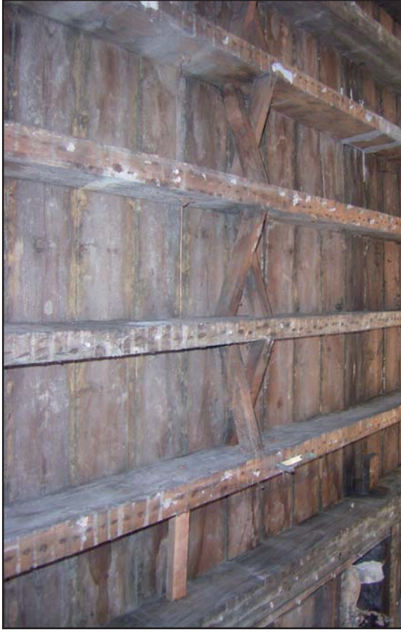
Plate 73: Scissors struts in 2nd floor structure (July 2010)
