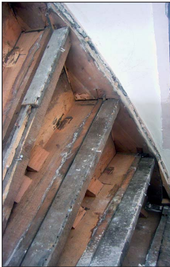
Plate 83: Staircase detail during soft strip (July 2010)
