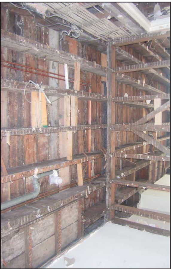
Plate 77: Partition at 2nd floor (July 2010)
