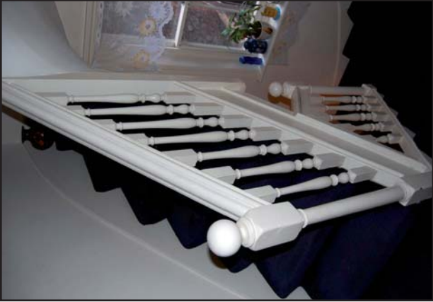
Plate 53: Staircase showing ball finial to newel post, bannisters and handrail with raised central profile, second floor (Jan 09)
