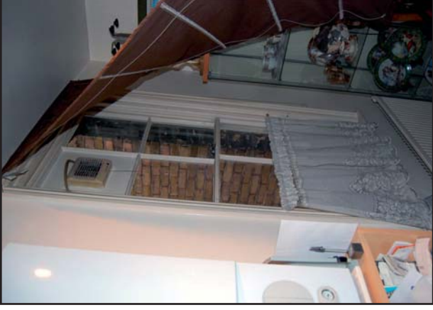
Plate 33: Potential location of former window opening prior to extension (Jan 09)
