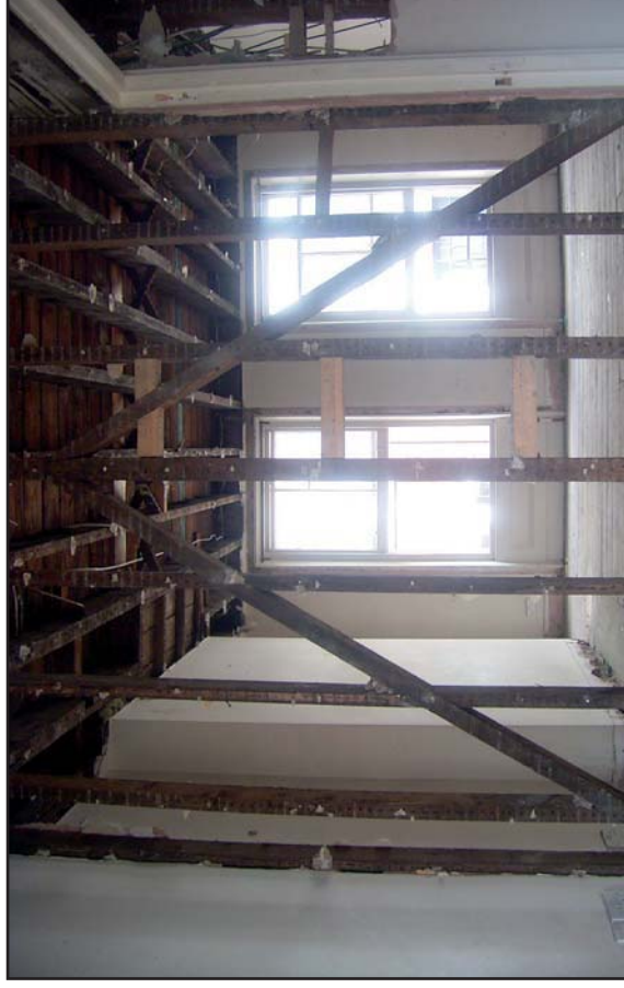
Plate 76: Partition at 2nd floor (July 2010)
