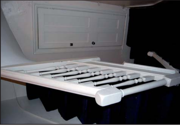
Plate 49: First floor staircase, showing newel post with its ball finial removed and handrail with raised central profile (Jan 09)
