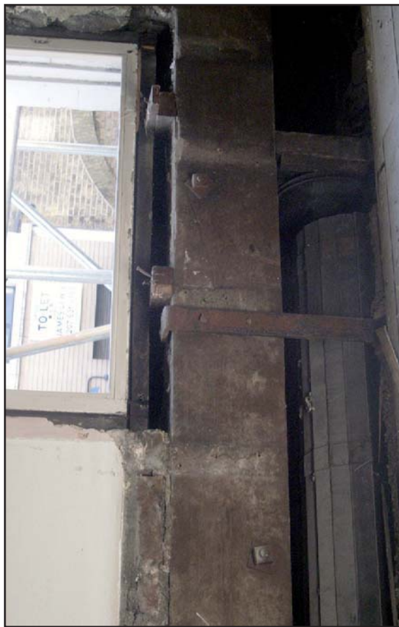
Plate 71: Detail of shop front roller shutters (July 2010)
