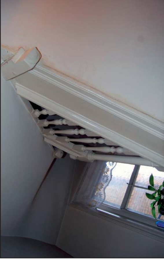
Plate 49: First floor staircase, showing newel post with its ball finial removed and handrail with raised central profile (Jan 09)
