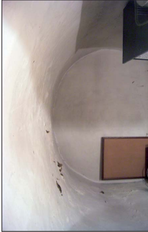
Plate 63: Vaults beneath road (July 2010)
