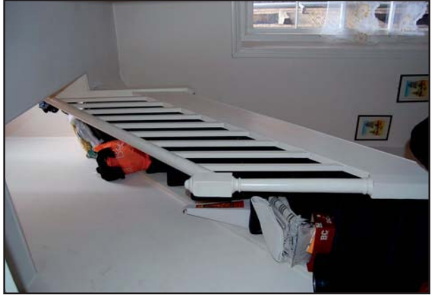
Plate 55: Non-decorative bannisters, handrail and newel post leading to roof, third floor (Jan 09)
