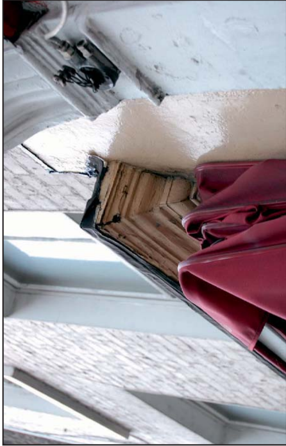
Plate 3: Stone shopfront cornice detail (Jan 09)
