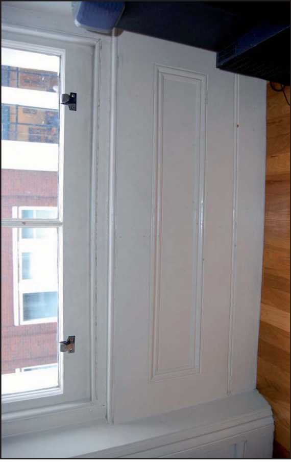
Plate 38: Recessed timber panelling below 2 x 2 sash, bedroom No. 1 second floor (Jan 09)
