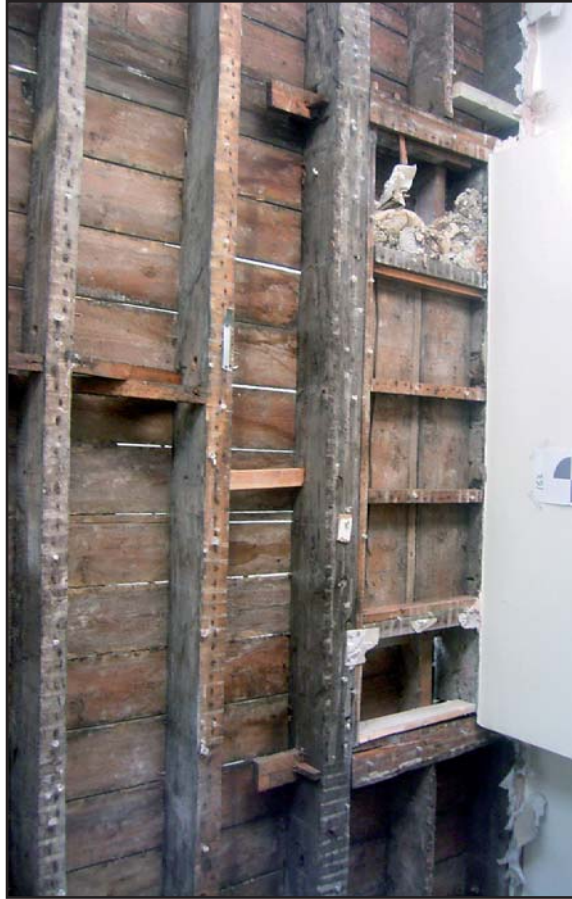
Plate 72: Underside of 2nd floor hearth detail (July 2010)
