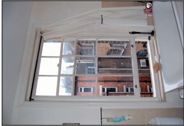
Plate 47: 3 x 6 timber sash, bathroom, third floor (Jan 09)
