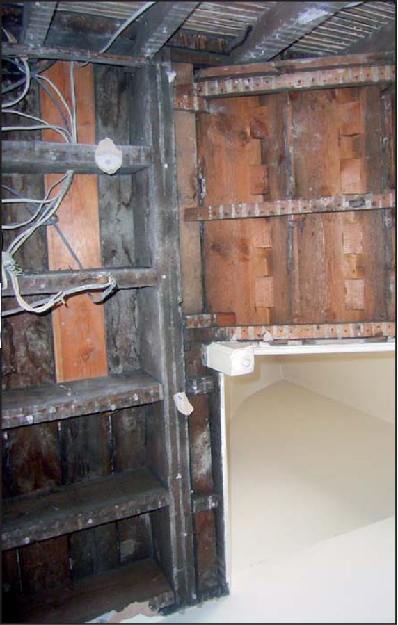
Plate 82: Staircase detail during soft strip (July 2010)
