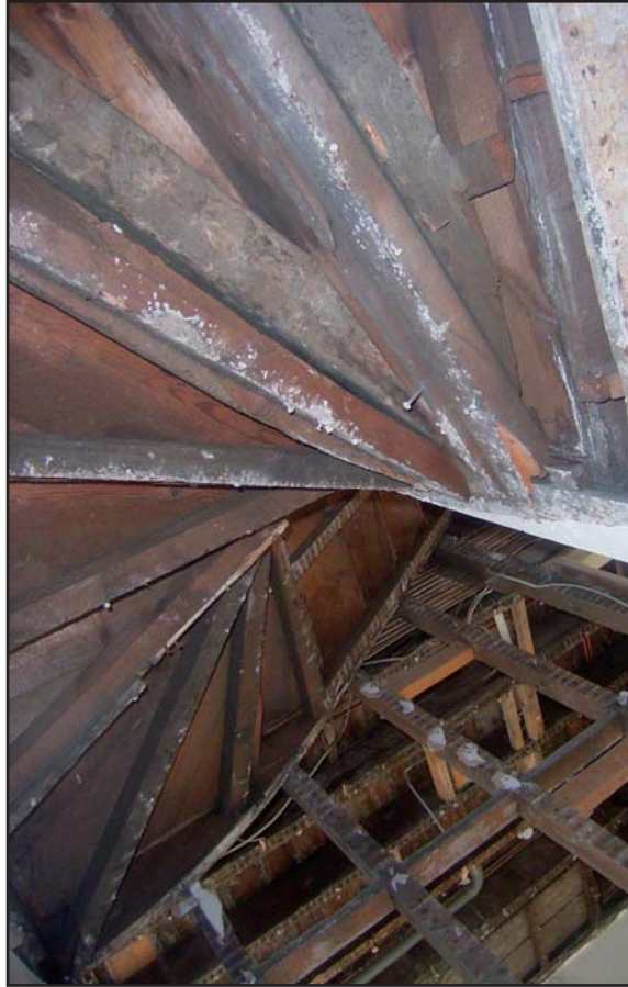
Plate 84: Staircase detail during soft strip (July 2010)
