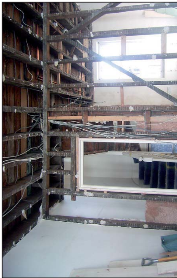
Plate 79: Partition at 2nd floor after soft strip (July 2010)
