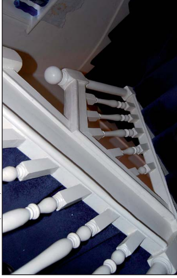
Plate 51: Staircase leading to second floor showing decorative newel with ball finial, bannisters and handrail with only slightly raised profile (Jan 09)
