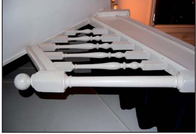
Plate 51: Staircase leading to second floor showing decorative newel with ball finial, bannisters and handrail with only slightly raised profile (Jan 09)
