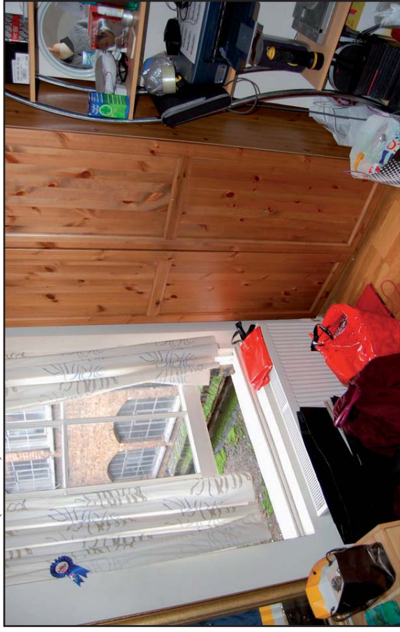
Plate 38: Recessed timber panelling below 2 x 2 sash, bedroom No. 1 second floor (Jan 09)
