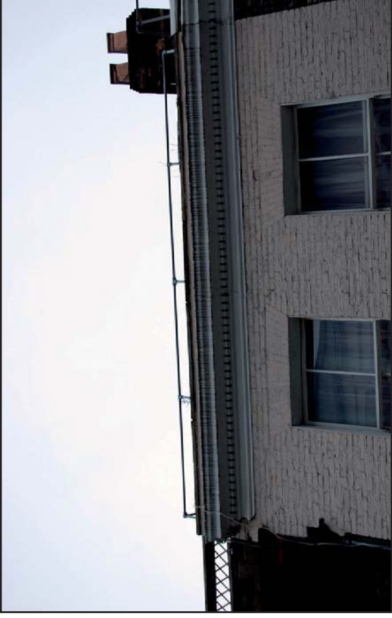
Plate 2: Cornice with dentillation detail & masonry cut by rainwater goods (Jan 09)
