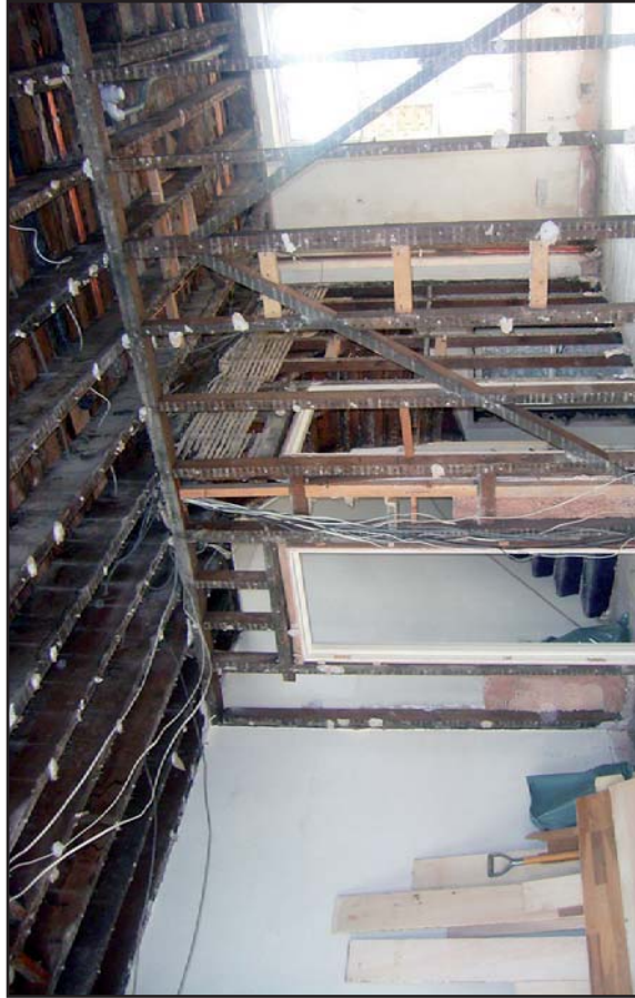
Plate 80: Partition at 2nd floor after soft strip (July 2010)
