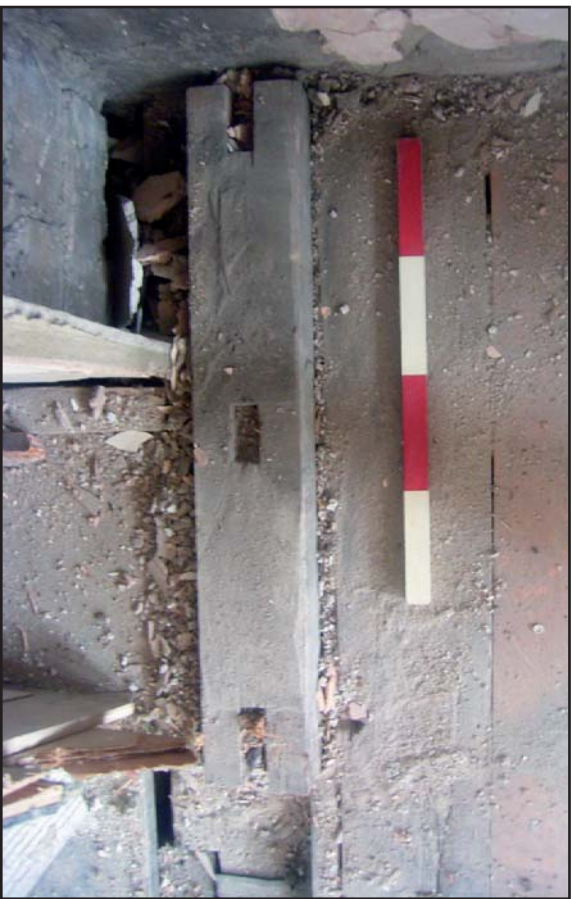
Plate 69: Mortices from removed partition at 1st floor (July 2010)
