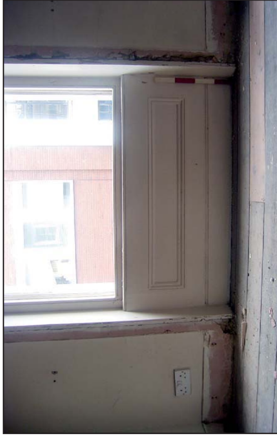
Plate 75: Panelling beneath window at 2nd floor (July 2010)
