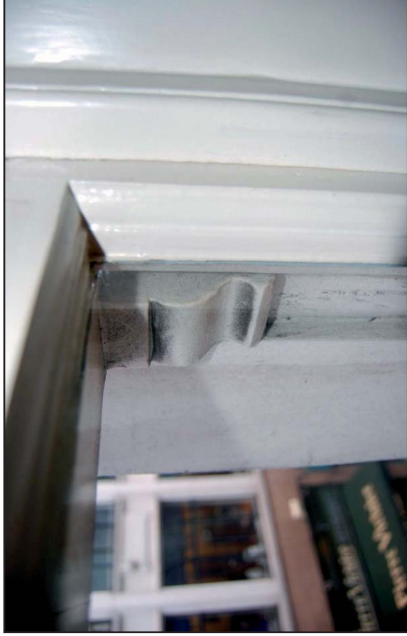
Plate 39: Horn detailing on 2 x 2 sash, bedroom No. 1, second floor. (Jan 09)
