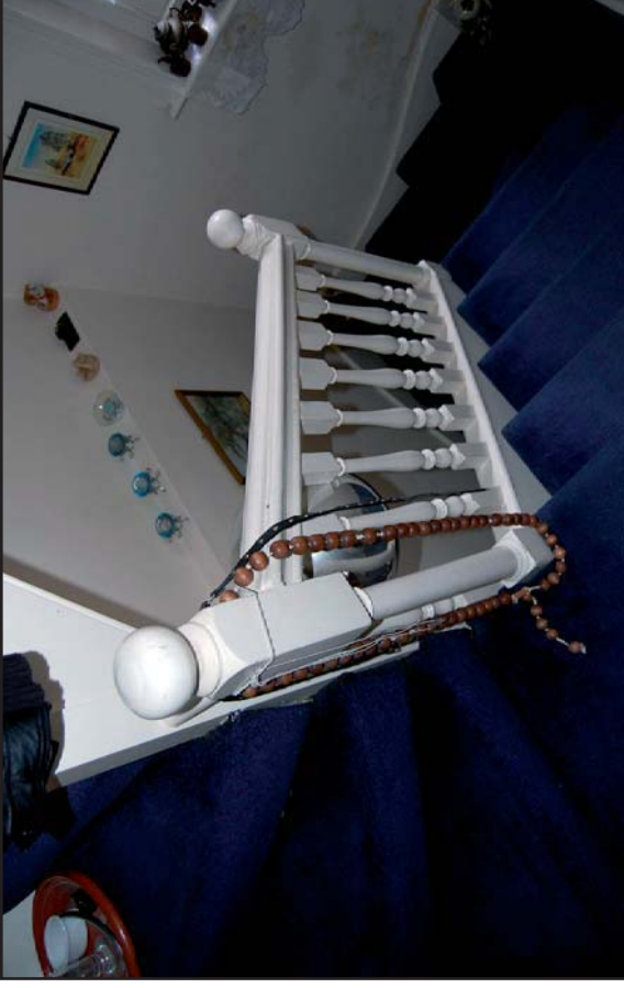
Plate 54: Staircase with newel post featuring ball finials and handrail with raised profile, third floor (Jan 09)
