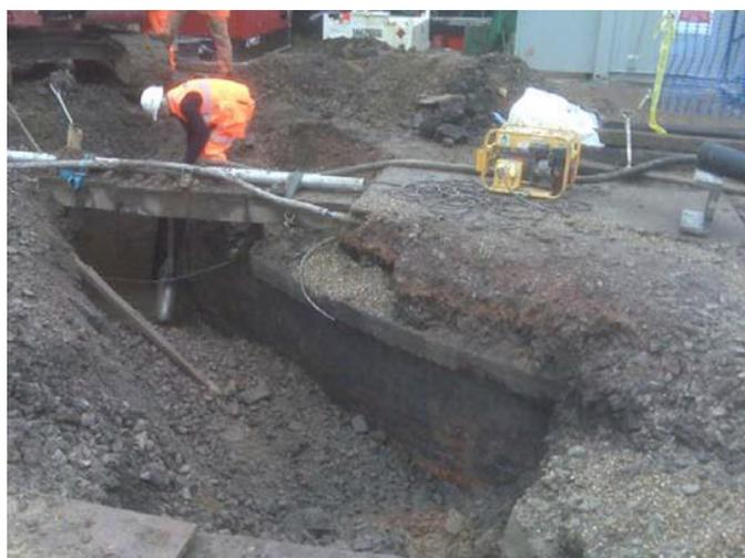
**Figure 4: Part of the 1882 turntable (Structure 14) exposed during utility works**
