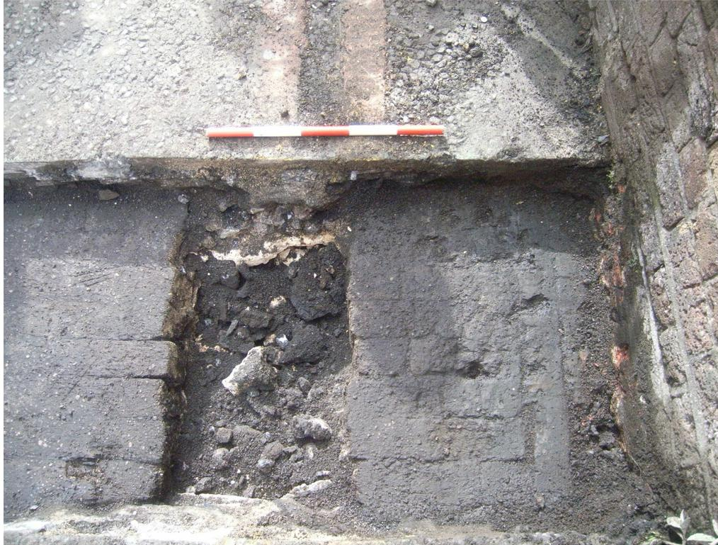
Plate 2: Detail showing setts set length ways against Eastbourne Terrace Wall Utilities Trench 2 (not illustrated)
