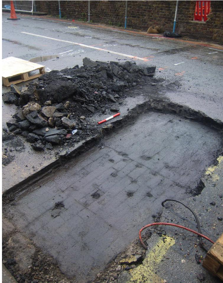
Plate 3: Detail showing re-laying 'seam' in joint construction TPSW3
