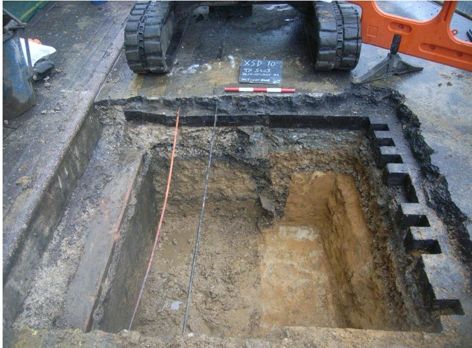
Plate 4: Section showing variation in cement base coinciding with basement construction cut and seam in roadway. TPSW3
