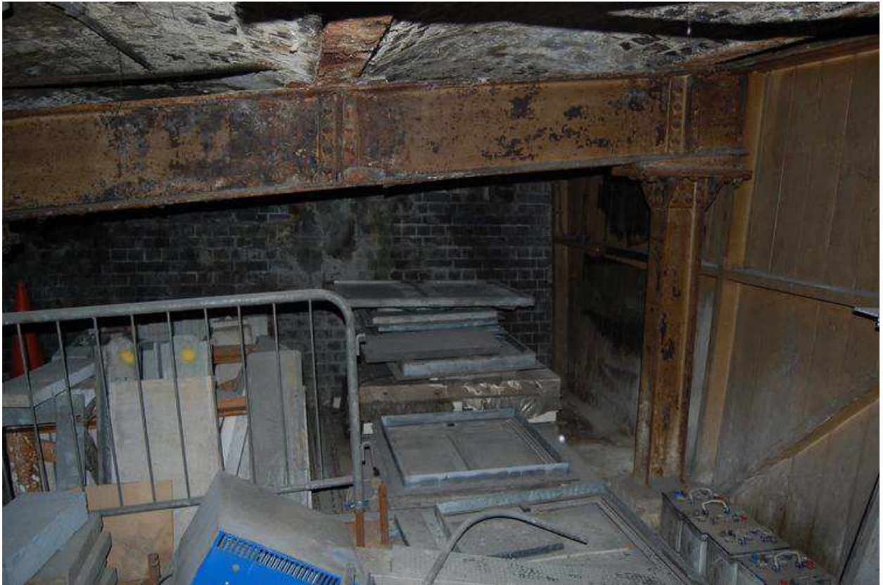
Plate 50: View of office below ramp – south end
