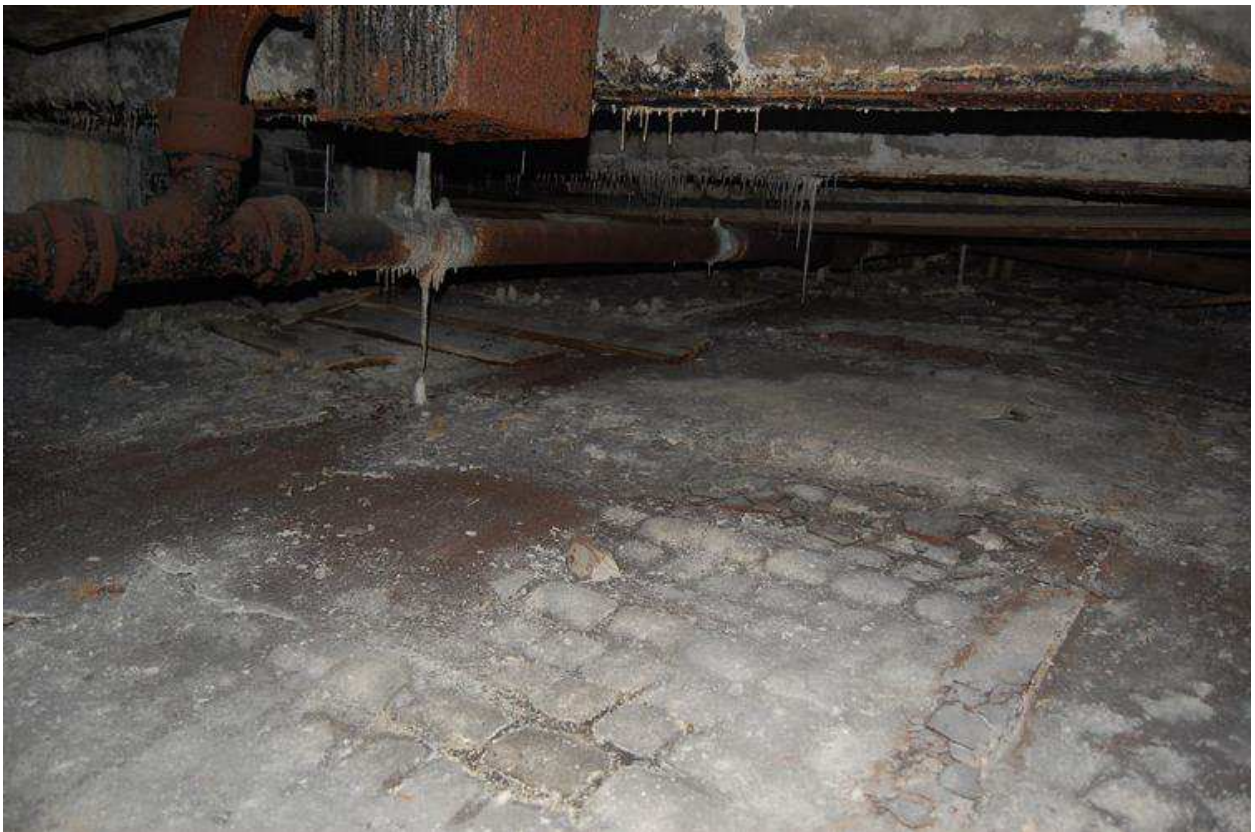
Plate 5: View of southern end of ramp
