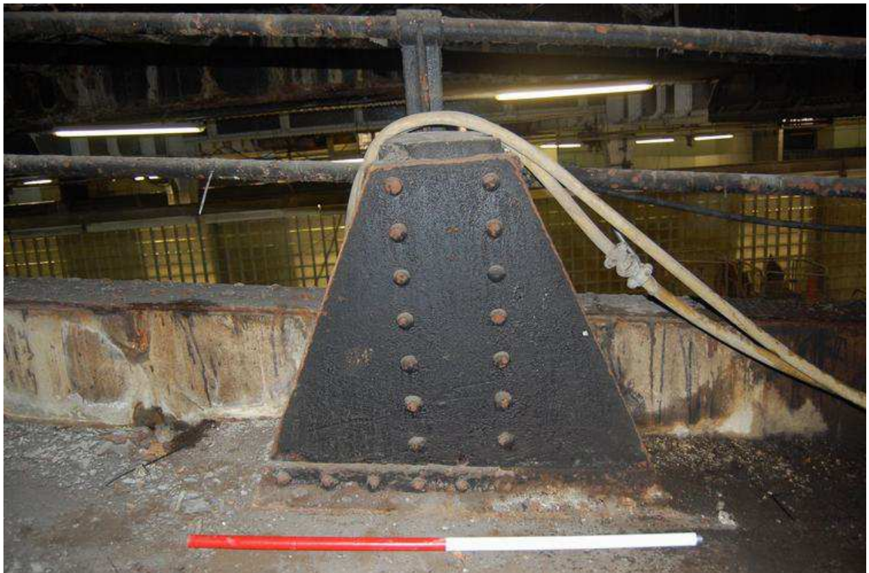
Plate 11: west elevation of inverted stanchion on ramp
