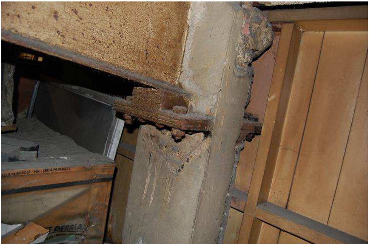
Plate 61: southern stanchion within office space, encased in concrete
