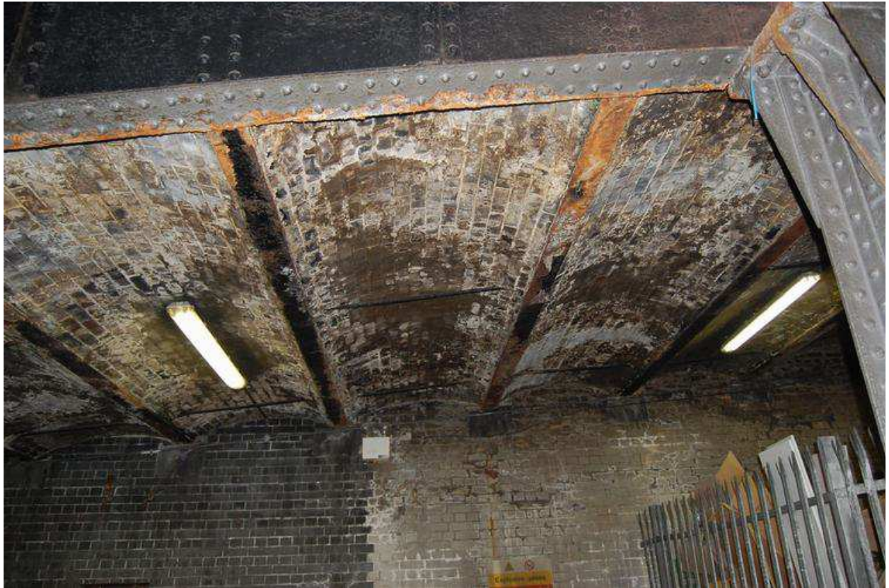
Plate 48: View of retaining wall below ramp – south end
