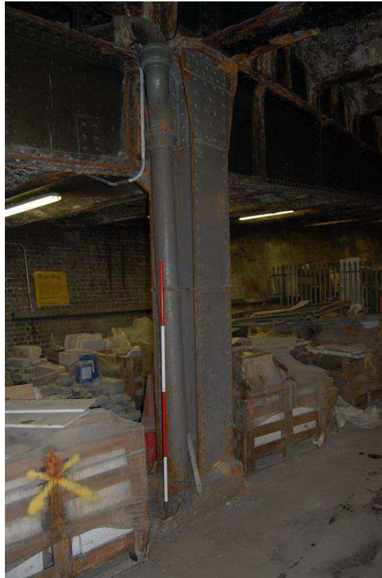
Plate 34: S5 south and east elevations
