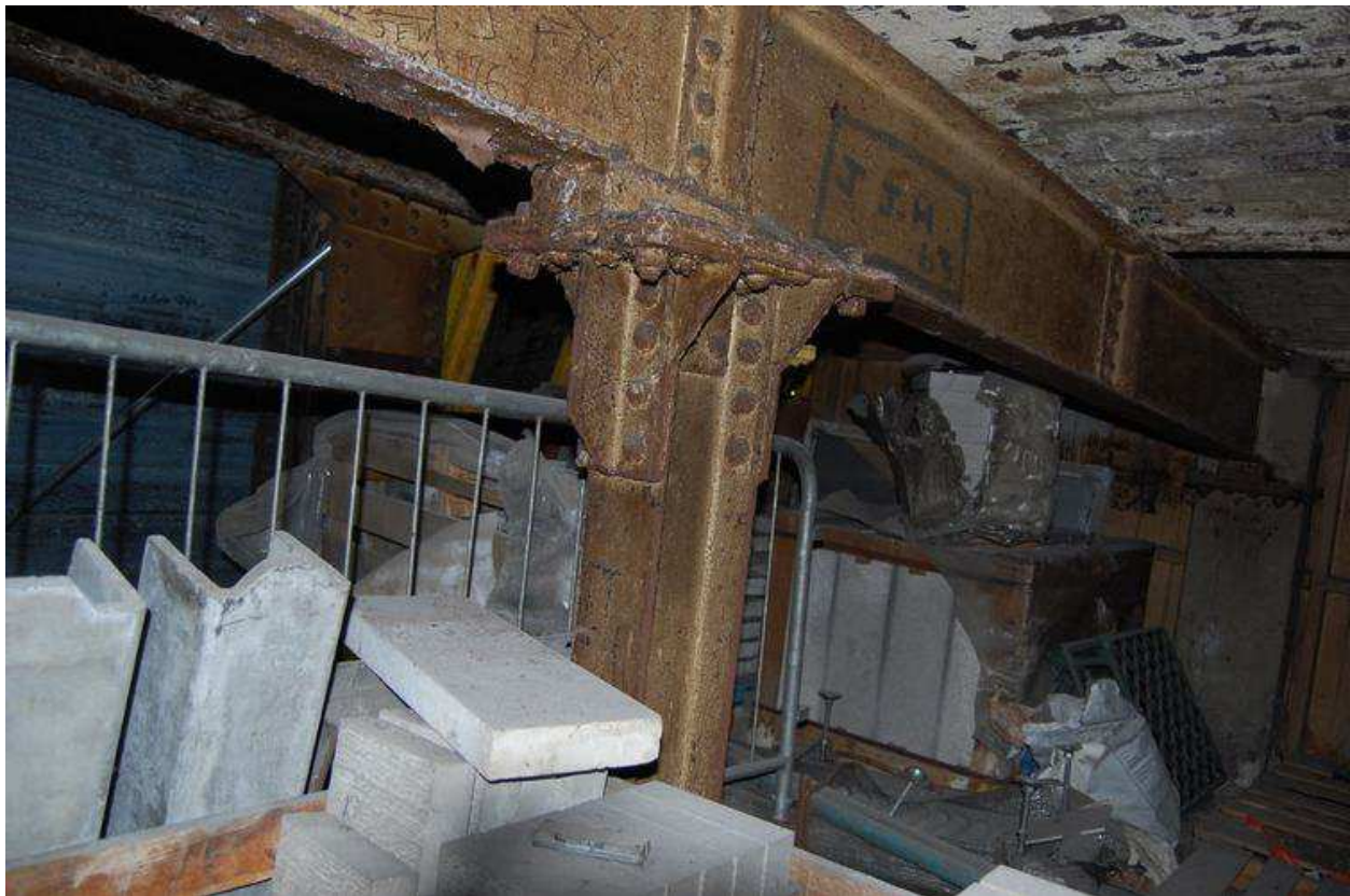
Plate 57: Central stanchion within office space – west elevation
