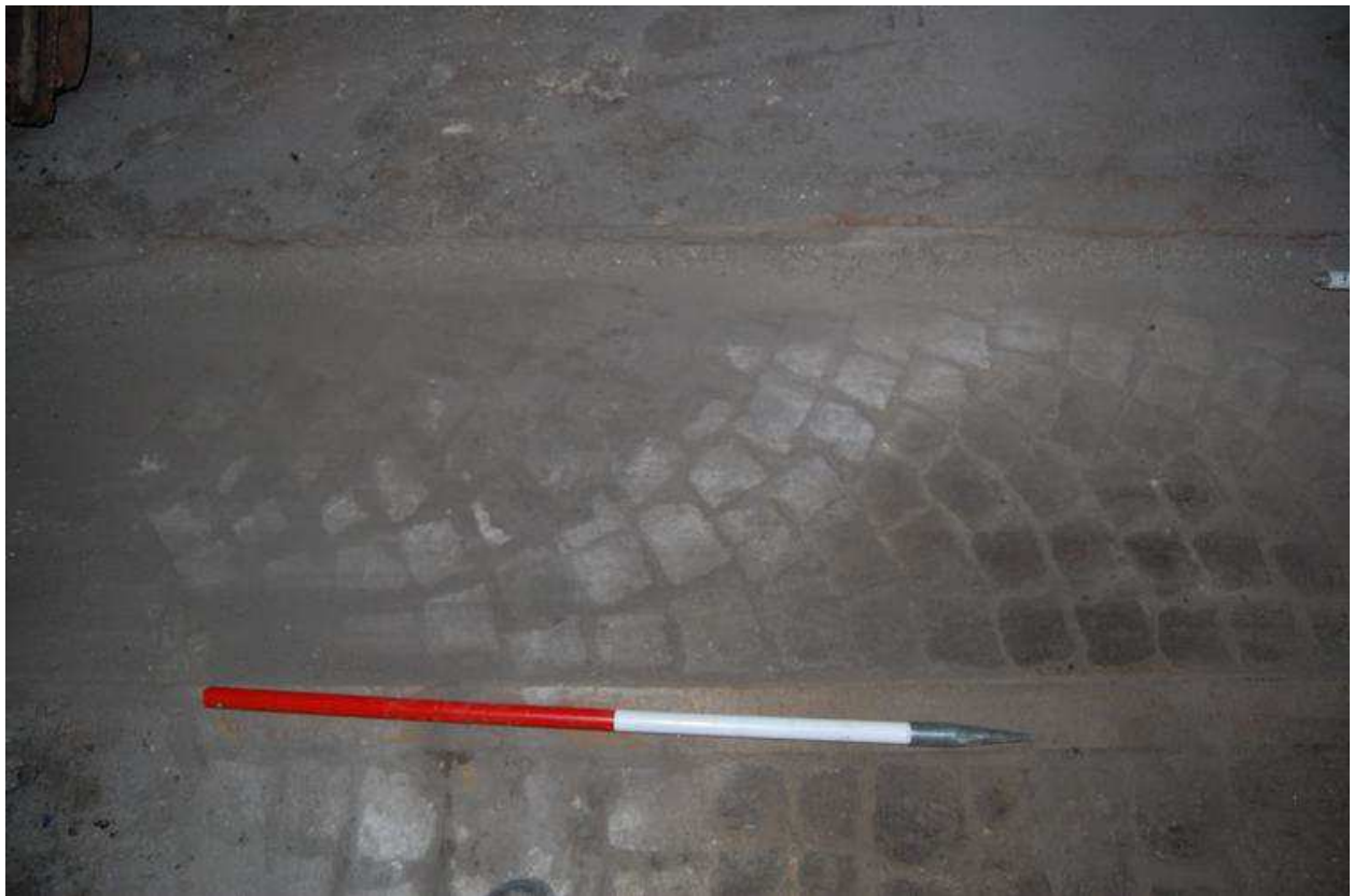
Plate 21: Detail of sett surface - edge
