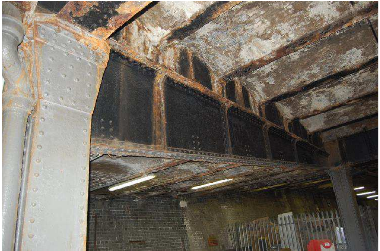
Plate 72: East elevation of ramp between S4 and S5
