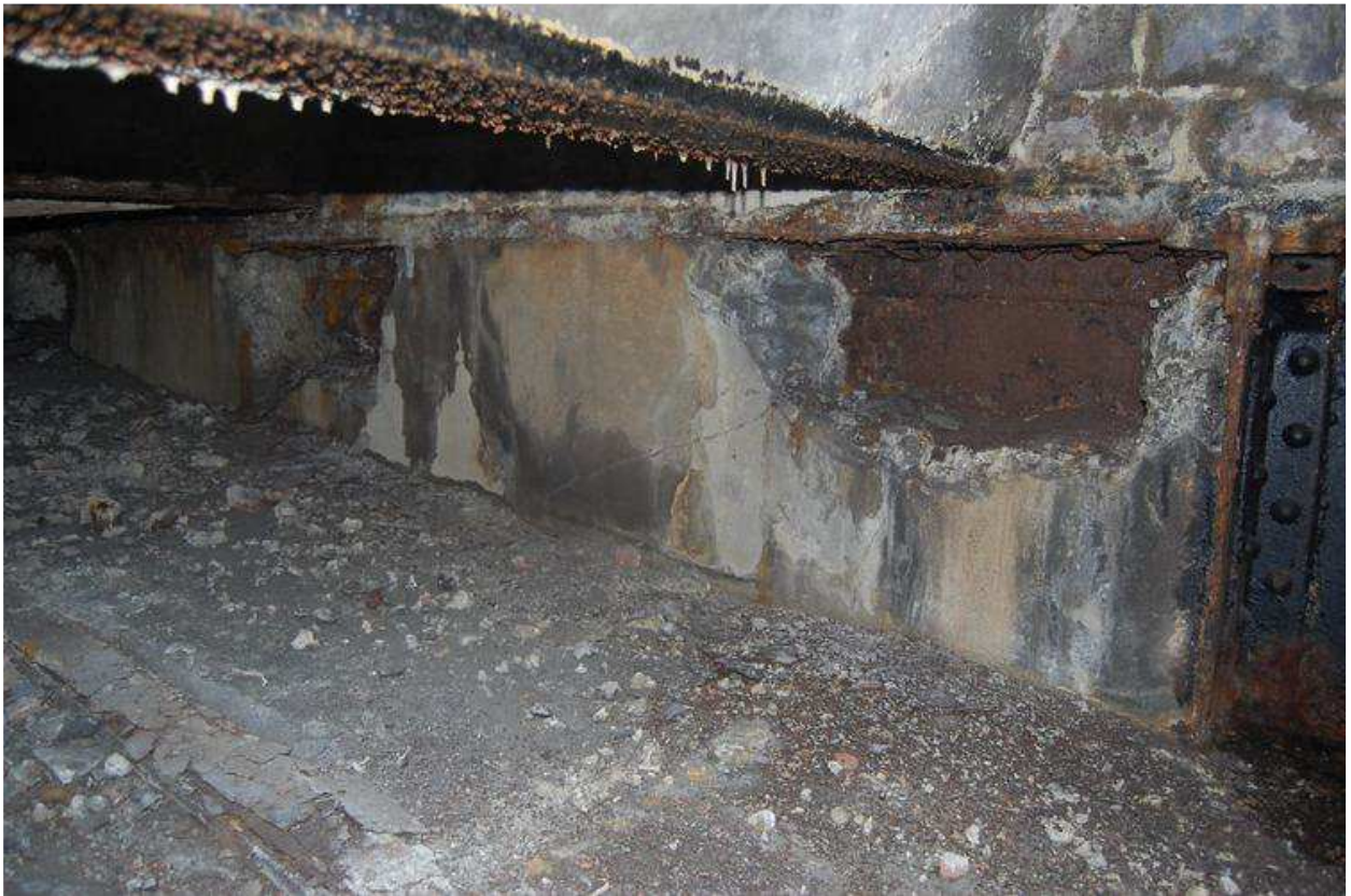
Plate 7: Detail of concrete infill to G3 west elevation
