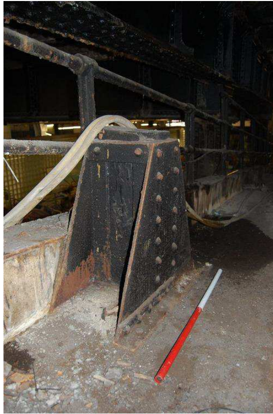
Plate 12: South and west elevations of inverted stanchion on ramp
