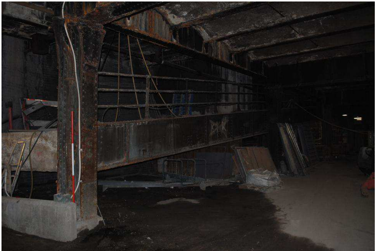
Plate 73: East elevation of ramp between S6 and S7
