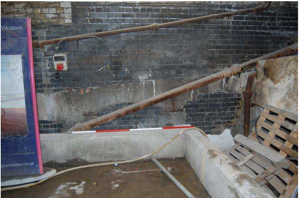
Plate 65: Detail of scar for continuation of ramp
