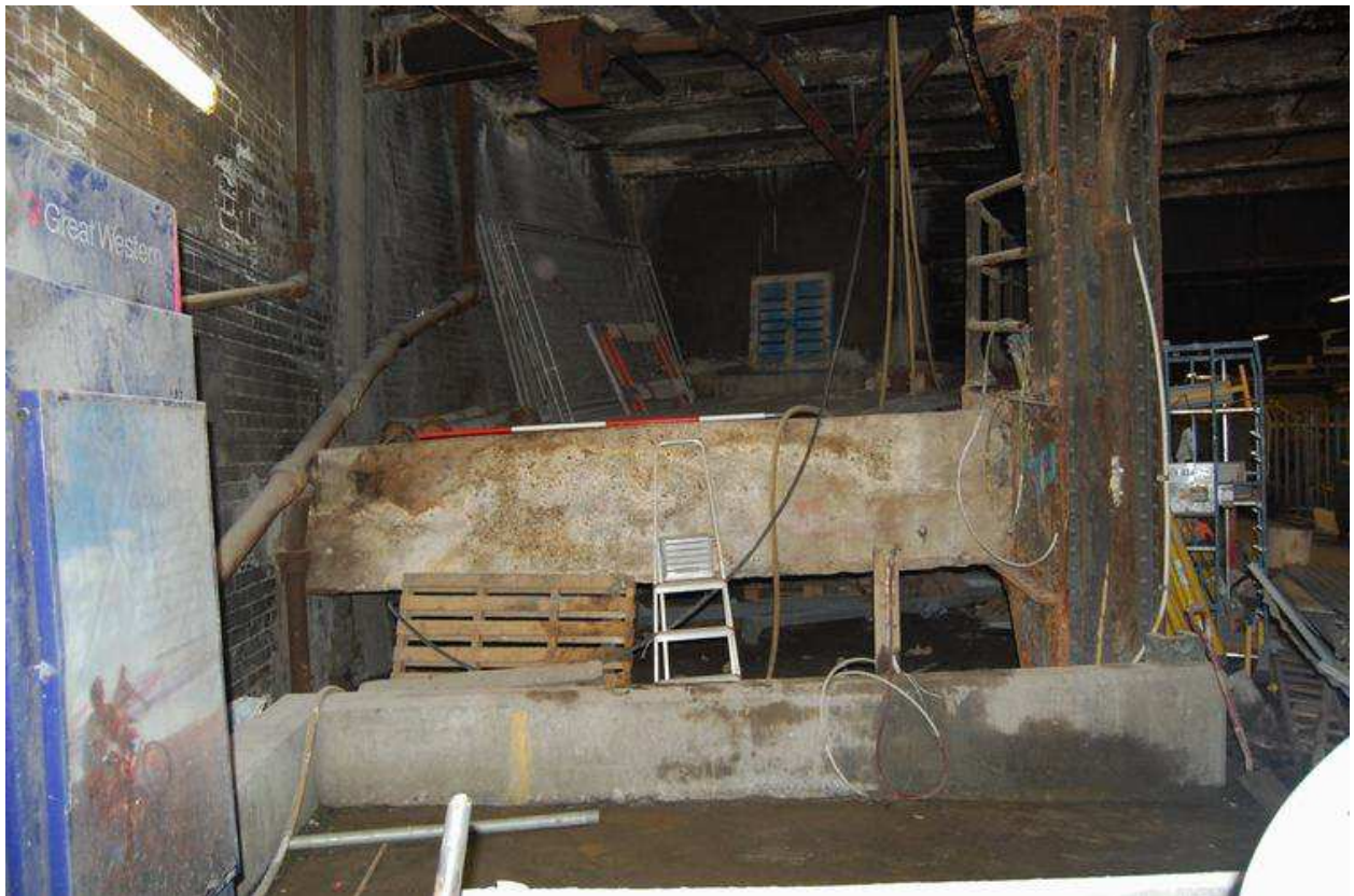
Plate 69: Detail of truncated end of ramp
