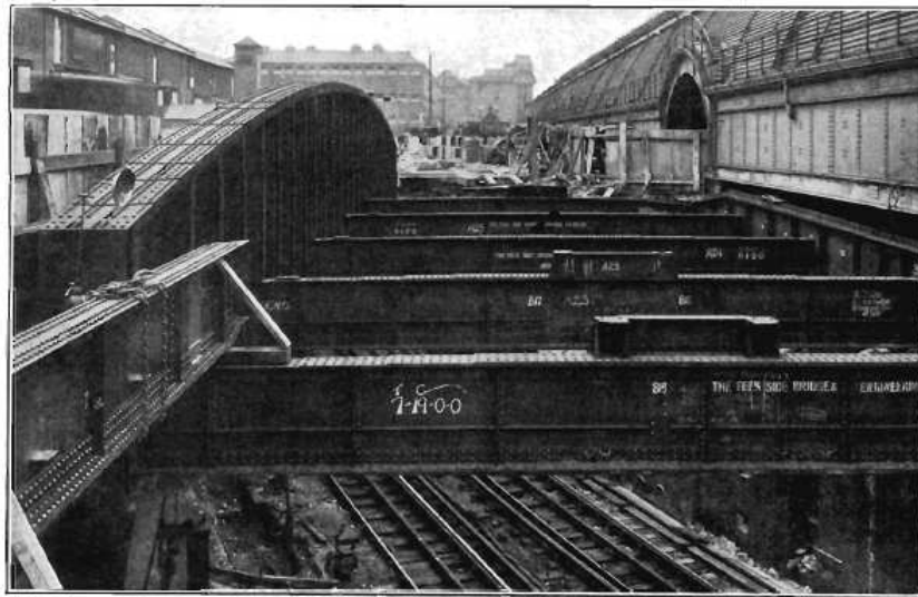
Plate H: Photo of showing bow string girder over the Bishops Road tunnel at the west end of the London Street Deck
