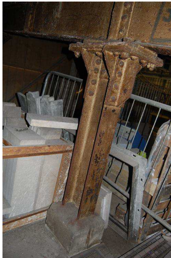
Plate 59: Central stanchion within office space
