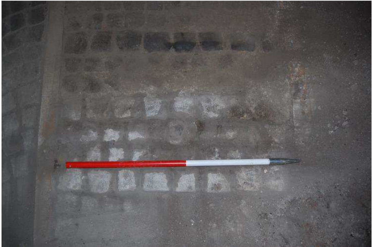
Plate 20: Detail of ramp sett surface – centre
