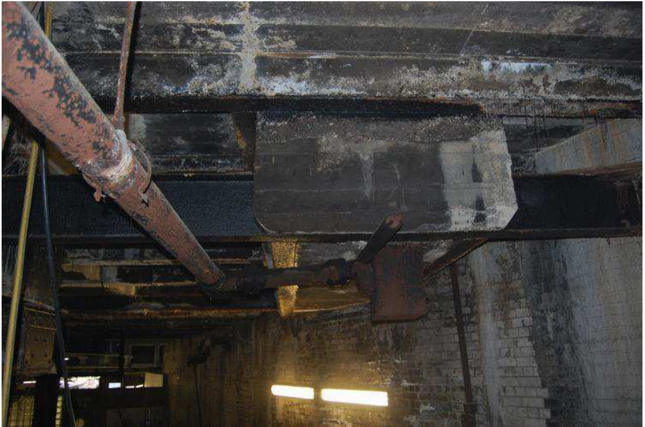
Plate 24: Detail of inserted inspection pit – south end
