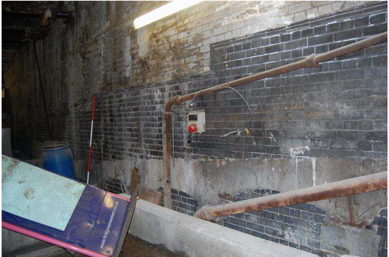
Plate 68: Detail of scar for continuation of ramp
