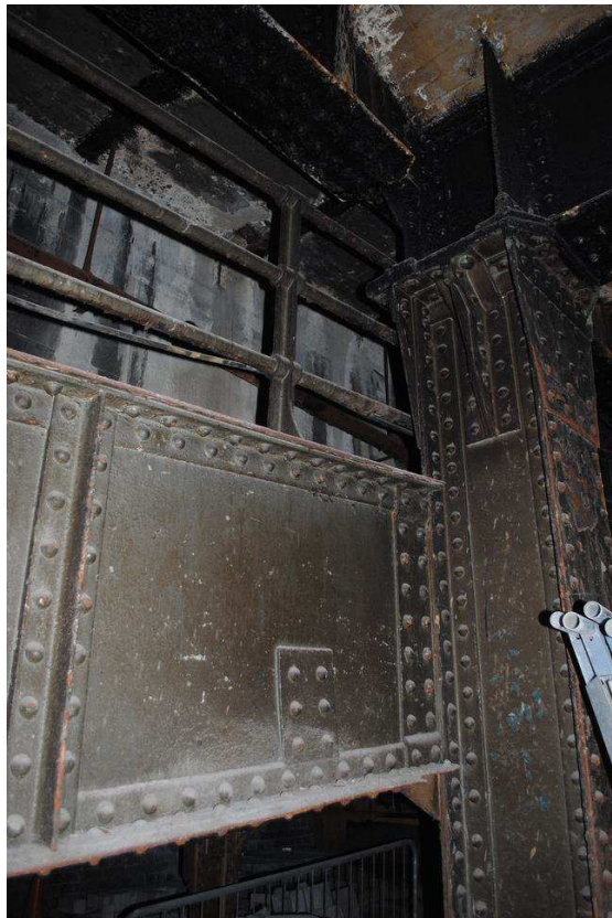
Plate 77: Detail of junction between G4 and S6
