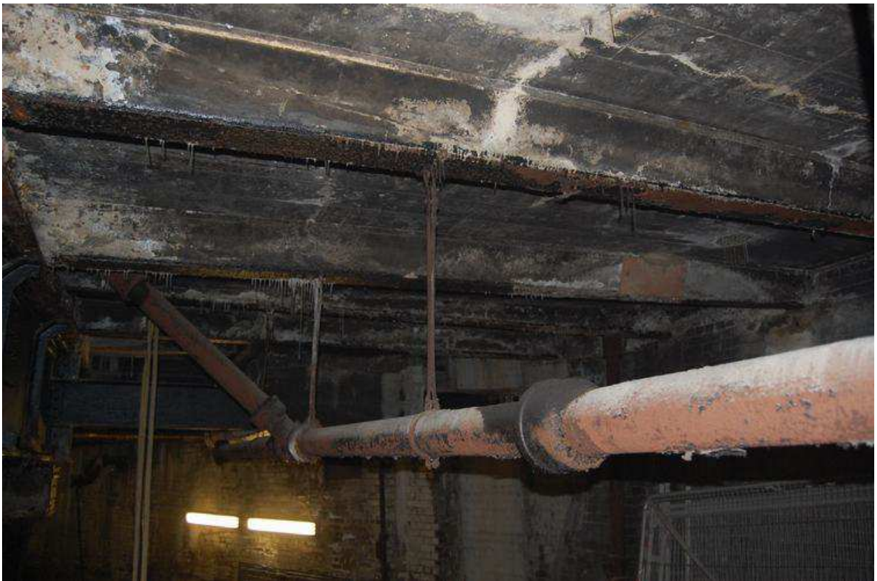
Plate 25: detail of concrete reinforcement of jack arches over ramp
