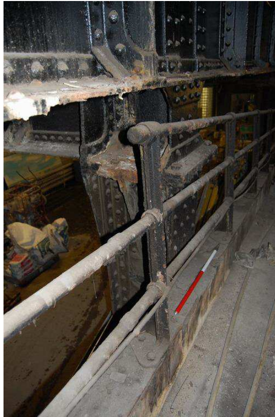
Plate 14: South view of stanchion S6 capital
