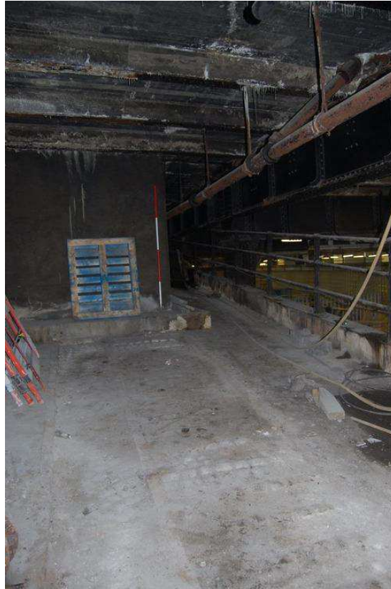
Plate 1: View south along ramp – north end
