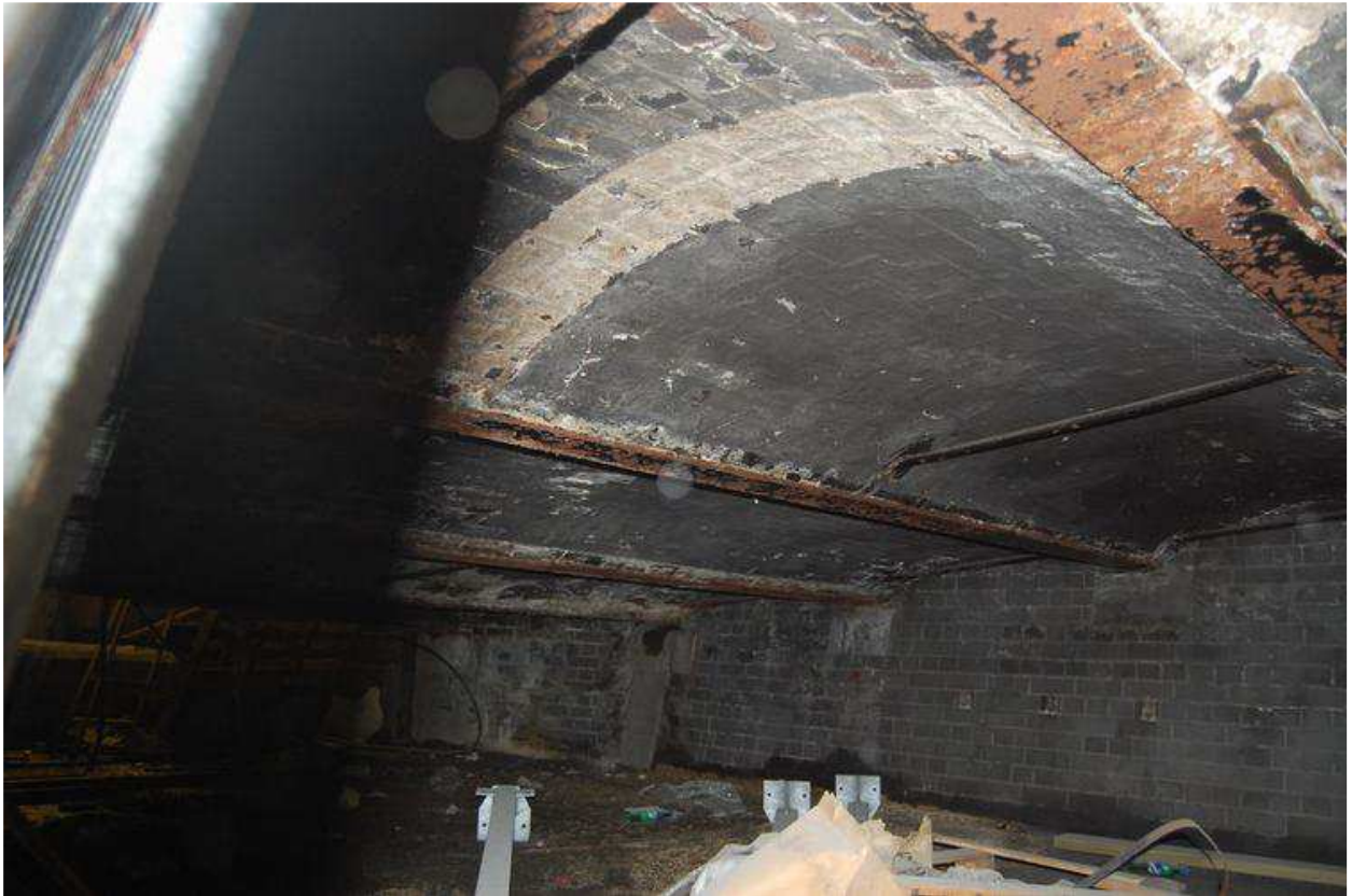
Plate 64: View below ramp – south end
