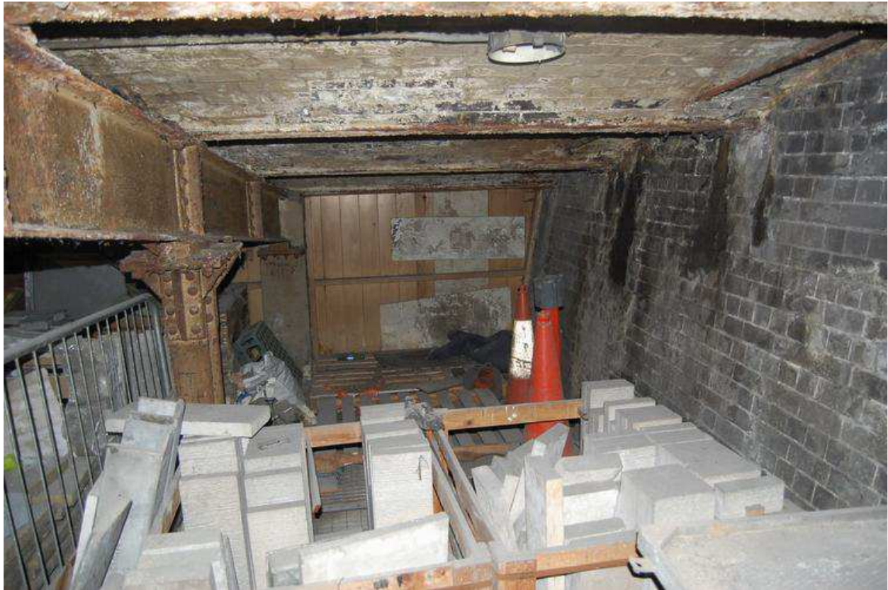
Plate 56: View south within office space
