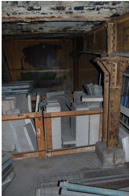
Plate 62: View south inside office space
