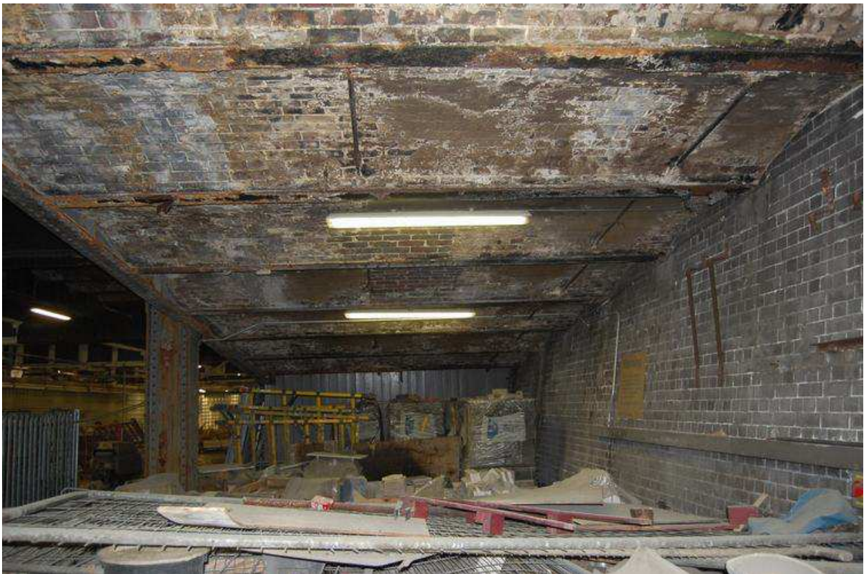
Plate 45: View south under ramp – south end
