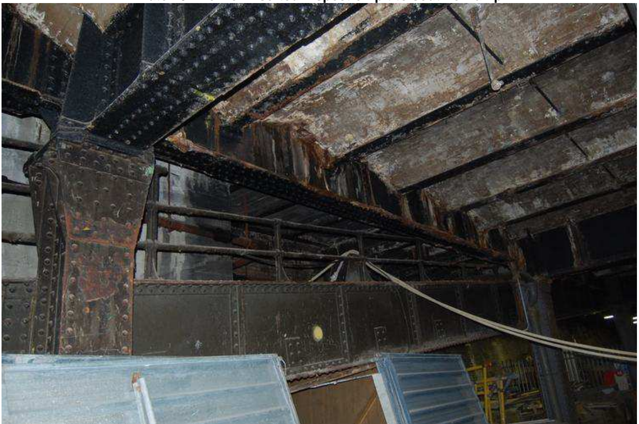
Plate 71: East elevation of ramp between S5 and S6
