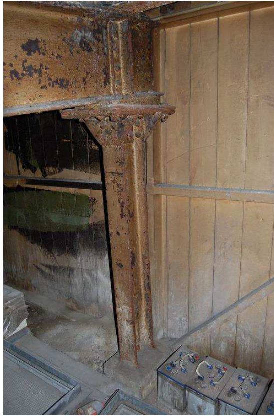
Plate 52: Stanchion at south end of office space
