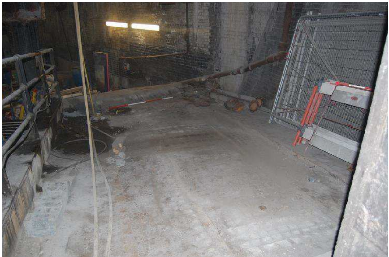
Plate 27: View south along ramp – south end
