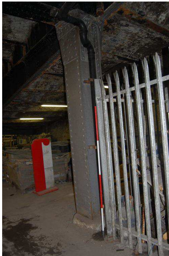
Plate 41: S4 south and east elevations
