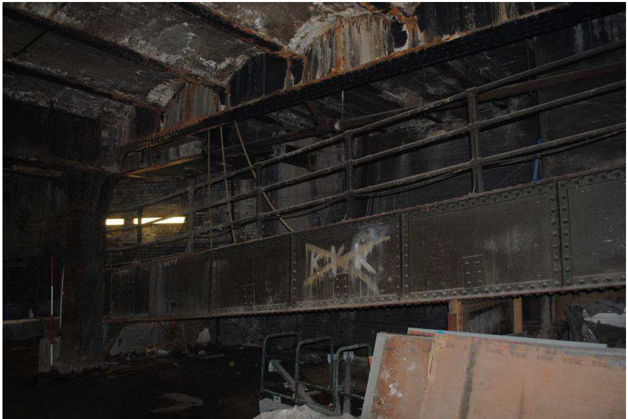
Plate 78: East elevation of G4 between S6 and S7
