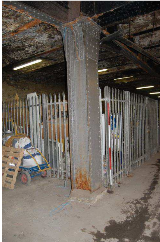
Plate 40: S4 south and east elevations
