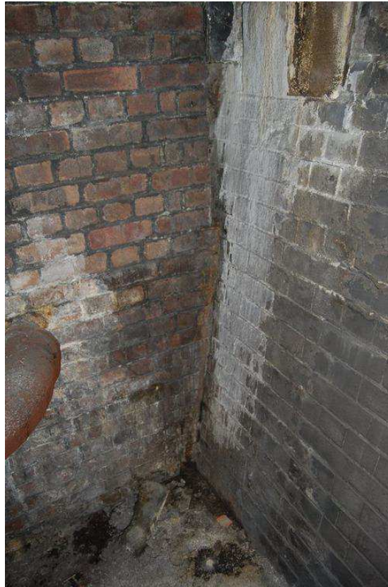
Plate 10: Junction between retaining wall and petrol inceptor
