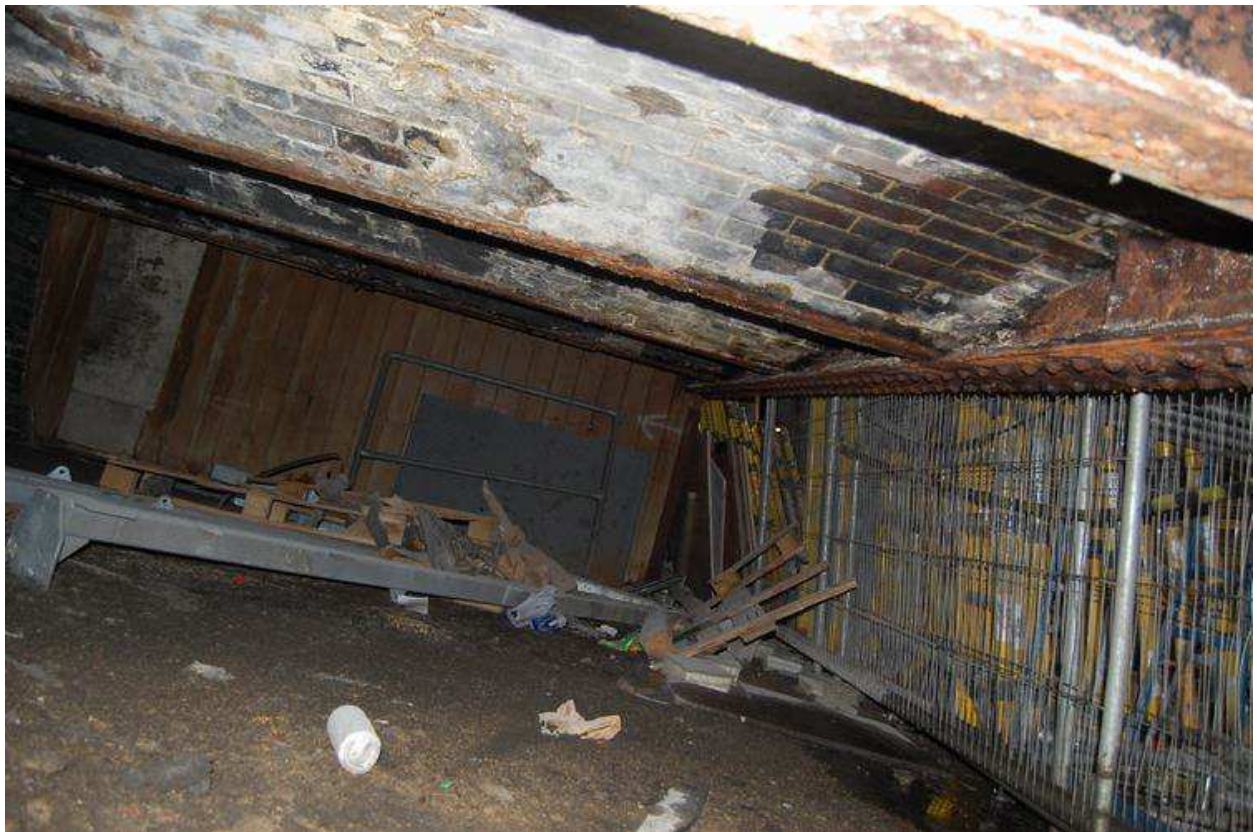
Plate 67: View below ramp towards the south
