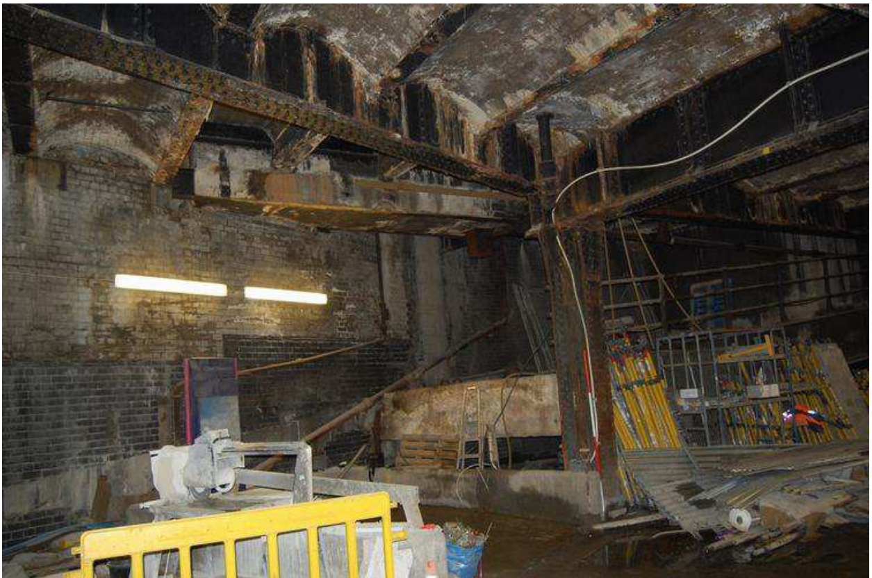
Plate 33: General view of ramp showing truncation
