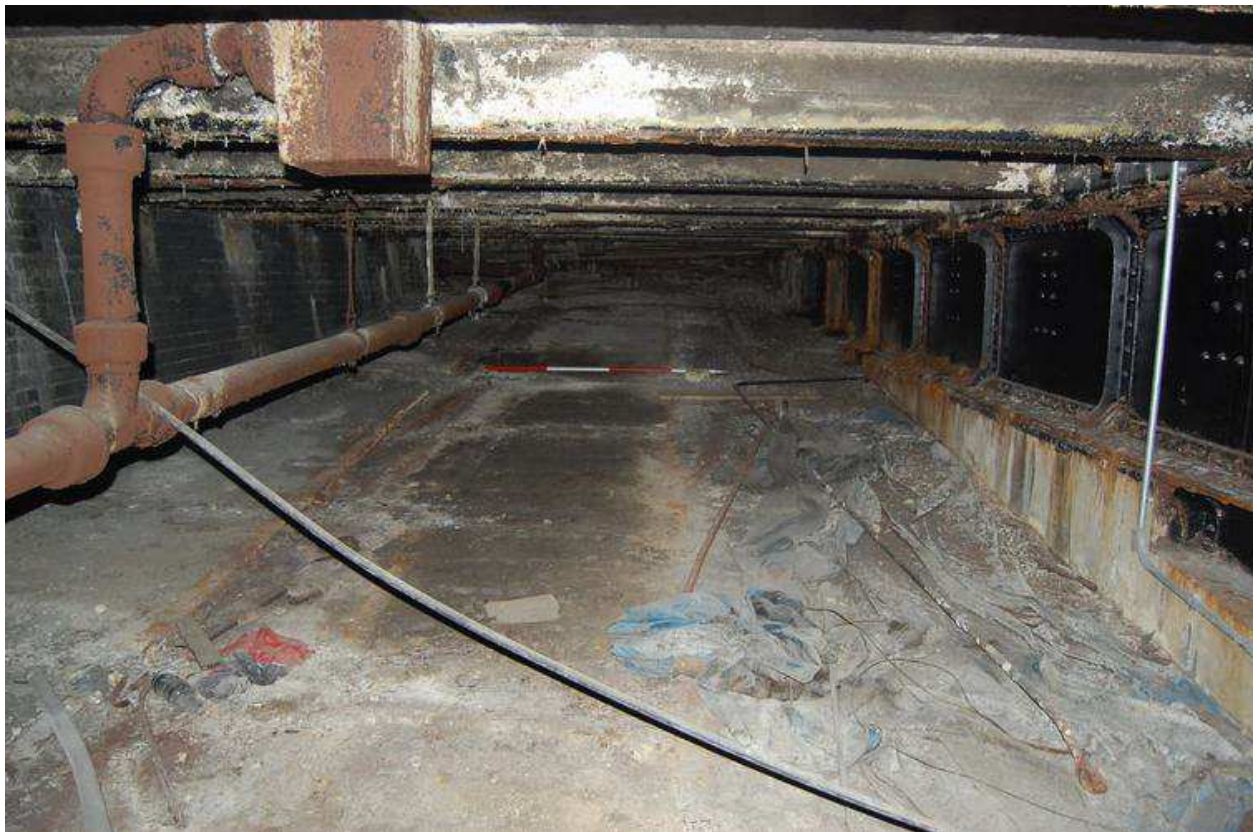
Plate 3: View south along ramp –south end
