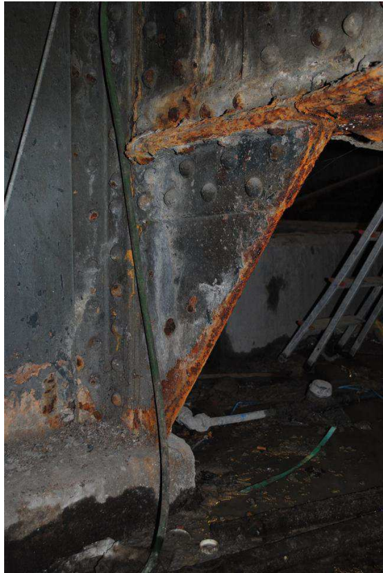
Plate 74: Detail of junction between G4 and S7
