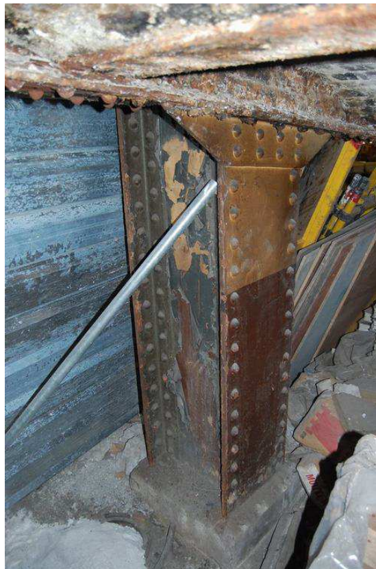
Plate 51: S6 west elevation within office space
