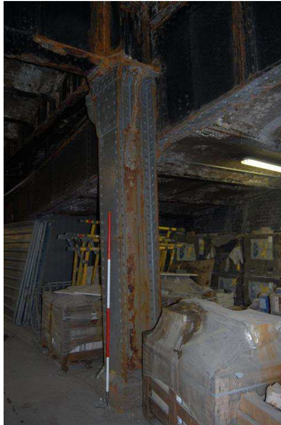
Plate 36: S5 south and east elevations
