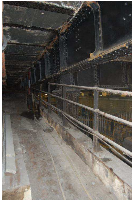
Plate 2: View south showing west elevation of railings
