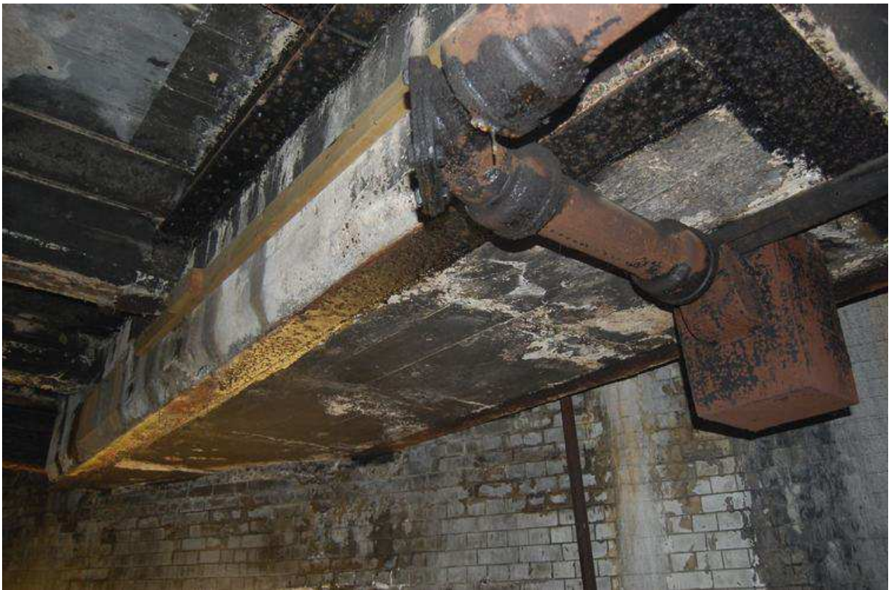
Plate 23: Detail of inserted inspection pit
