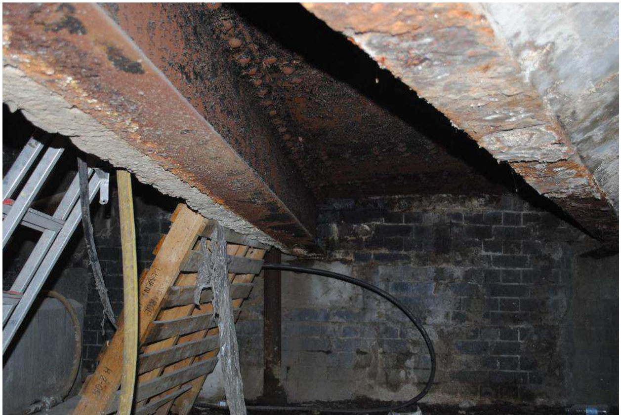
Plate 75: Underside of ramp showing change in angle
