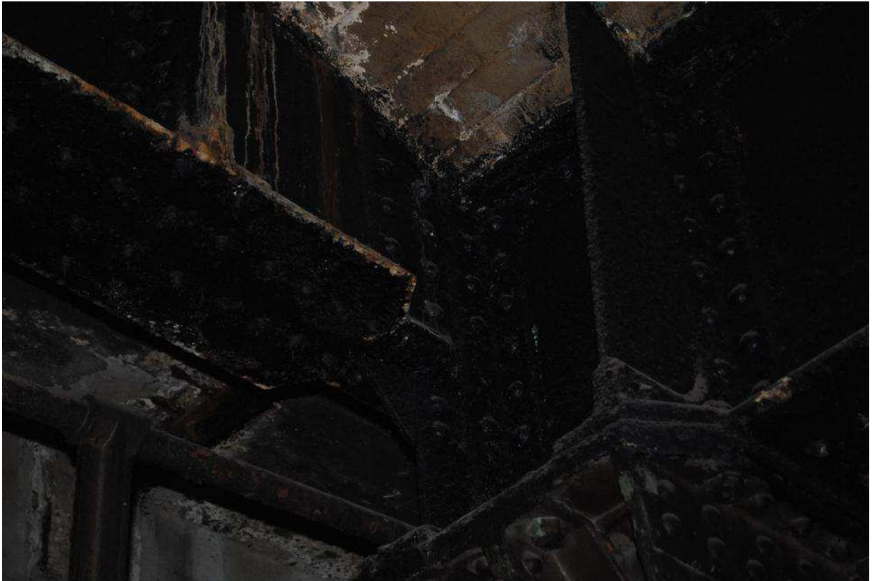
Plate 6: Detail of junction between G4 and S6
