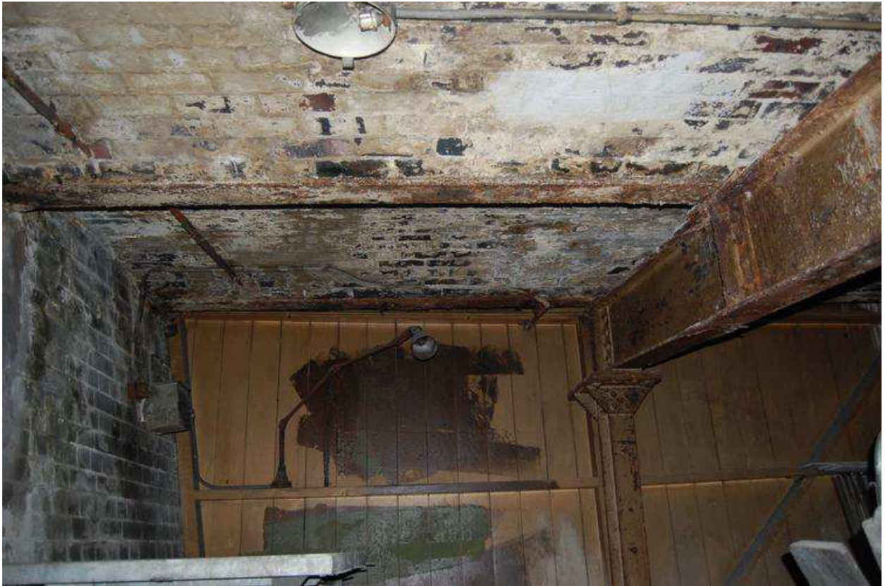
Plate 60: Southern elevation of office
