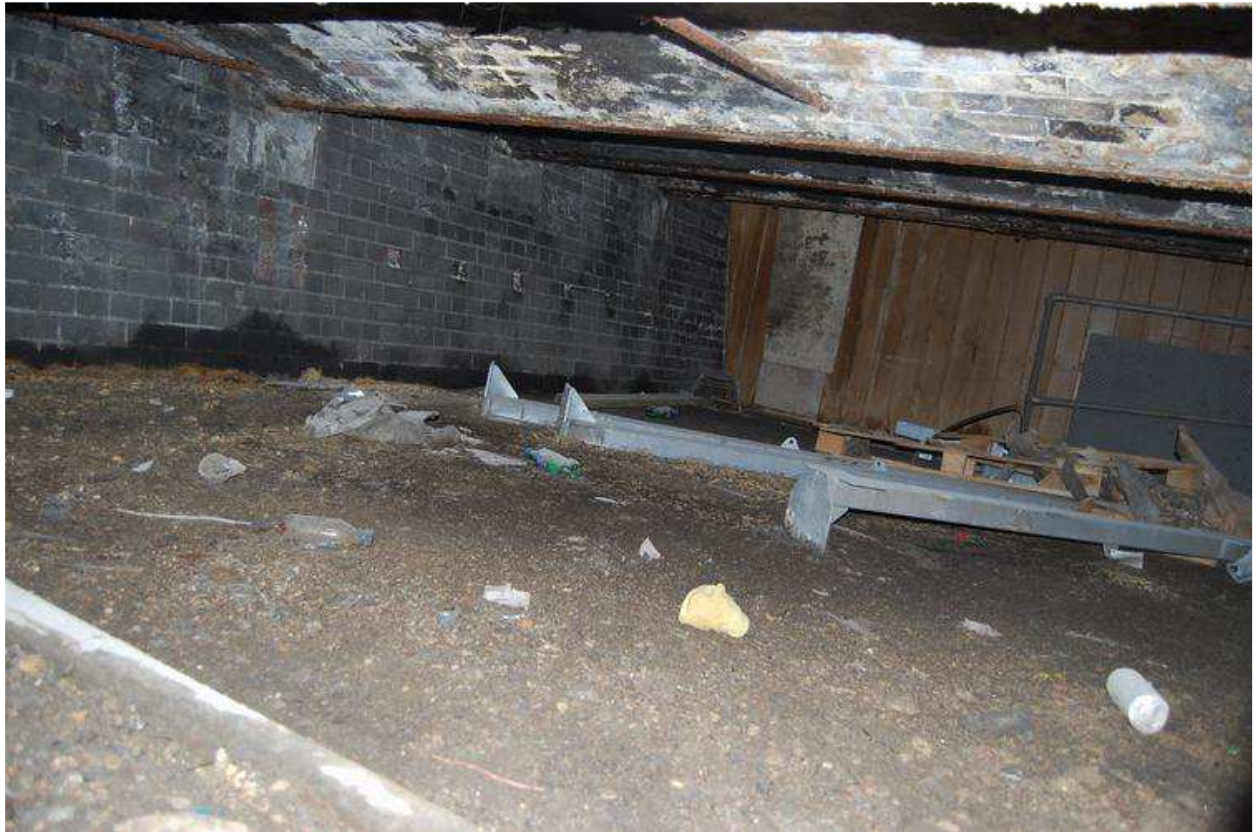
Plate 66: View below ramp towards the south
