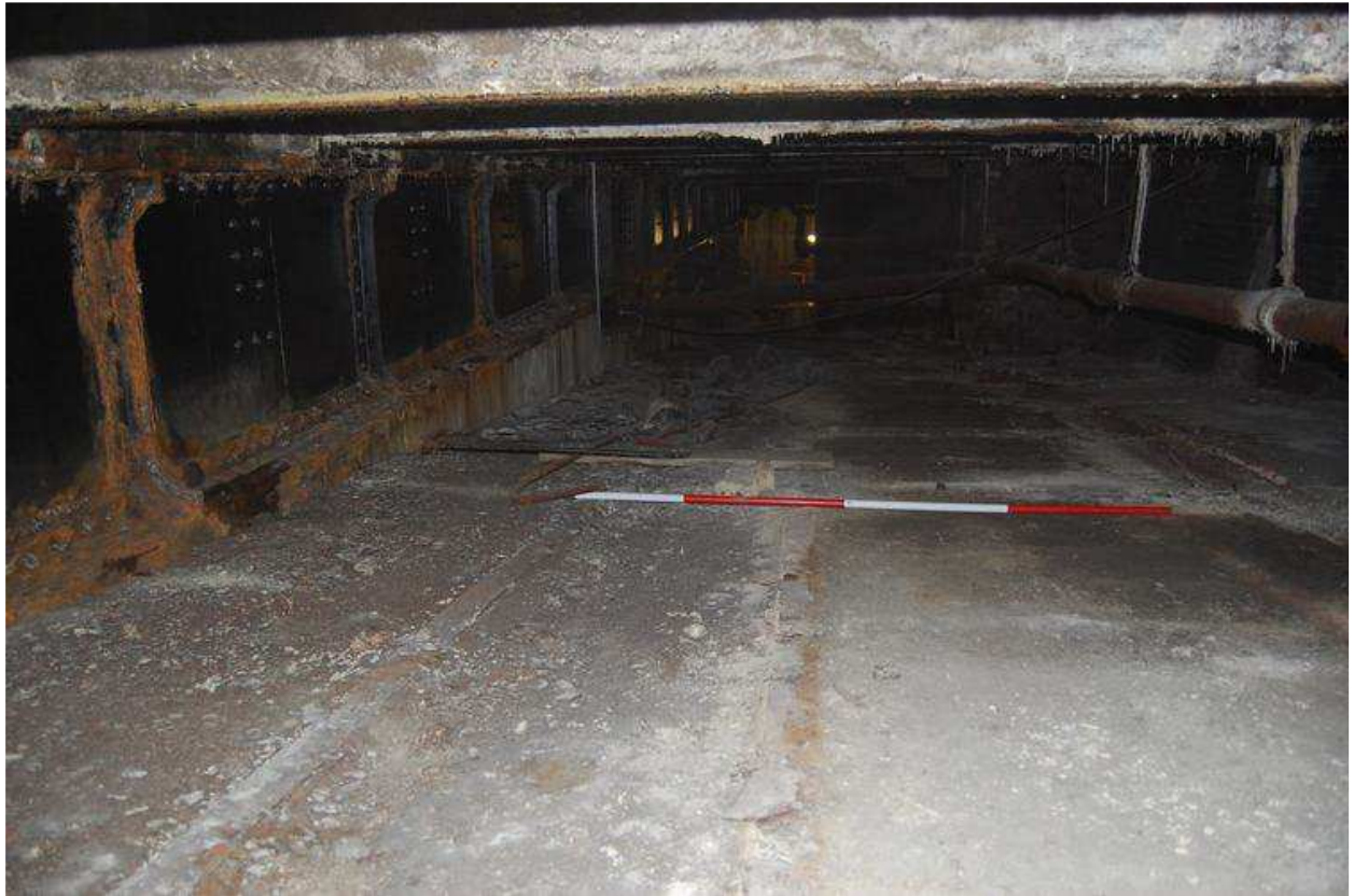
Plate 8: View south along ramp – south end
