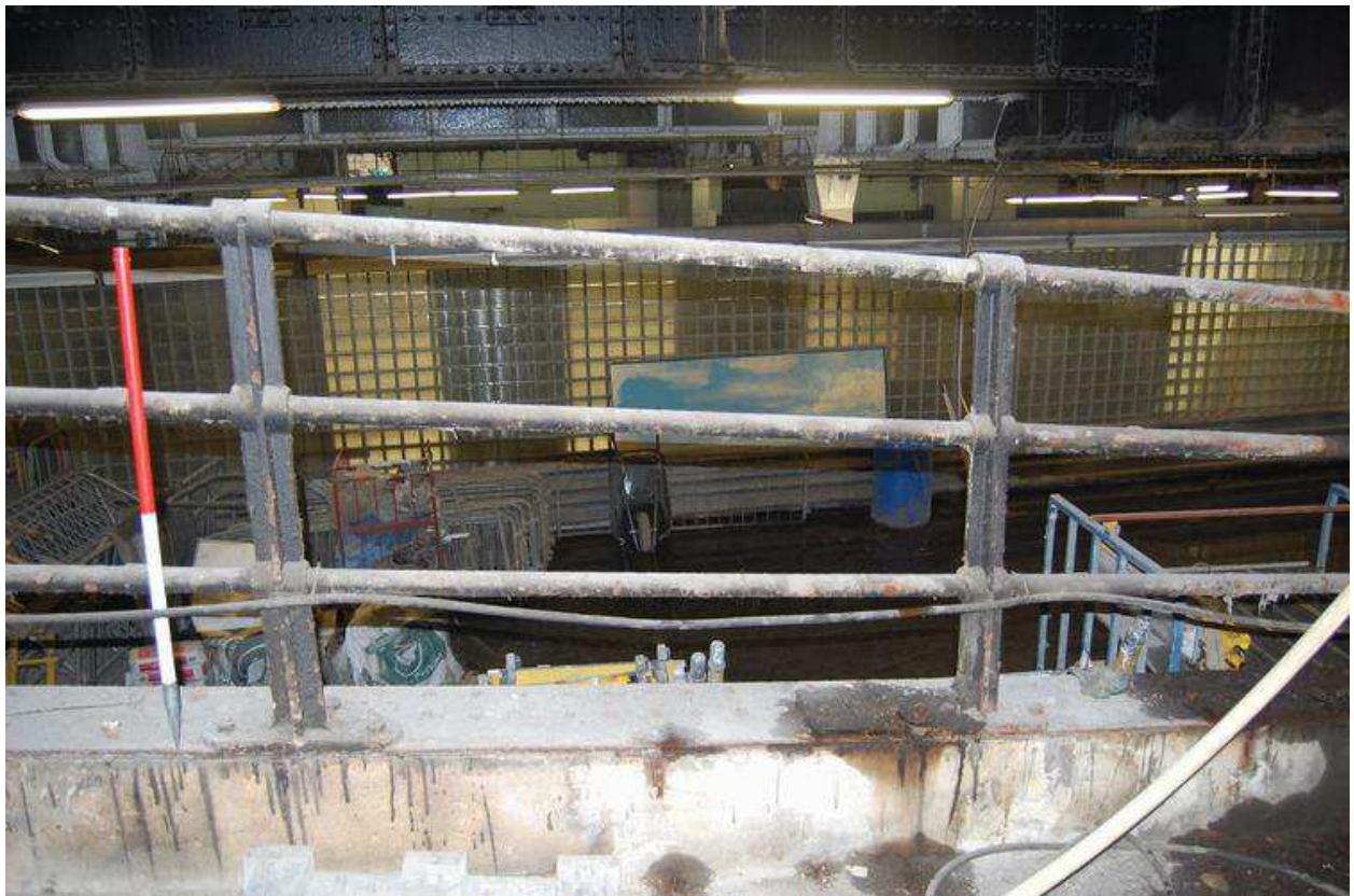
Plate 17: Detail of railings
