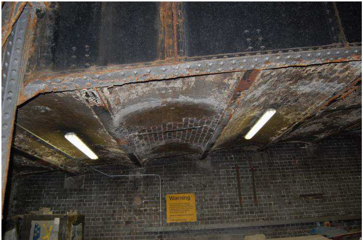
Plate 49: View of retaining wall below ramp – south end
