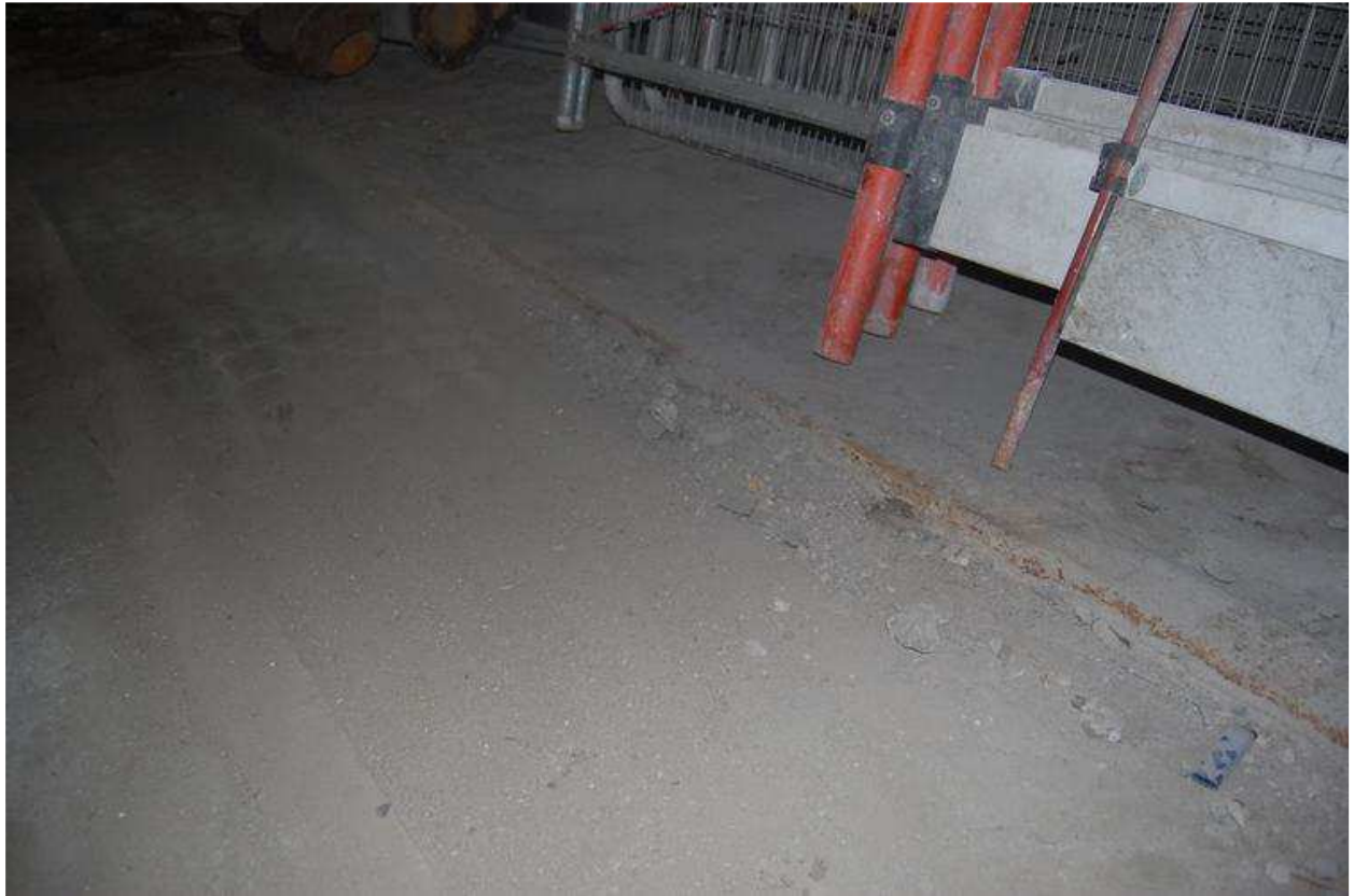
Plate 28: Detail of iron rail to edge of sett surface
