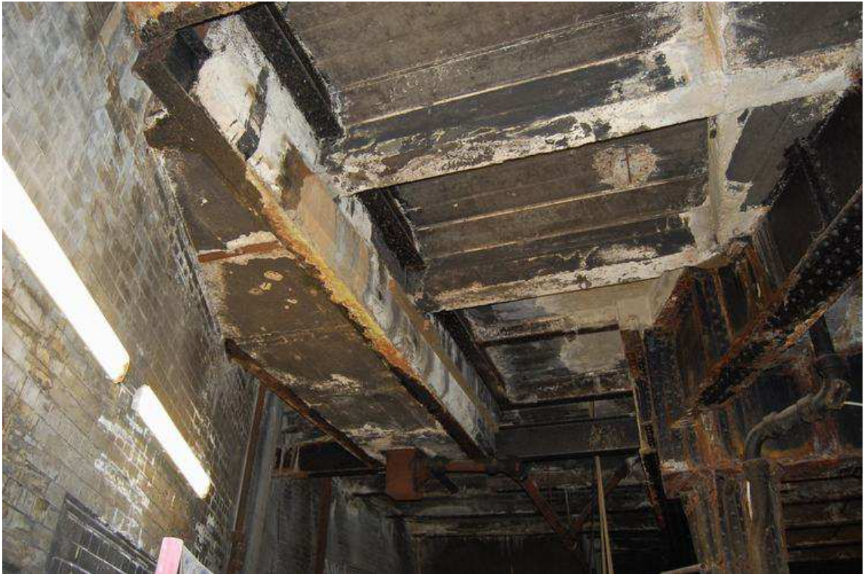
Plate 70: View of inserted inspection pit to south of ramp
