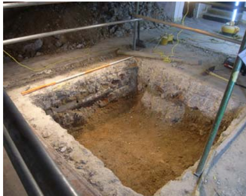
Plate 1: Test Pit 1 - Looking north west
