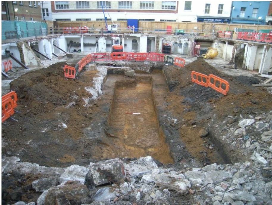
Plate 1: Uneven nature of the quarrying, looking west
