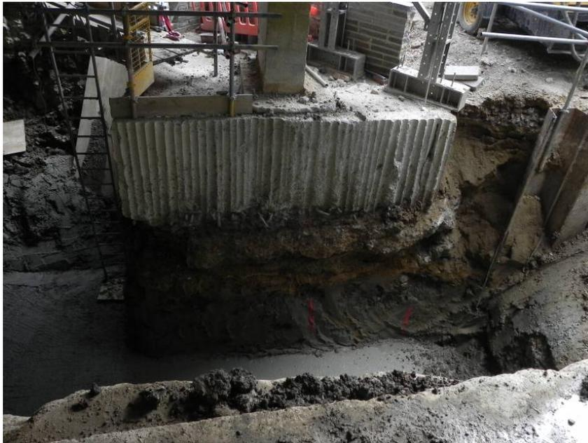
Photo 6 Sewer run S2–S3, foundation pads for Moorgate Underground ticket hall truncating to natural strata, looking east
