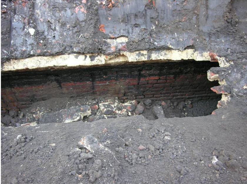
Photo 3, culvert [37] (provisionally) dated by brick types as early 19th-century or later, looking north.
