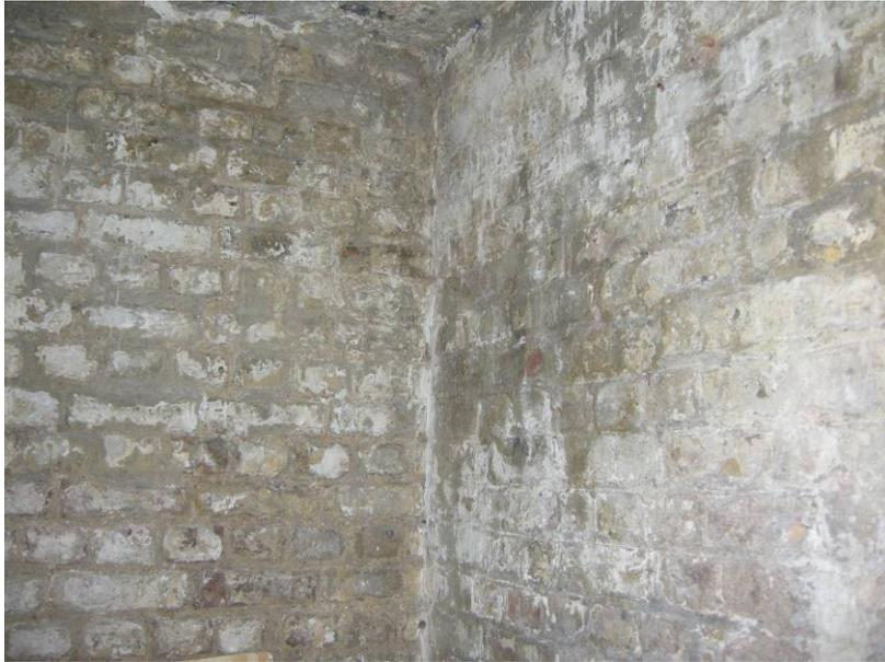
*Fig 54 Straight joint between trackside wall and later room partition, in second room from east, looking west*
