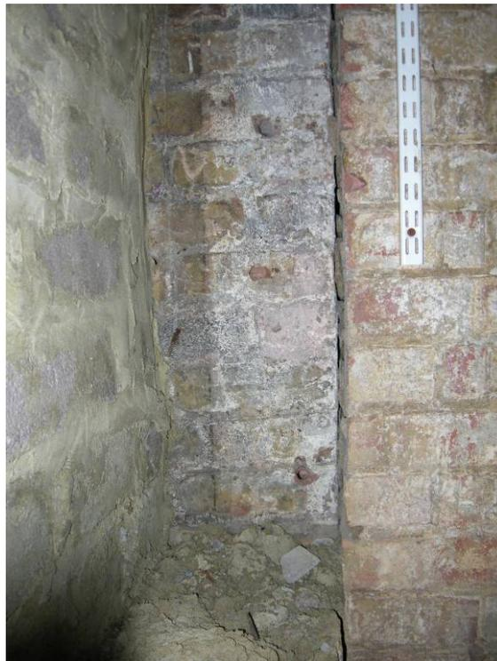
*Fig 53 Straight joint between trackside wall and later room partition, in second room from east, looking east*
