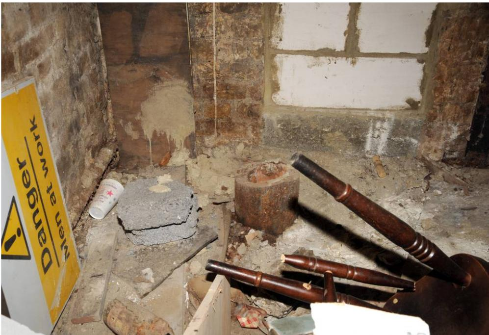
*Fig 31 The surviving stump of the direct acting hydraulic lift piston beneath the geometric staircase, lower ground floor level looking west*
