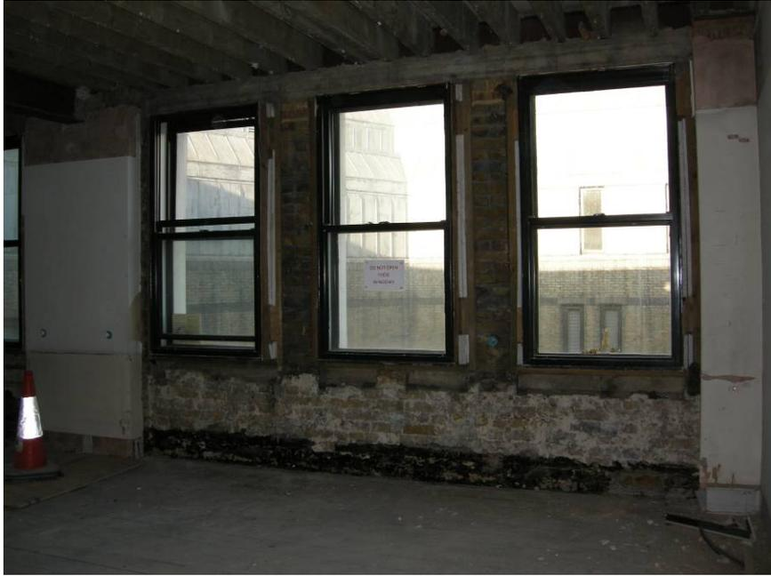
*Fig 40 Alterations around the windows in the second room from the west staircase, along the trackside, looking north*
