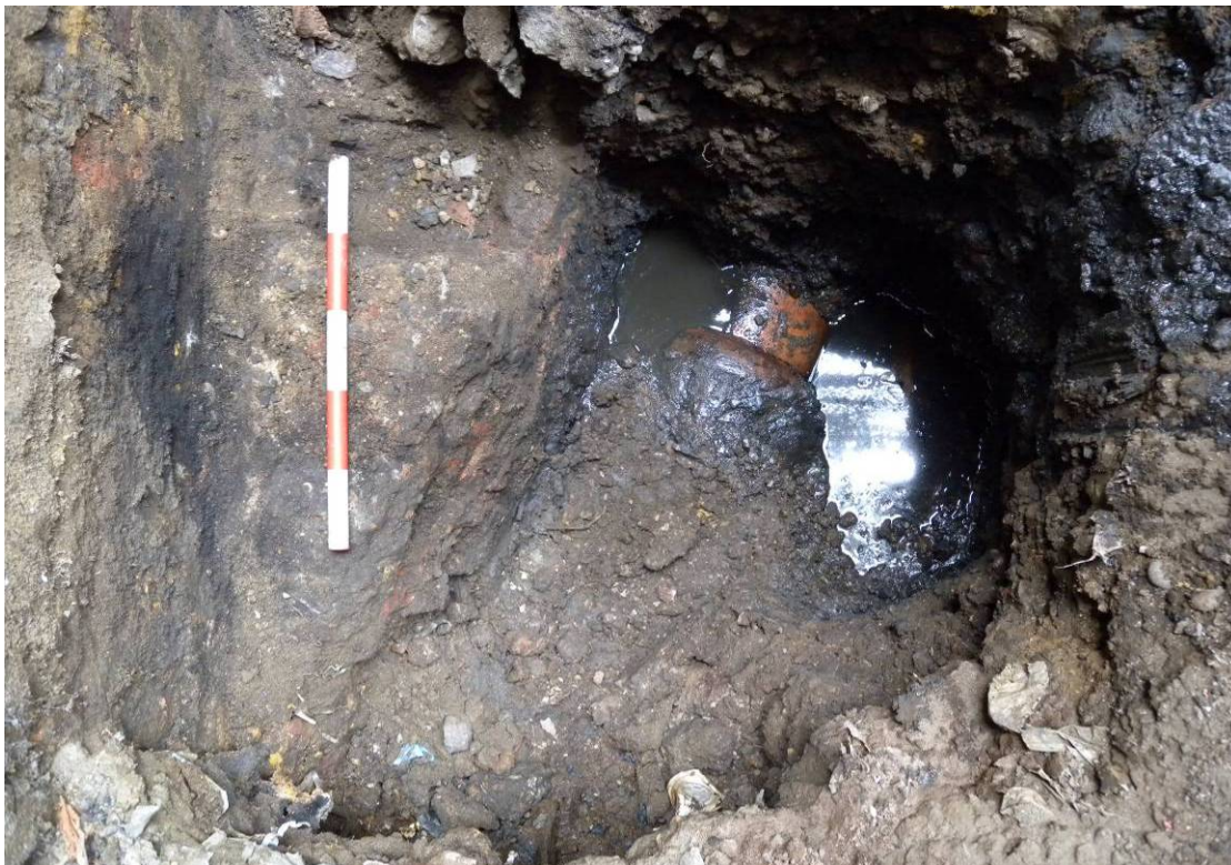
Photo 7 Test Pit TP/E3, looking north, showing foundations on the east face of pier F of Lindsey Street Bridge
