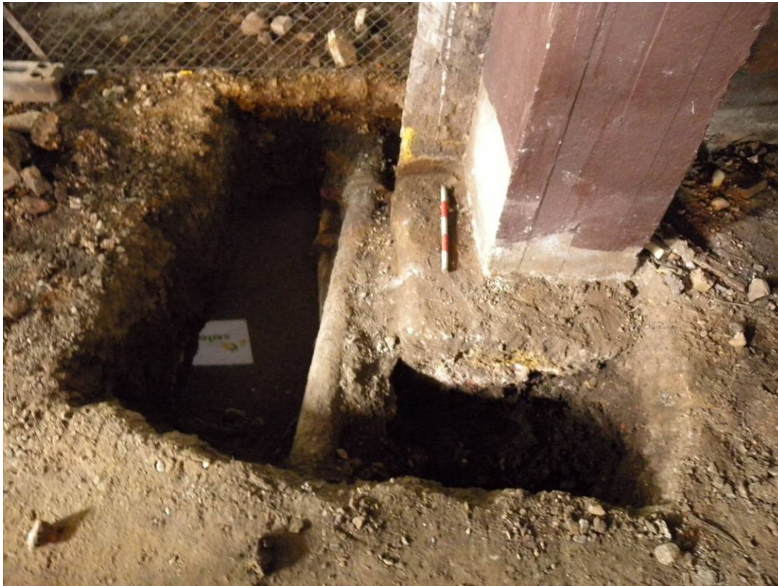
Photo 3 Test Pit TP/B1, looking west, showing foundations
