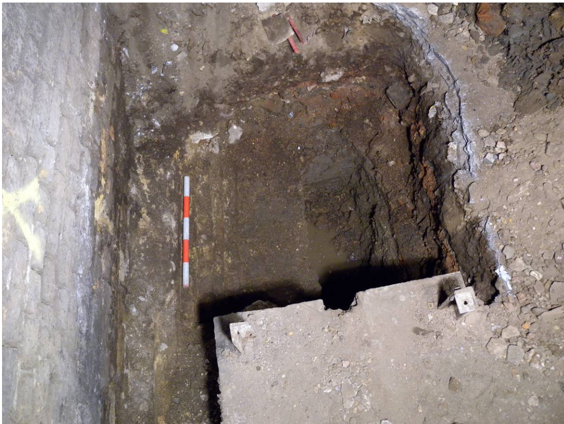
Photo 1 Test Pit TP/A1, looking east, showing foundations on south face of LUL party wall
