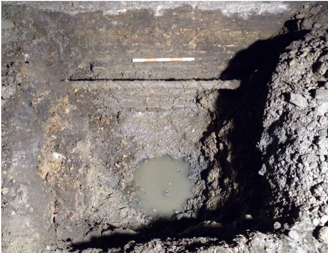
Photo 4 Test Pit TP/E1b, looking north, showing foundations on the south face of pier B-C of Lindsey Street Bridge
