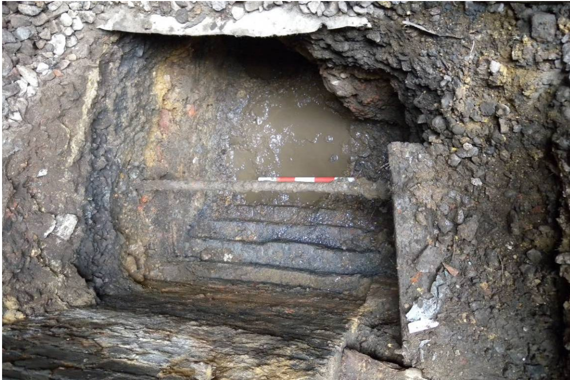
Photo 6 Test Pit TP/E3, looking south west, showing foundations on the north face of pier F of Lindsey Street Bridge
