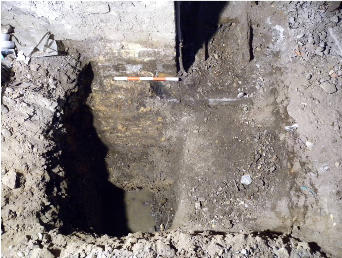
Photo 2 Test Pit TP/B1, east corner of LUL party wall, looking north, showing foundations
