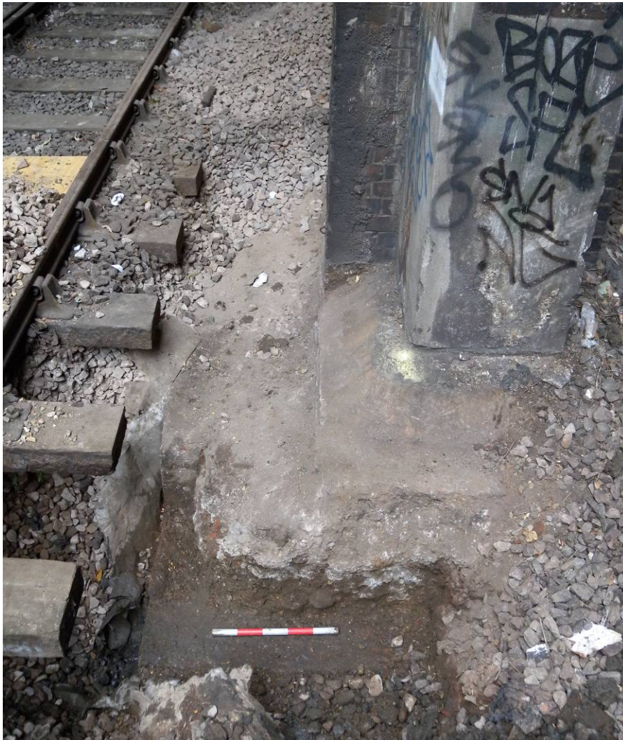
Photo 5 Test Pit TP/E2, looking south west, showing foundations of pier E of Lindsey Street Bridge
