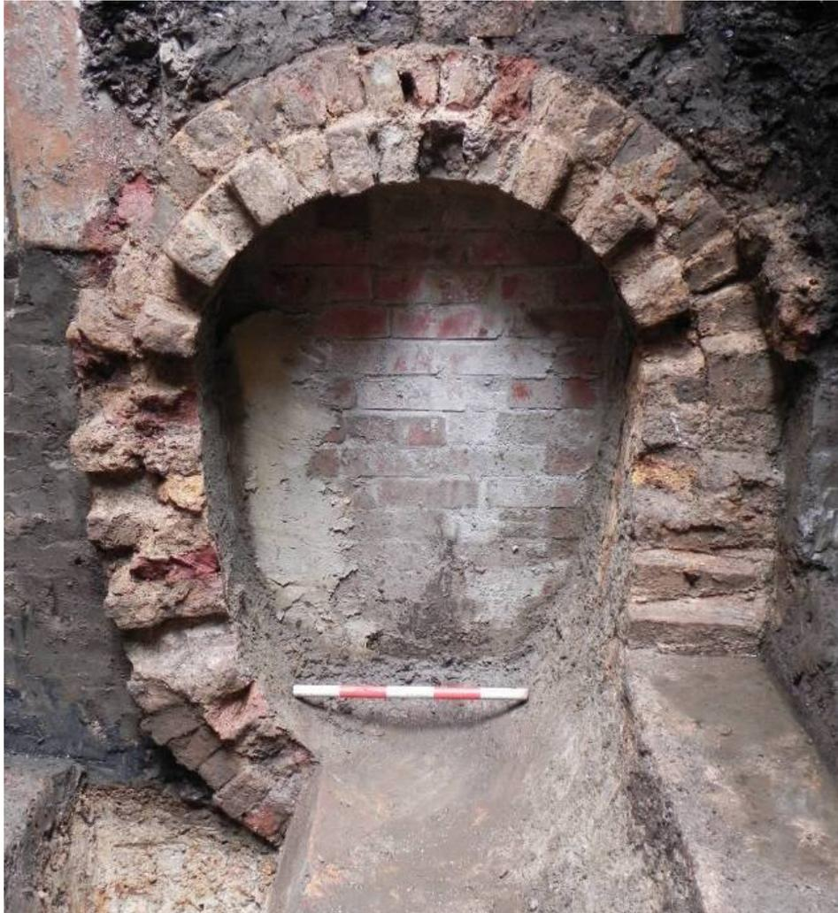
*Photo 4: Trench 1 - Profile of sewer [535] with a 0.5m scale. During the excavation it was backfilled and bricked up westward, and largely broken out within the trench (looking west).*
