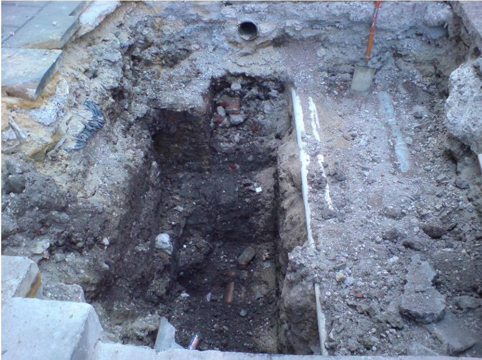
Photo 10: Trench 1a – Gas pipe (right) and telecommunication cables (white pipes), with a deeper utility trench (ceramic pipes) truncating the south half of the trench (centre and left)(looking west).
