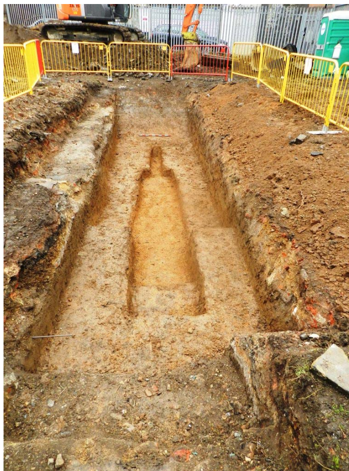
Temporary Shaft Evaluation Trench, looking north
