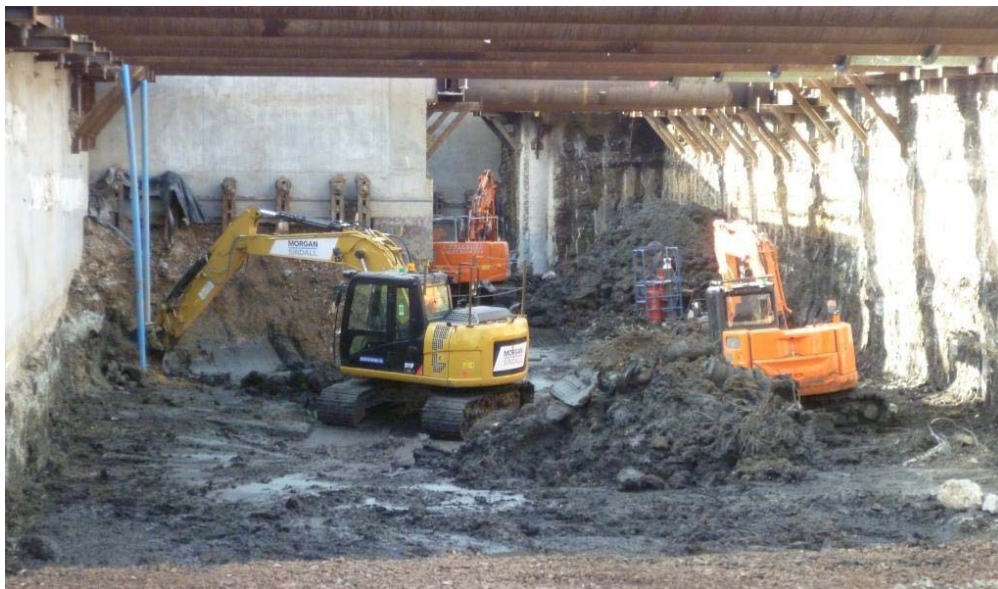
Photo 6 Exposing the top of alluvium at the level for the second layer of props, Cut and Cover 3, looking east 24th February 2015
