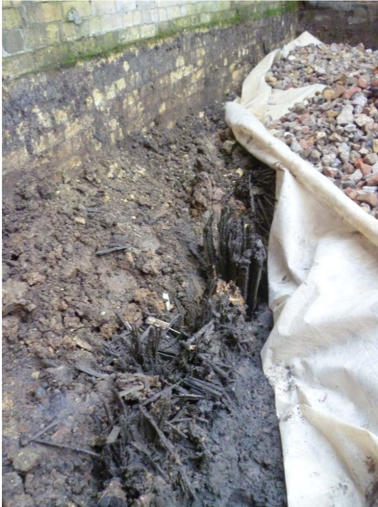
Photo 8 Timbers [127] looking north, with in-filled City Mill River to the right (east) and the Great Northern Outfall Sewer, 11th January 2012
