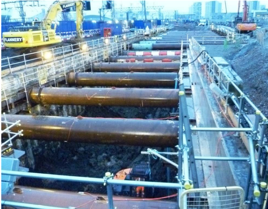
Photo 5 , Excavation of Cut and Cover (Section 3) looking east, 19th February 2015
