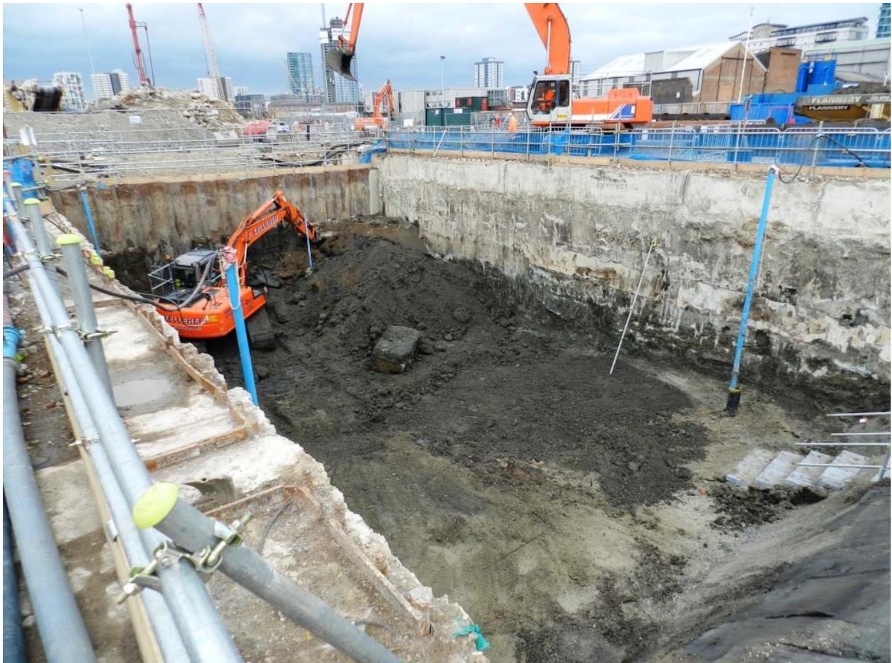
*Photo 5 Cut and Cover Section 1 excavating through alluvium and into natural terrace gravels (last of concrete intrusions removed), looking east, 1st Feb 2011*
