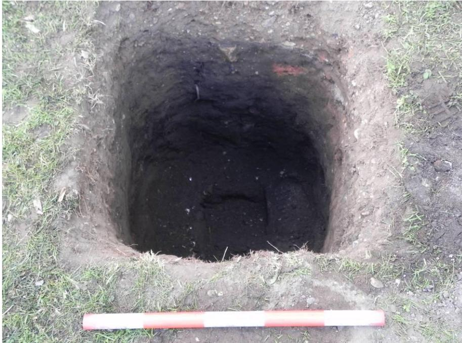
Photo 3, starter pit for borehole WH\_59, looking north
