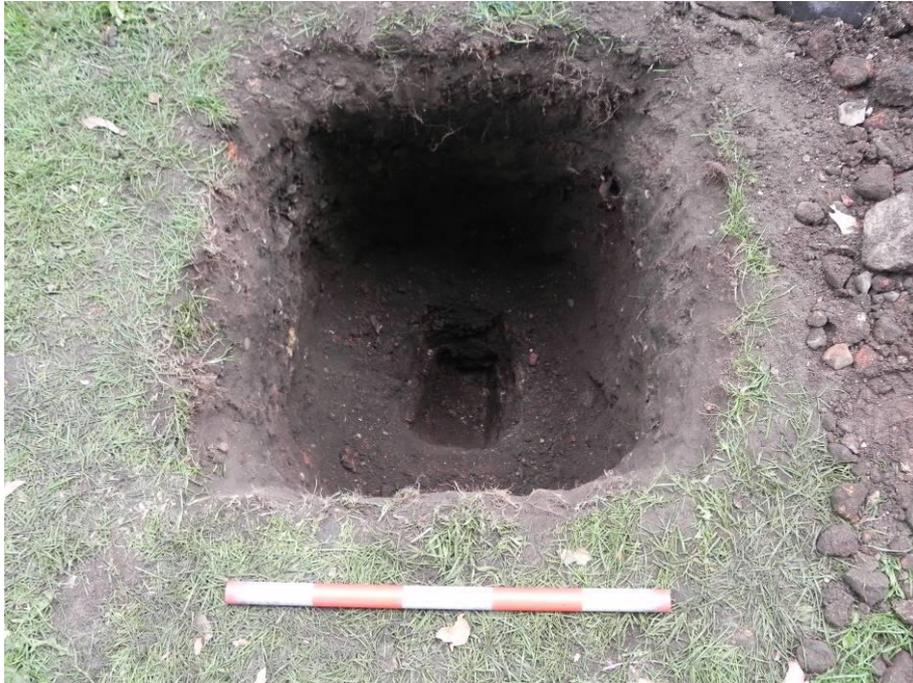
Photo 6 starter pit for borehole WH\_62, looking east
