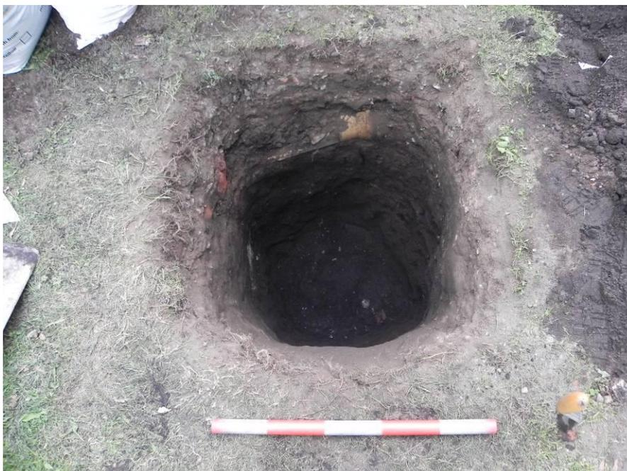
Photo 8 starter pit for manhole XR\_50901, looking north
