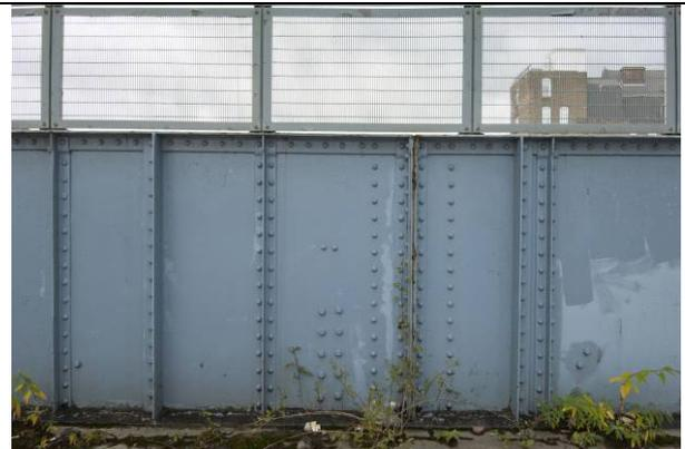
Fig 24 Cast iron panels along the sides of the Woods Buildings footbridge
