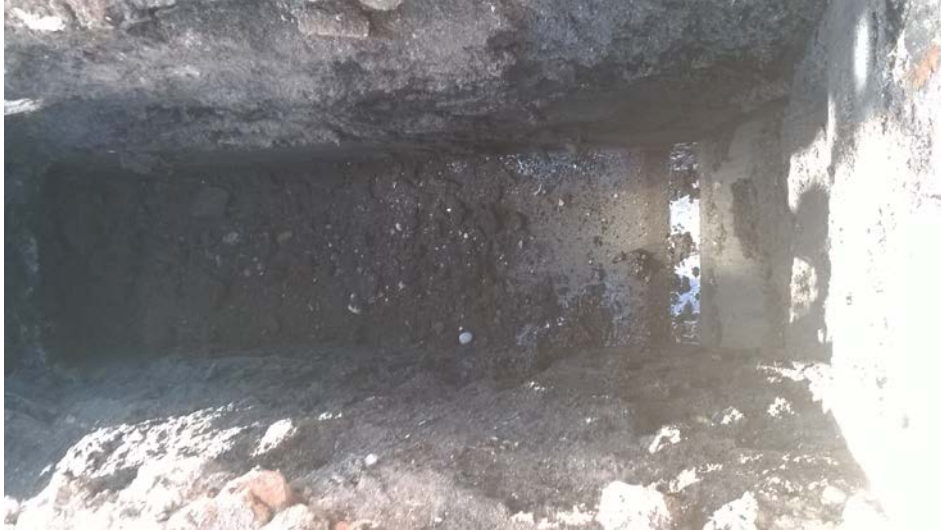
Photo 4 Trial Pit TP F, looking north.
