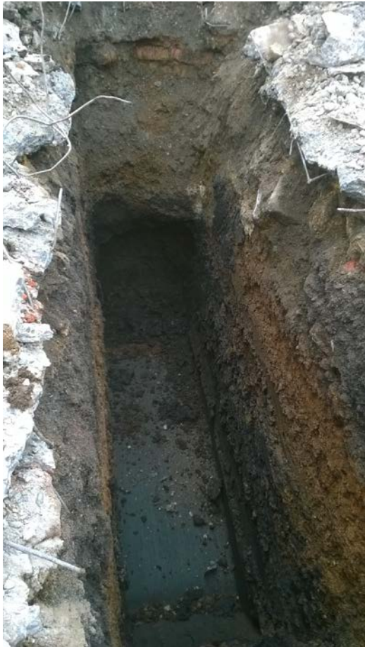
Photo 2, Trial Pit TP C, looking south.
