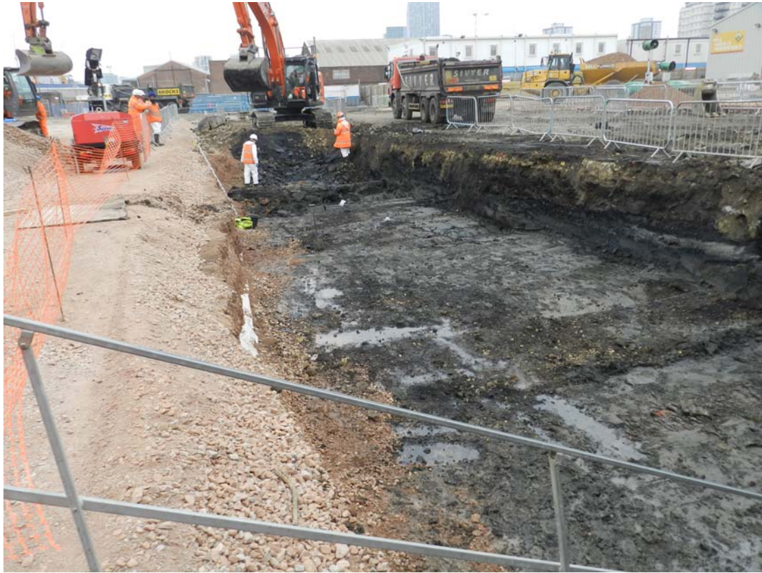
Photo 1 Showing excavation of strip 9 with exposed alluvium, looking north-east
