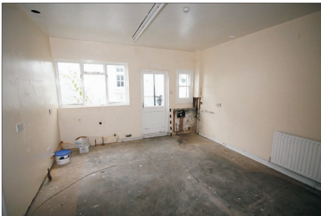
Plate 3: Ground floor kitchen with inserted double casement window
