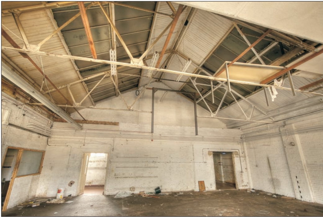
Plate 9: Central factory working space with compound fink trusses supporting the roof
