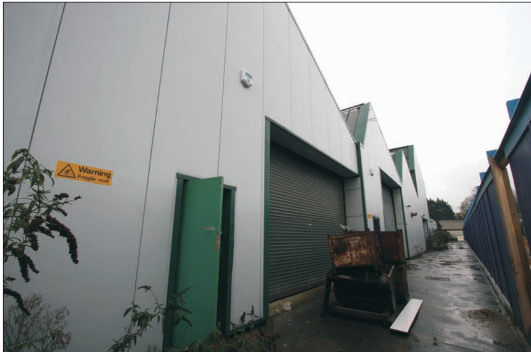
Plate 19: Various openings in north-west elevation
