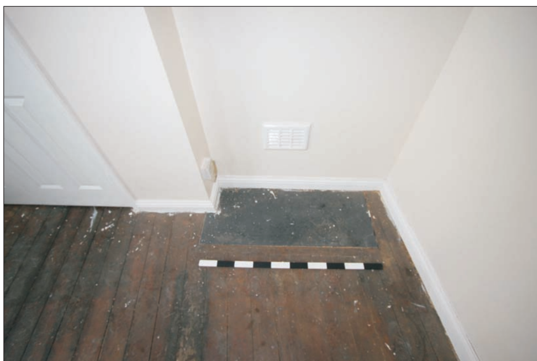
Plate 4: First floor north-west bedroom. Hearth with blocked fireplace in north wall. Modern dividing stud wall to right of image
