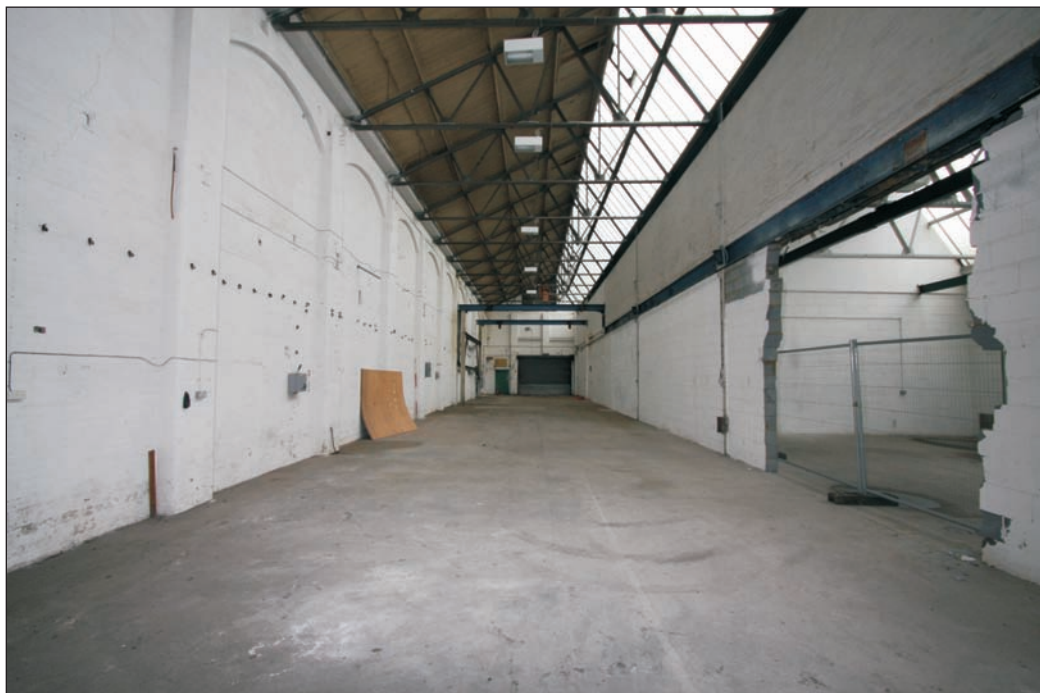
Plate 20: Raised south-west bay showing evidence of travelling crane rails in opposite walls
