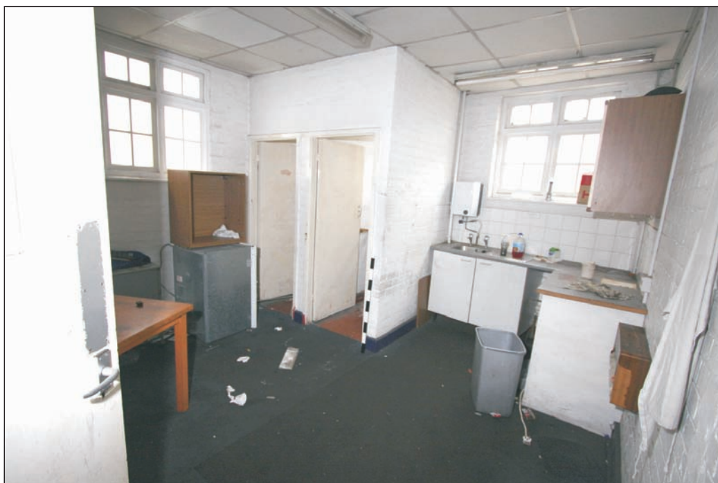
Plate 15: Internal view of kitchen and toilets on north side of building
