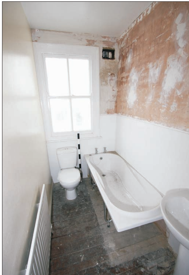
Plate 7: First floor bathroom
