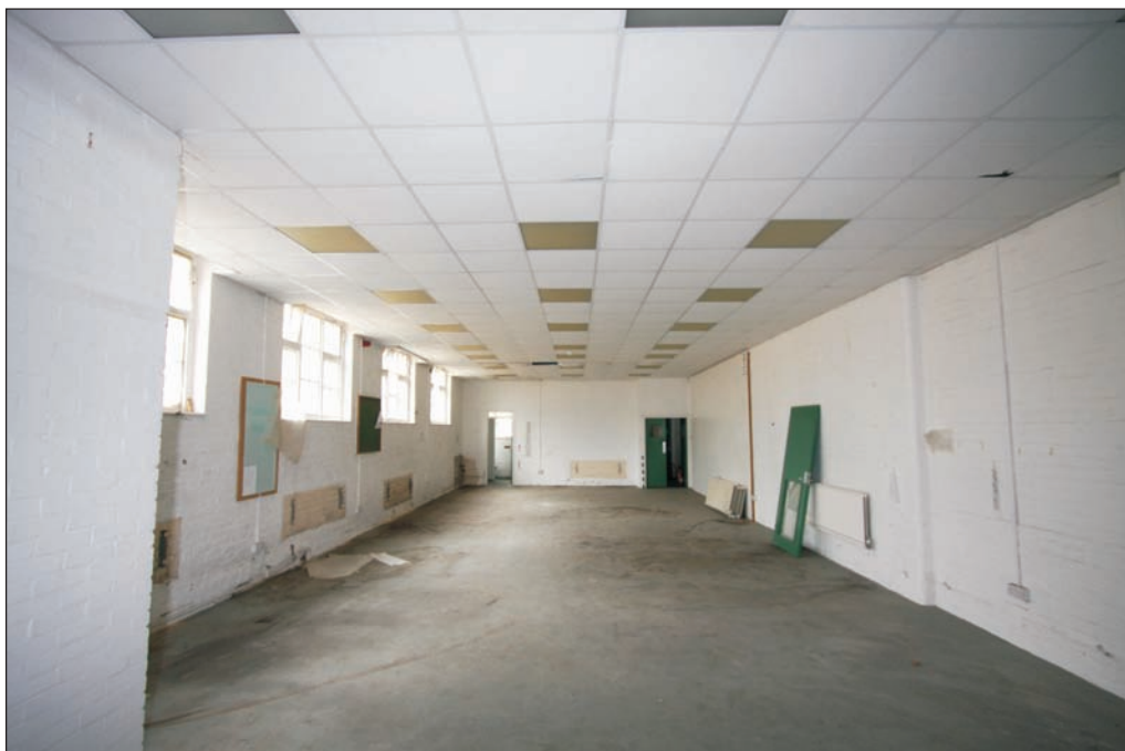
Plate 12: Ground floor south-east wing looking south
