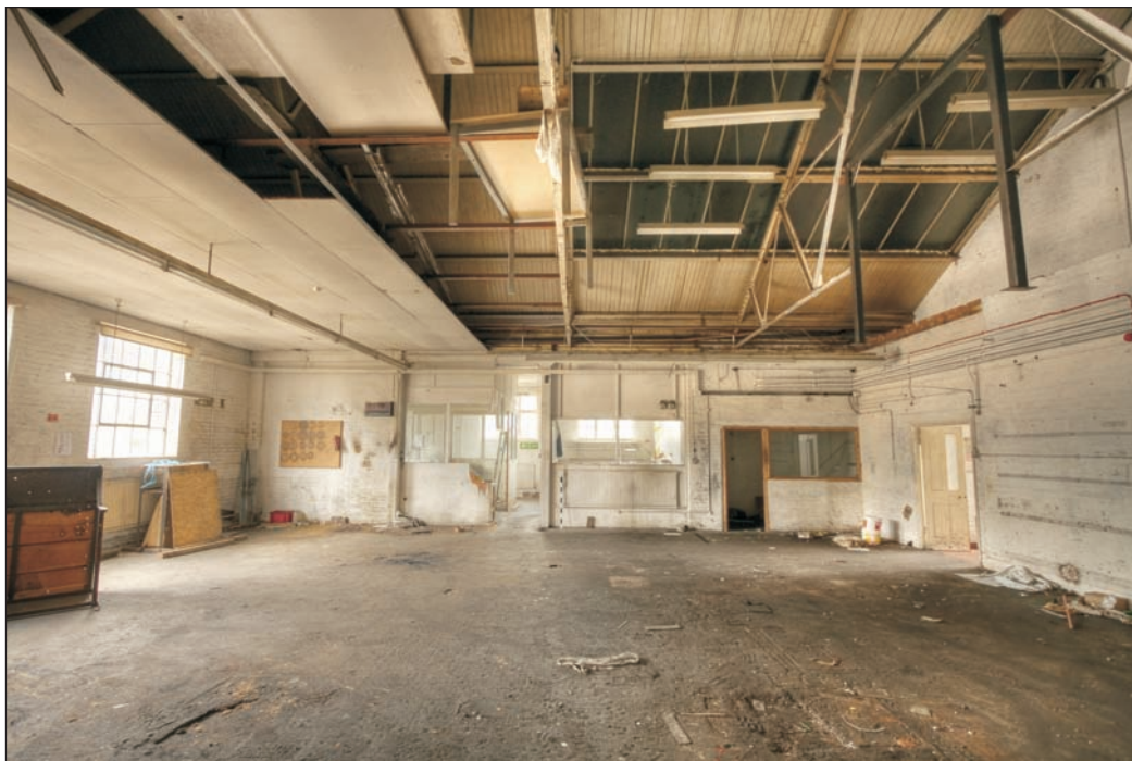
Plate 10: View looking north-west showing ground floor offices and stores created by knocking through north-west wall of factory space
