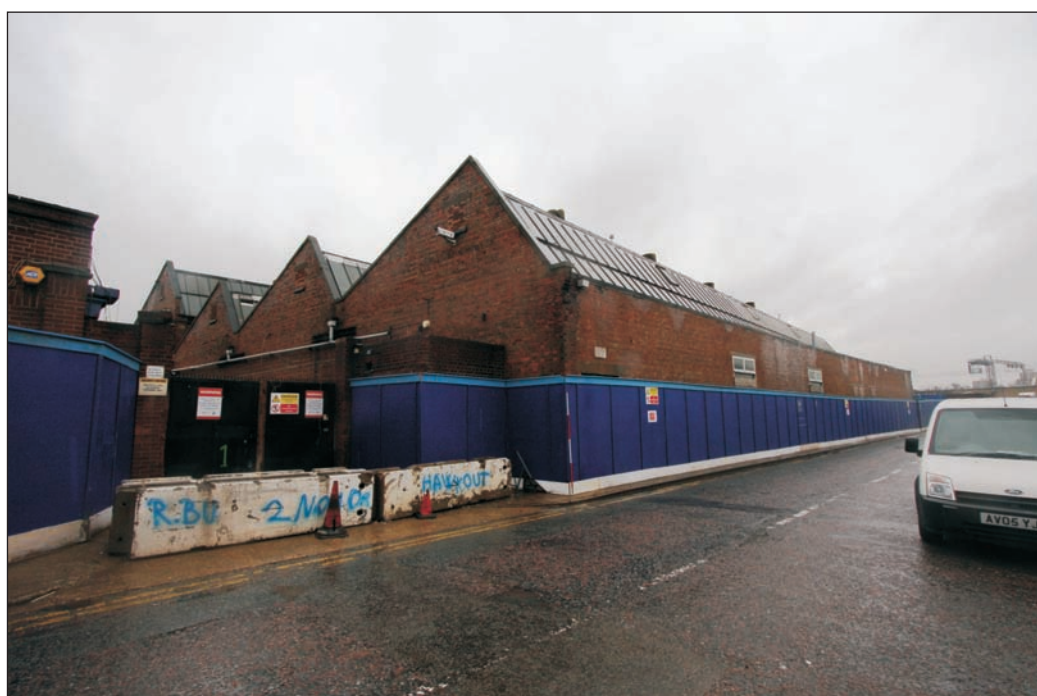
Plate 18: Exterior view of building 2 showing red brick walls and north-lit roof profile
