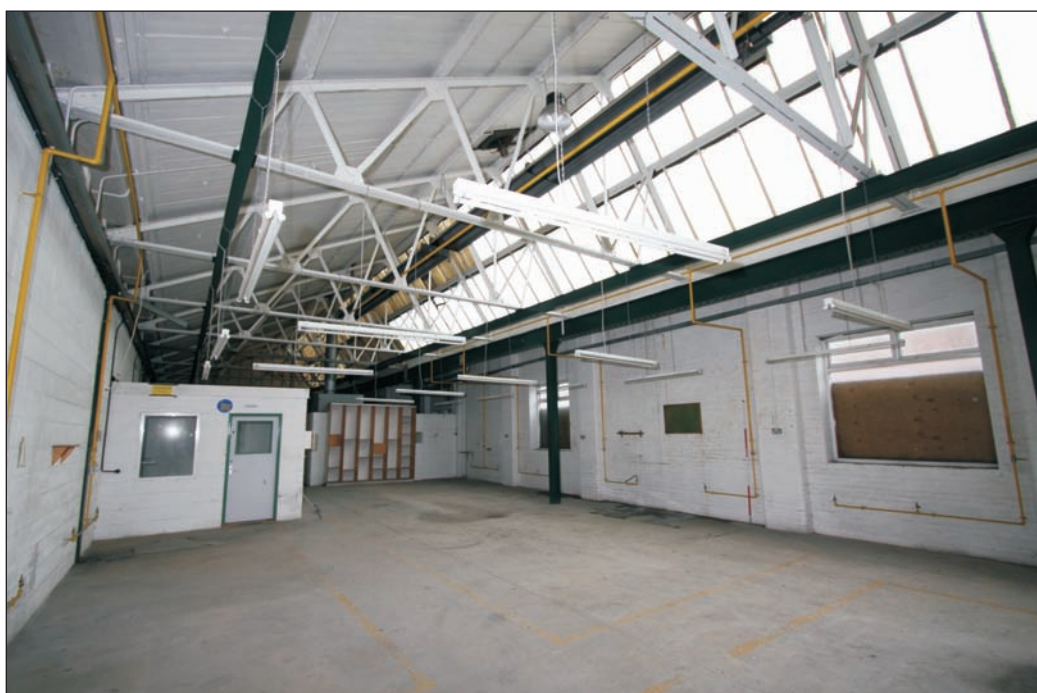
Plate 17: Building 2, typical view showing internal steel frame and north-lit roof design plus modern office divisions
