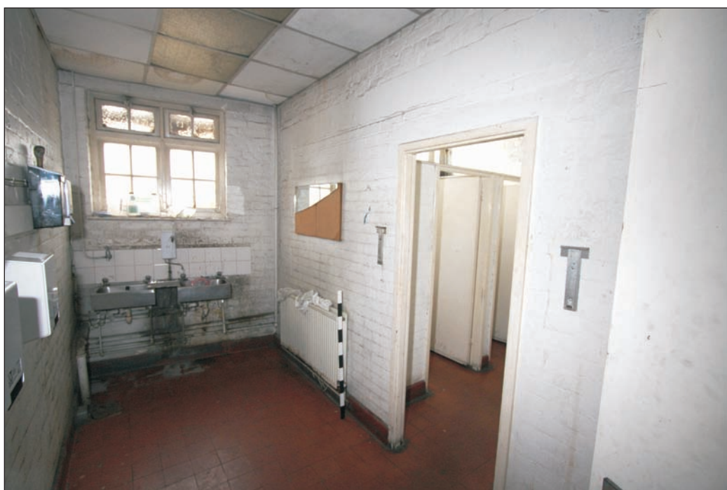
Plate 16: Internal view of toilets showing quarry tile flooring and wooden framed windows
