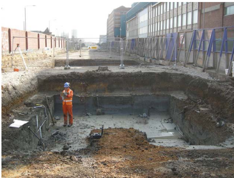
Photo 3 Looking east, sampling of upper alluvial deposits.
