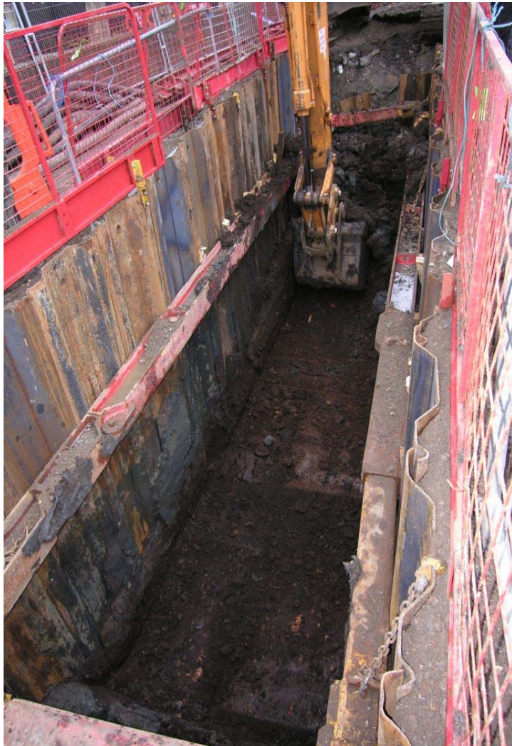
Photo 3 Sewer Diversion, working shot of trench excavation showing mid-brown organic peat deposit between 2.3-3.2m bgl, looking north-east.
