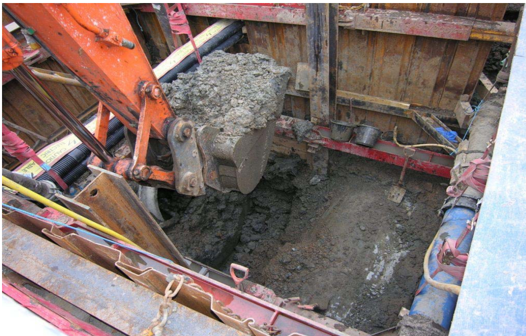
Photo 7 ARW5 Chamber showing excavation of blue-grey minerogenic alluvial clay [1] to the south of the existing brick culvert between 4.00-4.70m bgl, looking south-west.
