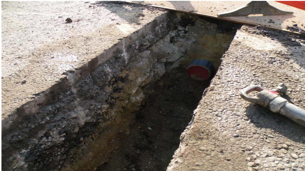
Photo 8 125mm Water Diversion on Albert Road looking south showing modern made ground to 1.5m bgl, looking south.
