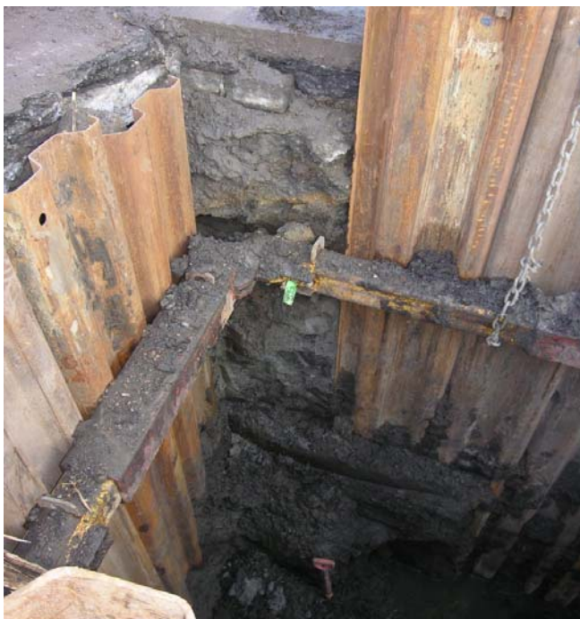
Photo 2 Sewer Diversion showing north profile to 4.5m bgl with modern overburden overlying blue-grey minerogenic alluvial clay [1], looking north.
