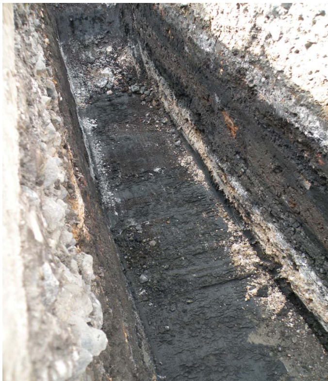
Photo 19 Gas diversion trench showing made ground overlying a blue-grey minerogenic alluvial clay [1] showing at 1.3m bgl, looking west.
