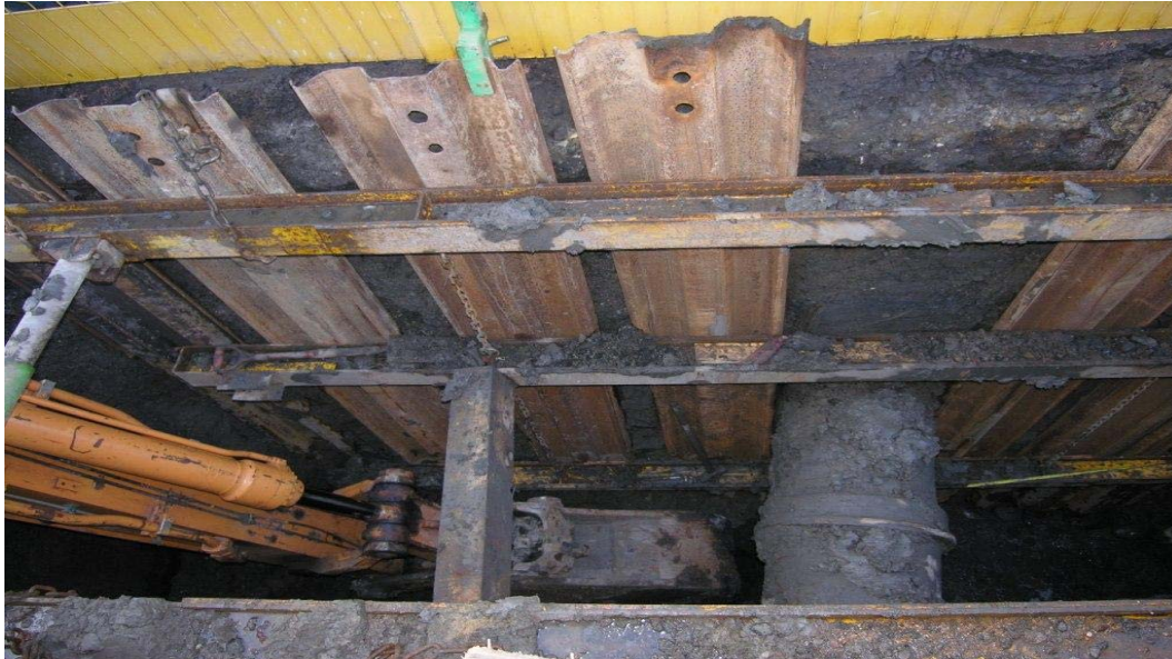
Photo 10 Working shot of excavation of sewer diversion trench showing utility running north to south with overlying redeposited material, looking south.
