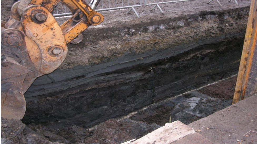
Photo 1 Sewer Diversion, working shot showing modern overburden and granite setts overlying blue-grey minerogenic alluvial clay[1] on the south facing section to 2.10m bgl, looking south-west.
