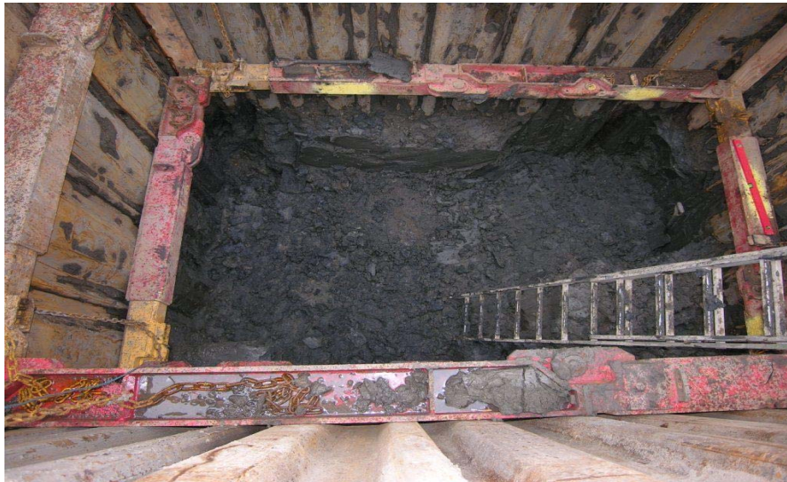
Photo 15 Elliptical Sewer connection chamber on Factory Road, looking south.
