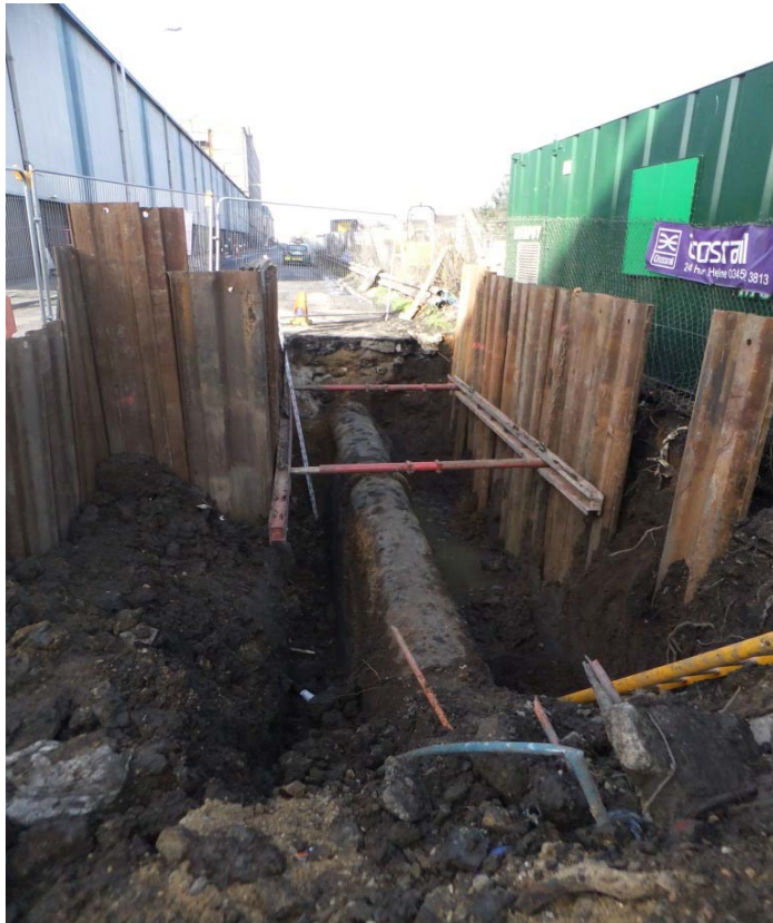
Photo 12 FRW1 showing modern made ground and utility pipe running east to west across trench, looking west.
