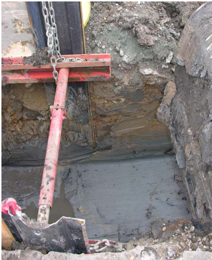
Photo 9 Gas and Water diversion trench showing modern overburden overlying a grey-blue minerogenic alluvial clay [1] appearing at 1.40m bgl, looking north.
