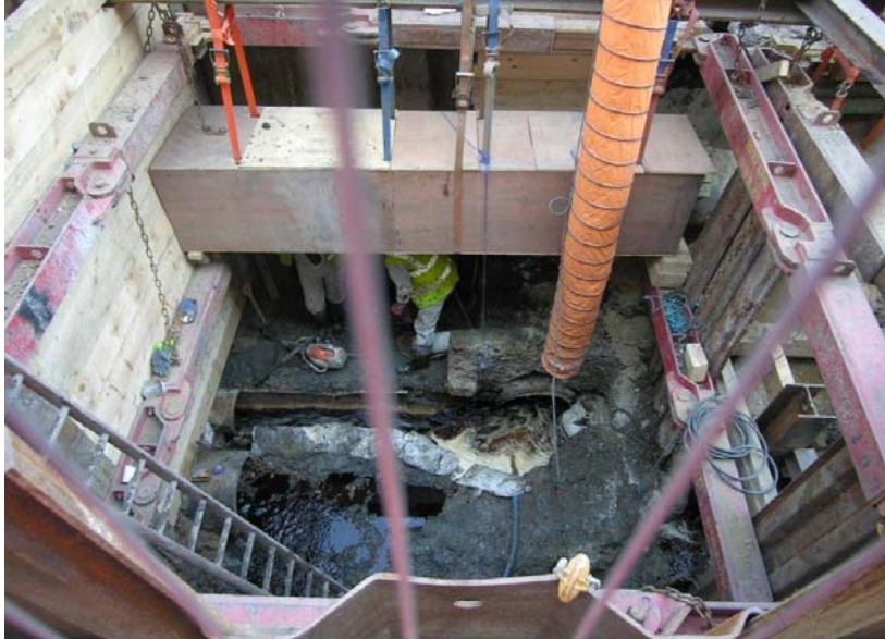
Photo 16 Sewer chamber at circa 3.5m bgl showing open sewers laid into blue-grey minerogenic alluvial clay [1], looking north.
