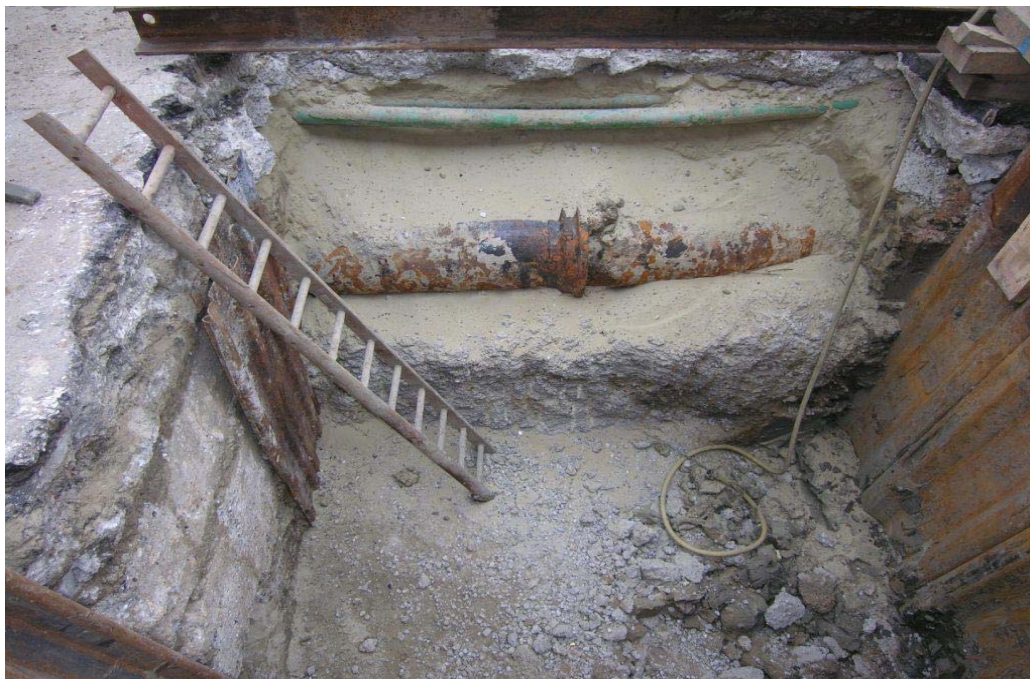
Photo 14 Connection chamber between FRW1 and FRW2, showing concrete to the north and west, looking north.
