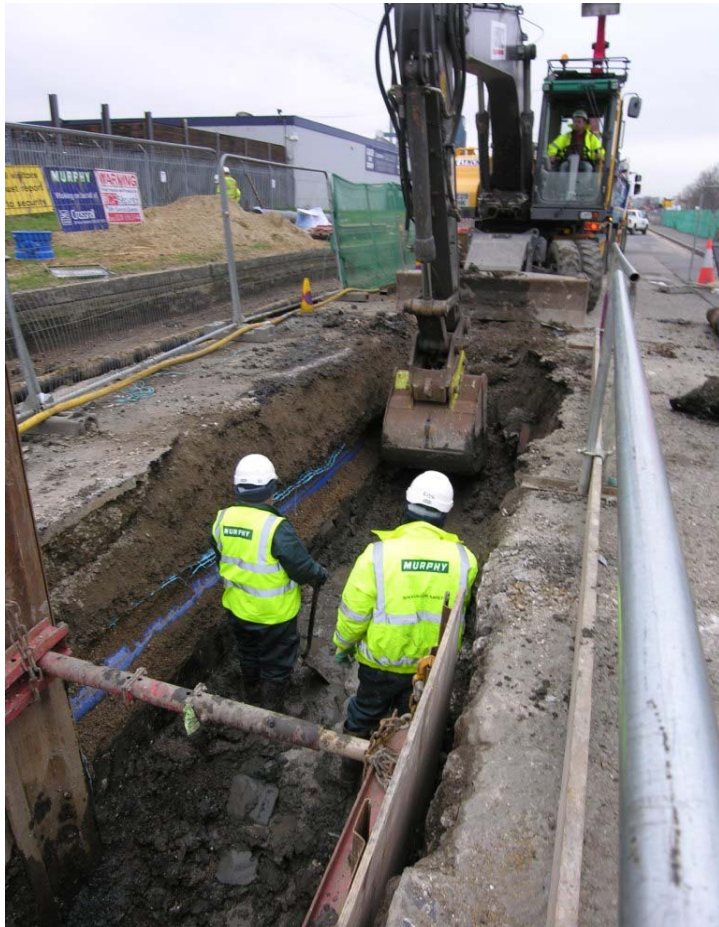
Photo 18 Excavation of 560mm water diversion showing blue-grey minerogenic alluvial clay [1] at 1.80m bgl, looking west.
