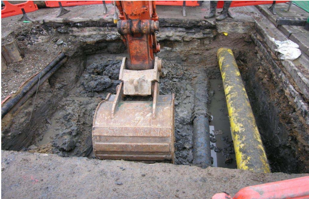
Photo 6 ARW5 Chamber showing excavation of redeposited blue-grey minerogenic alluvial clay [1] to 1.2m bgl. Gas and water utilities to the north. Looking west.
