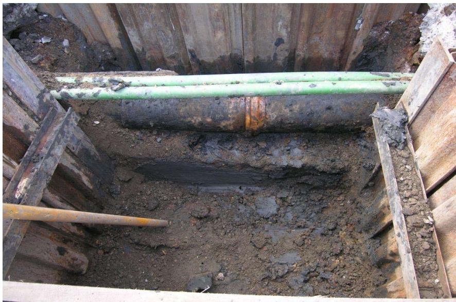
Photo 13 FRW2 showing utility overlying blue-grey minerogenic alluvial clay [1], looking north.
