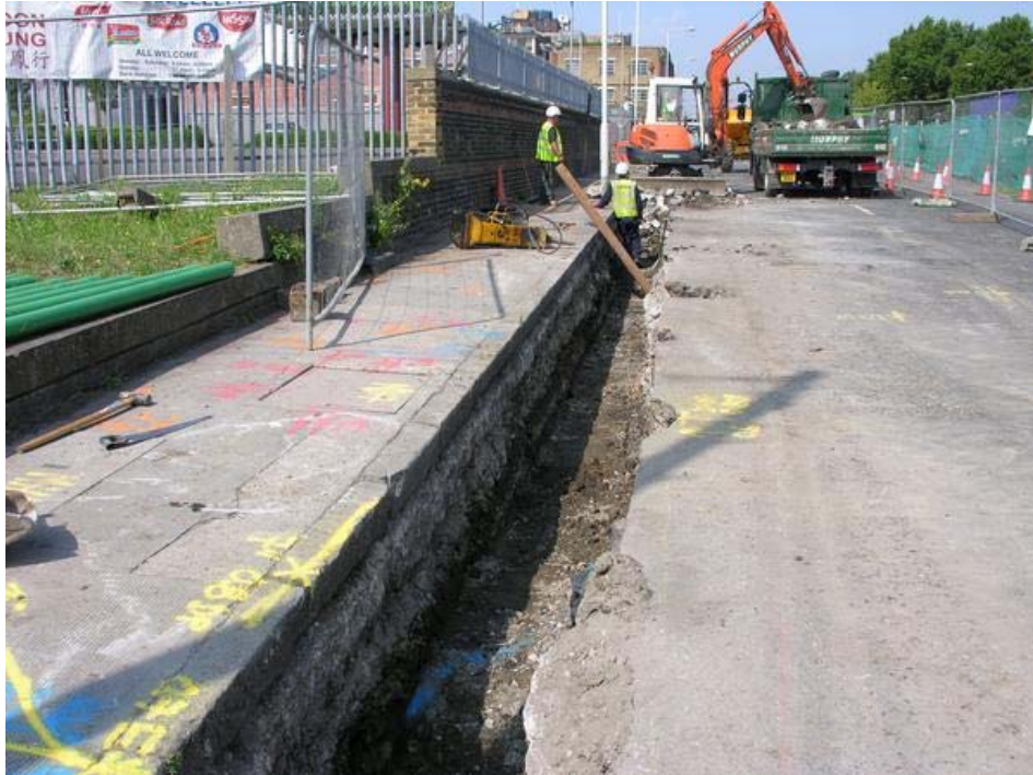
Photo 20 BT, Virgin, EDF and Interroute diversion trench, along the pavement edge on the south side of Factory Road, looking west.
