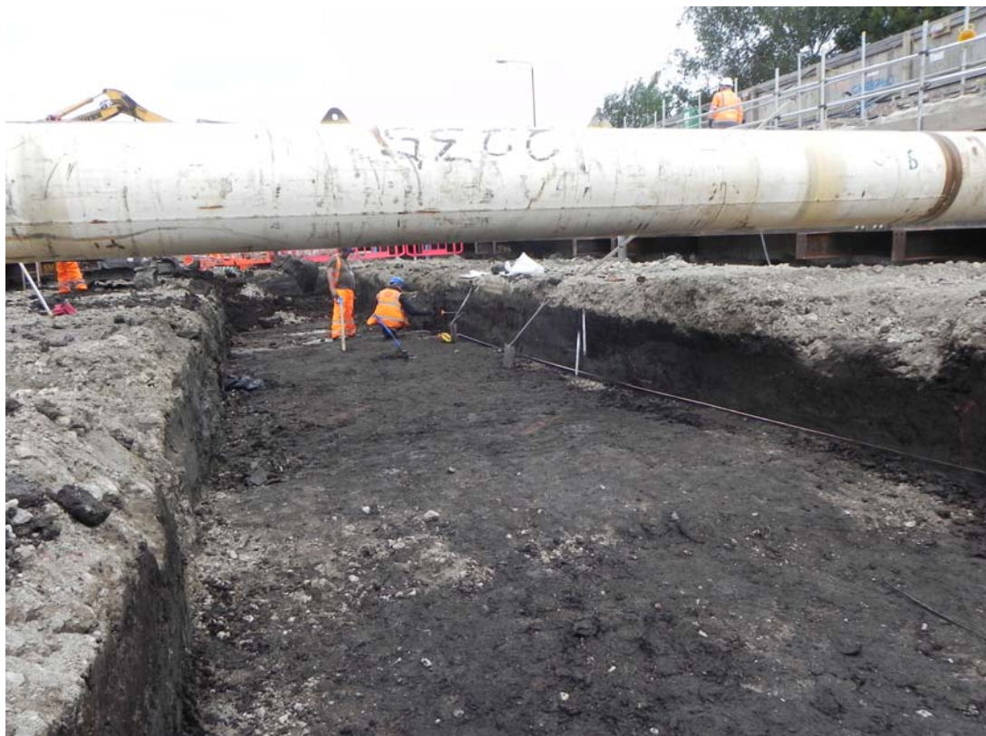
Photo 3 Trench 3 after machining to c.98.9mOD
