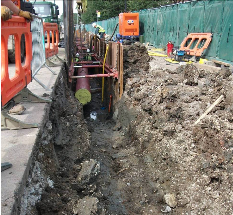
Photo 3 Eastern end of the gas main diversion trench, looking west.
