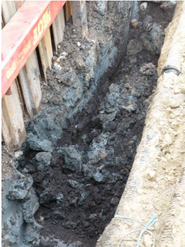
Photo 5 Southern edge of the Victoria Dock Road sewer excavation pit, located at the junction with Bridgeland Road, looking west.
