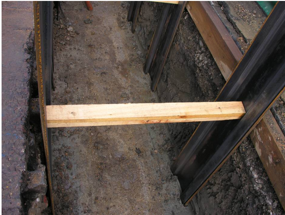
Photo1 EDF/Thames Water Diversion Trench, with another modern service trench running along the centre, looking north-west.
