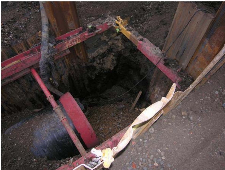
Photo 6 Sewer/Foul Water Drainage Diversion Trench showing peat deposits overlain by alluvial clay and modern made ground, looking south-west
