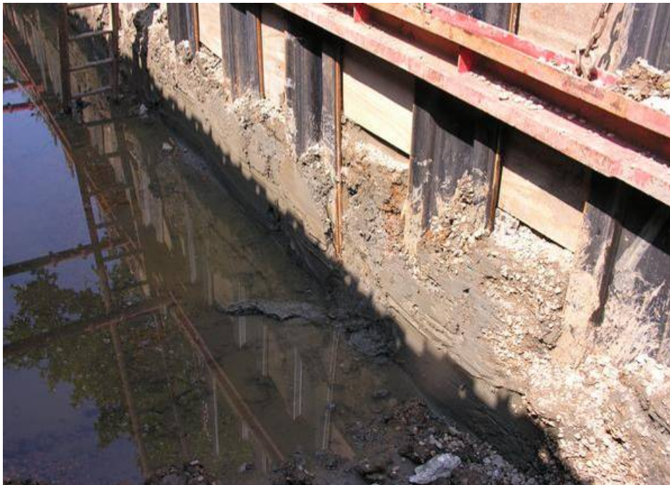
Photo 4 Gas main diversion trench, south-facing section, looking north-west.
