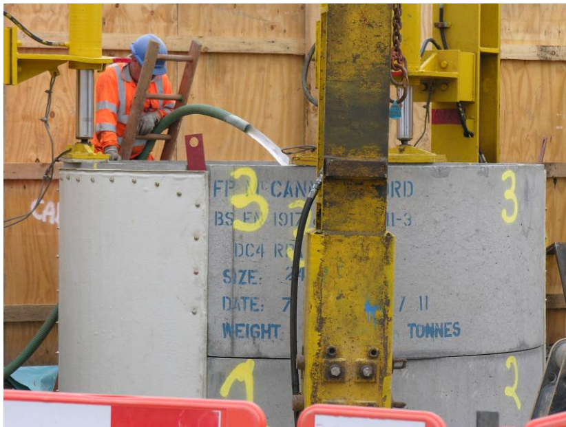
Photo 8 SL4a, showing the concrete rings and process of artificial flooding
