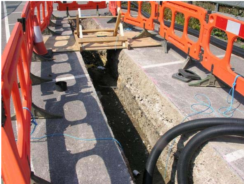
Photo 10 The western end of the EDF Diversion Trench, looking north-west.
