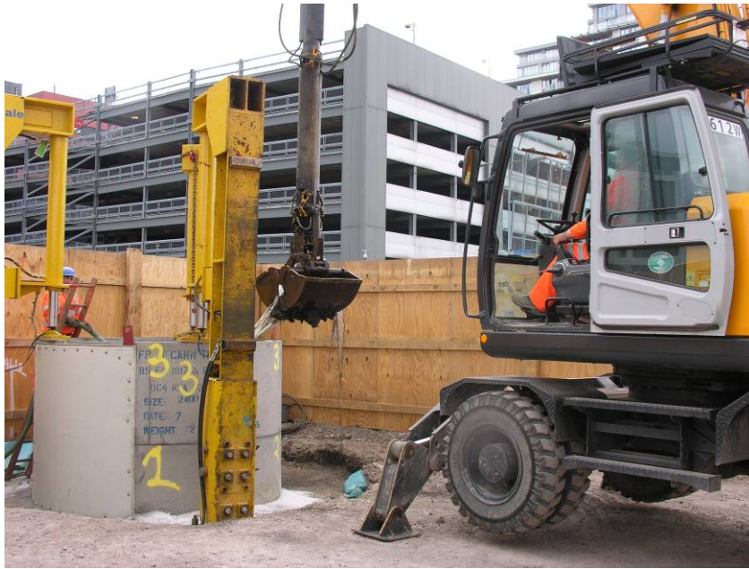
Photo 9 Excavation of SL4a showing the limitations imposed to archaeological observation by the construction methodology
