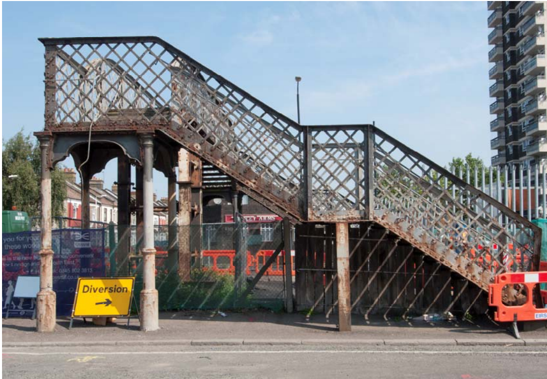
Photo 6 The southern façade of the structure, looking north. Note the RSJ replacing the small column.
