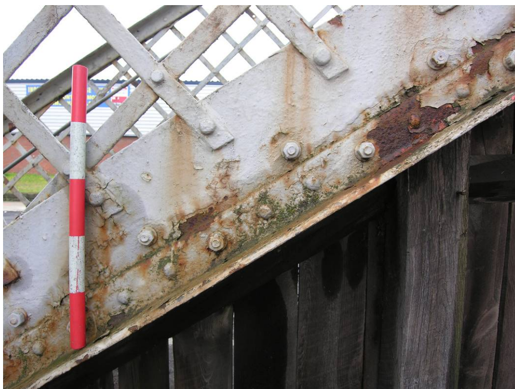
Photo 5 Rivets and bolts in the string panel of the southern steps, the rivets securing the lattice bars, whilst the pairs of bolts secure the brackets for each of the timber steps.
