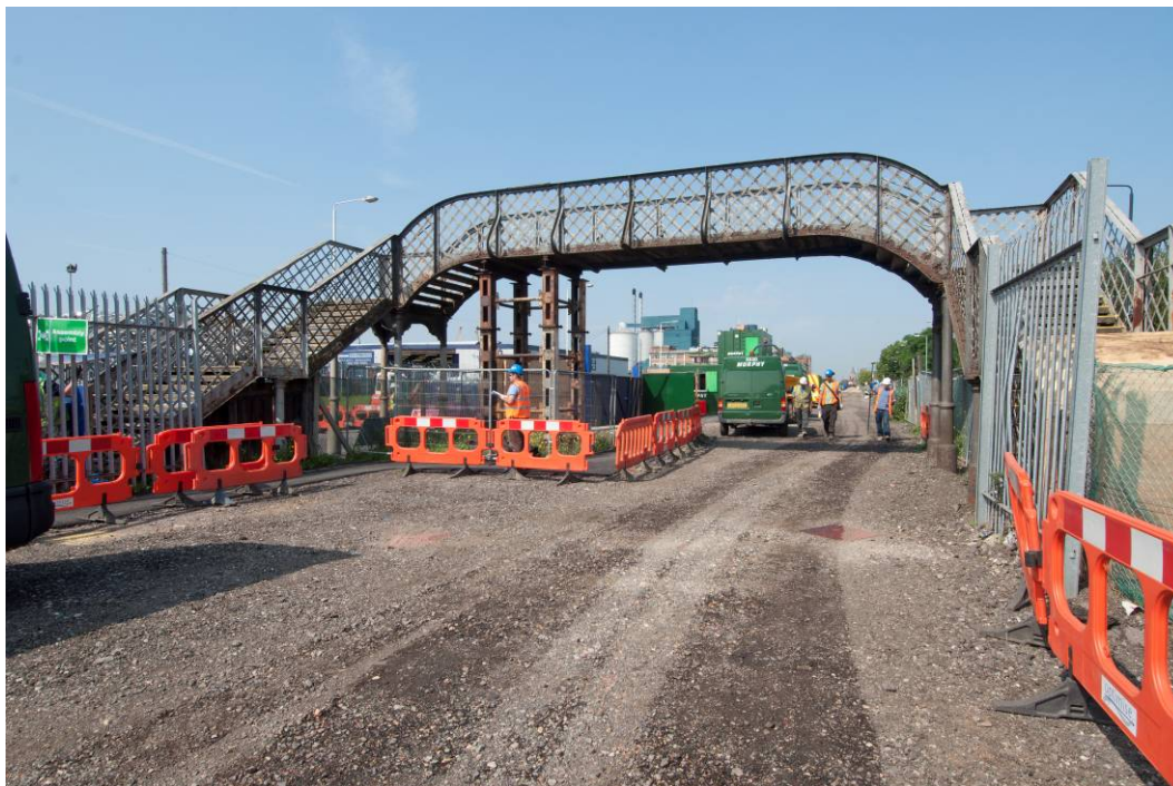
Photo 1 A general view of the late 19th century footbridge looking west
