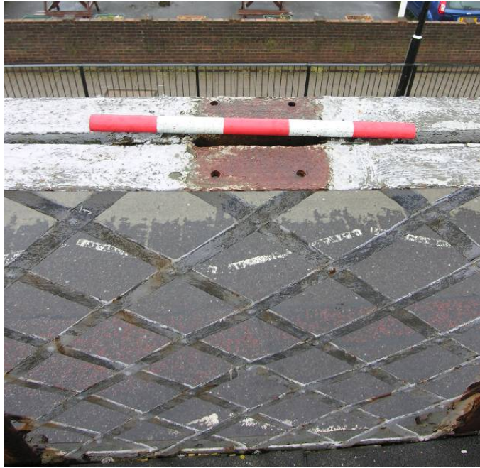
Photo 8 A scar on the upper surface of the foot bridge top-rail looking north, possibly from a lamp fixing or illuminated sign
