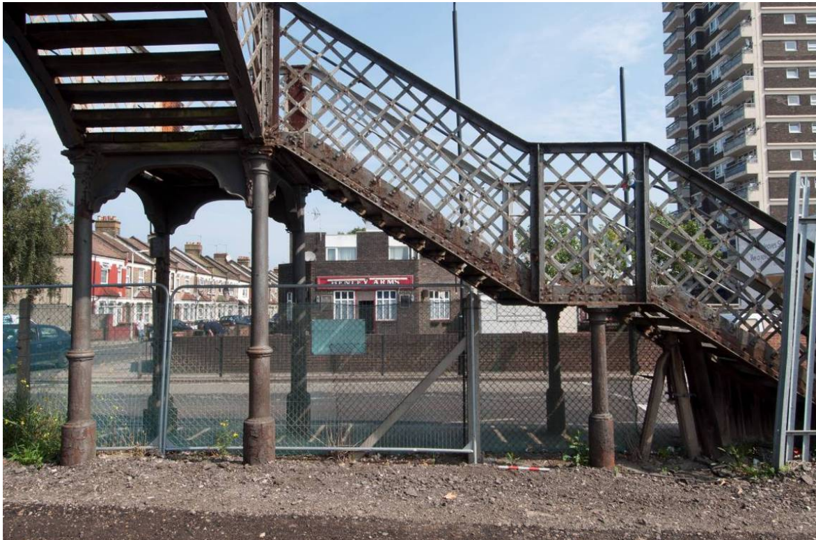
Photo 2 A view of the columns and staircase on the north side of the foot bridge, looking north
