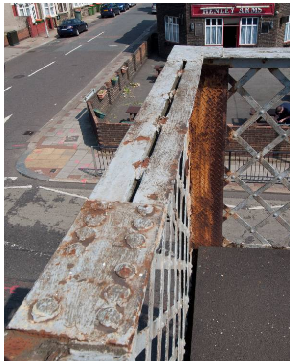
Photo 9 A fish plate securing two 'L' bars the foreground, and a steel plate added to the north-west corner of the structure, in the centre right of the photograph. Note the textured tread surface.
