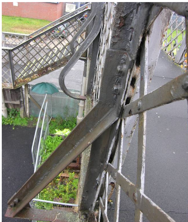
Photo 3 The central angled bracket on the eastern side, bolted onto the structure, looking south.
